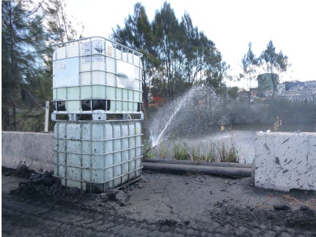
Photo 9 – Flocculant being sprayed into Dam M4
