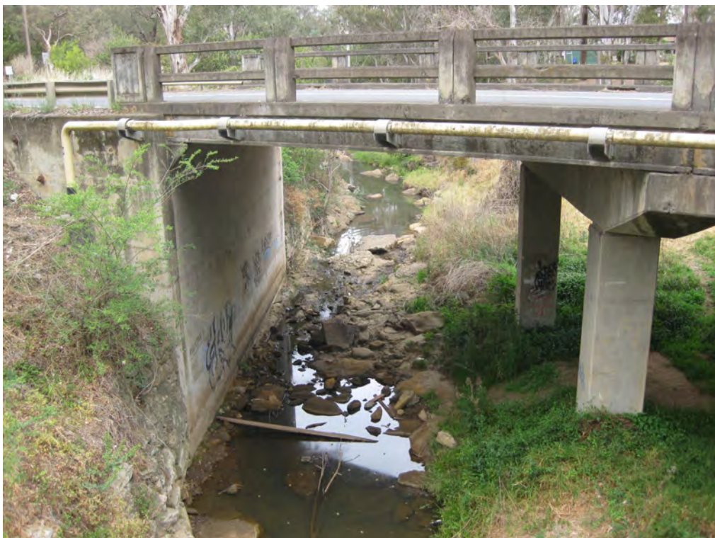
Photo 2 - Bridge Across Myrtle Creek on Remembrance Drive (not undermined)
