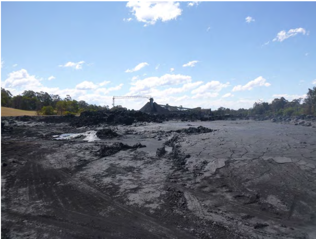
Photo 4 – ROM and product stockpile area
