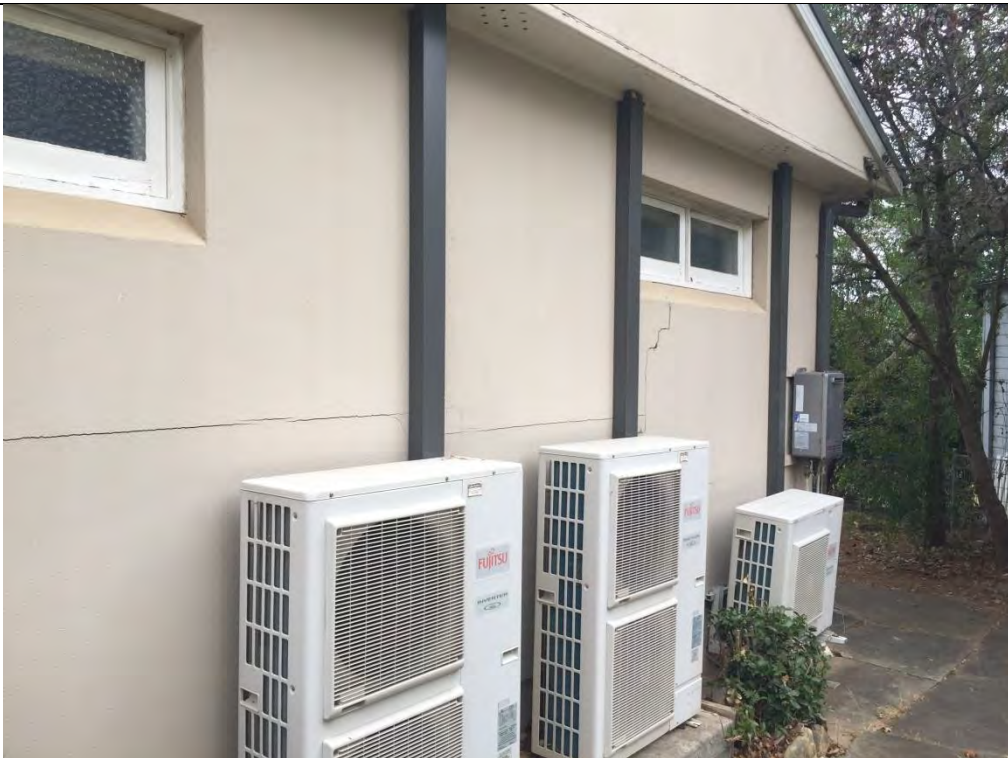
Photo 16 – Cracks in building caused by subsidence
