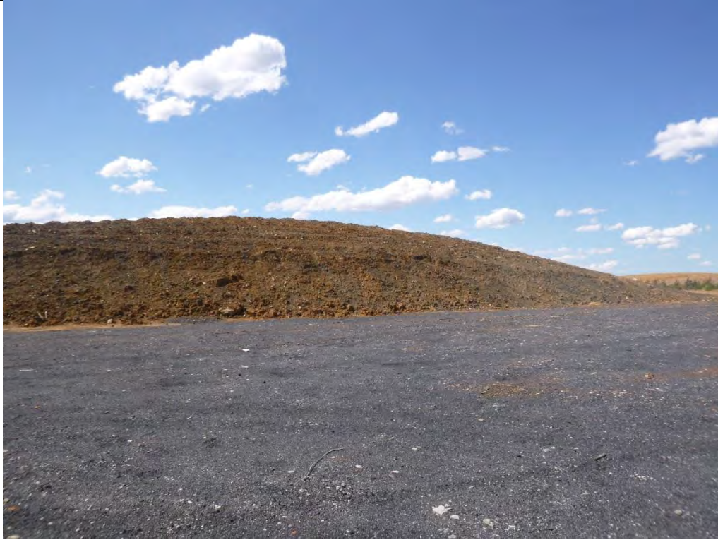
Photo 13 – Topsoil stockpile at REA over 3m in height
