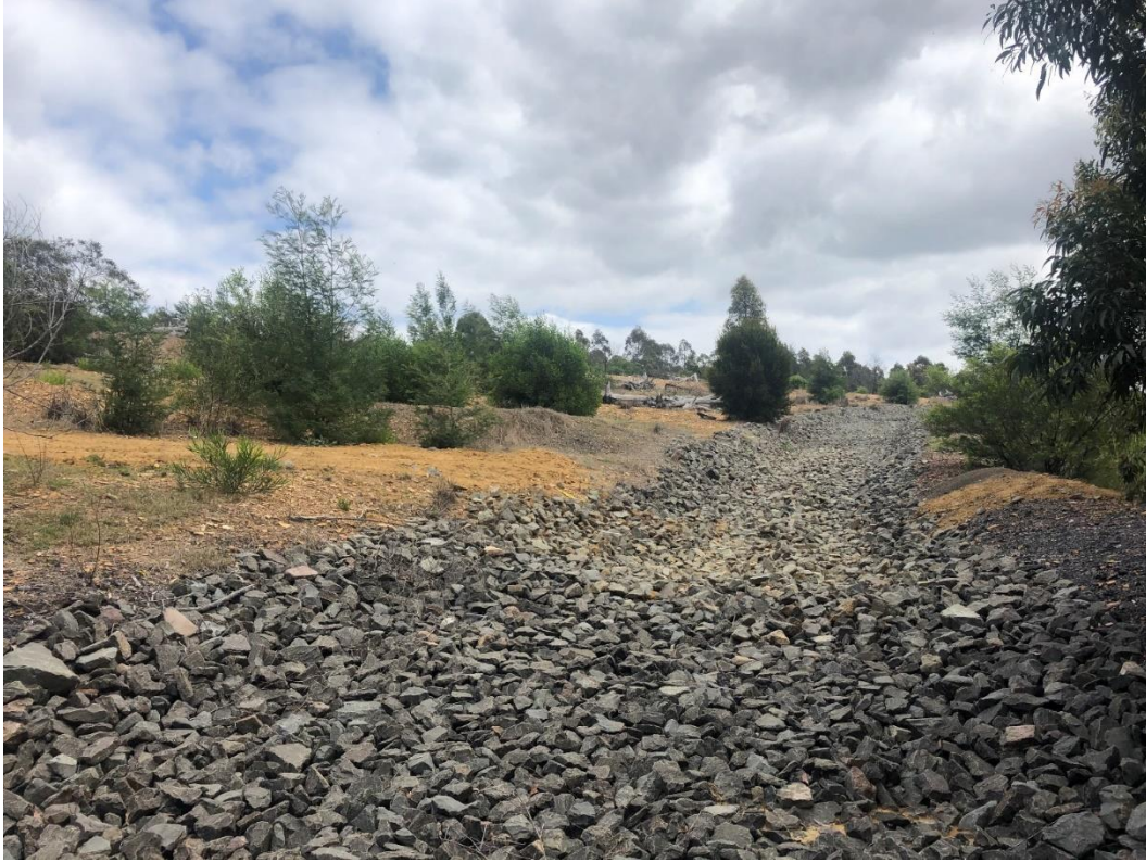
Photo 11 Successful implementation of rock armoured contour banks
