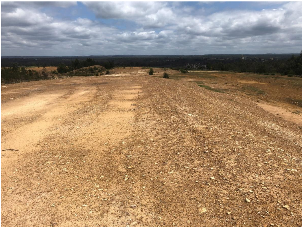
Photo 14 No cover vegetation on topsoil stockpile. Recommend seeding
