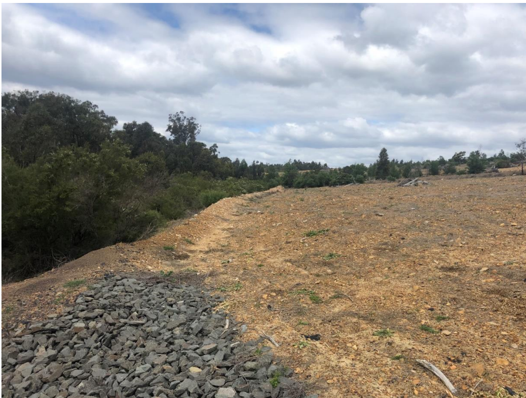
Photo 10 Successful implementation of rock armoured contour banks
