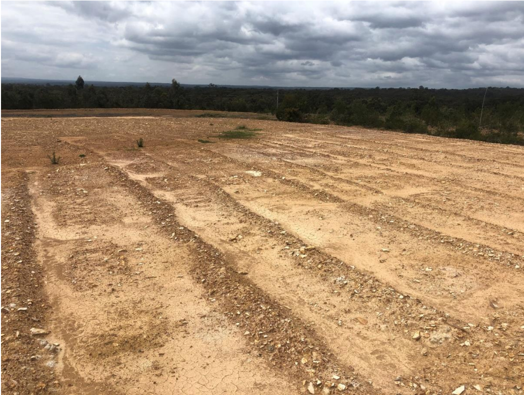
Photo 15 Photo 16 No cover vegetation on topsoil stockpile. Recommend seeding
