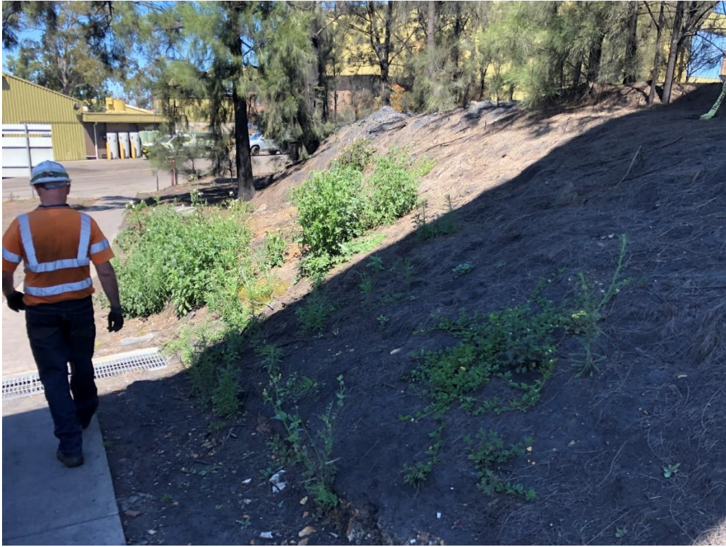
Photo 22 Evidence of weeds at the pit top
