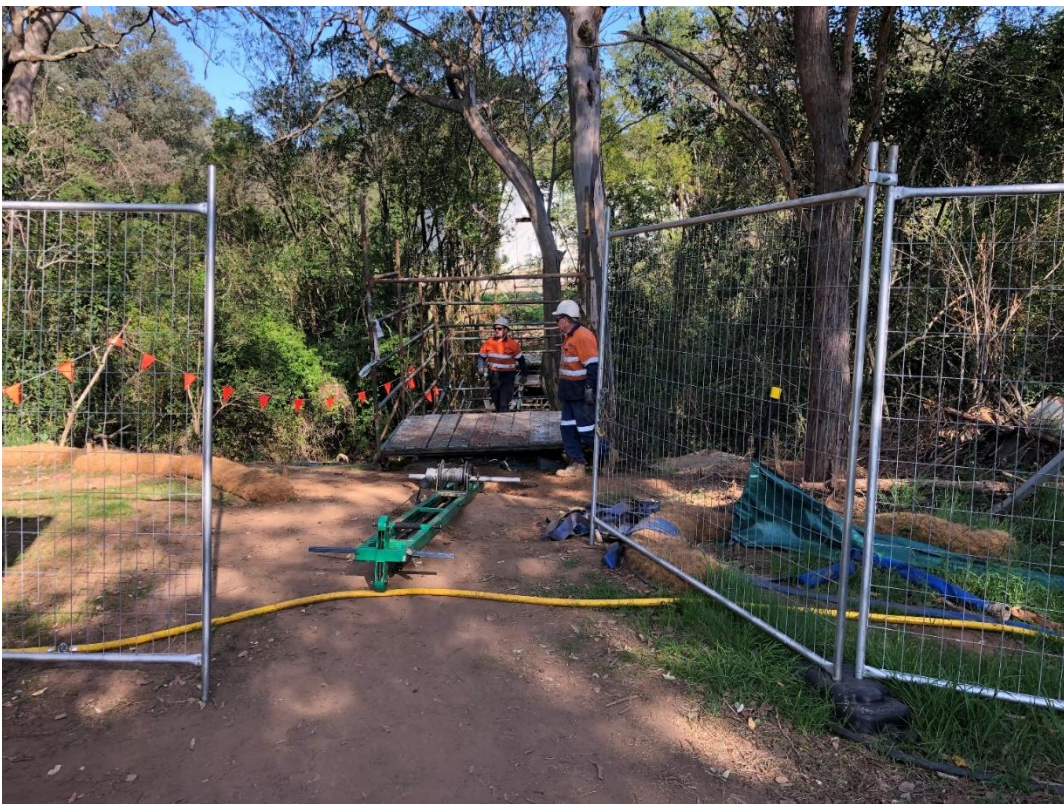
Photo 19 Creek CMAP works compound. Appropriate erosion and sediment controls in place
