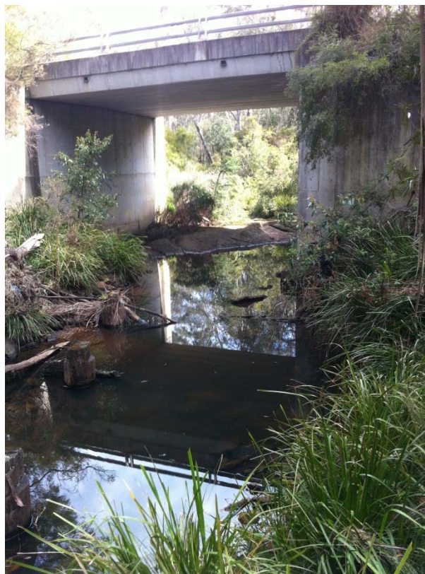
Fig. 5.7 Poned water in Dog Trap Creek near Bridge over Arina Road above previously extracted Longwall 13
