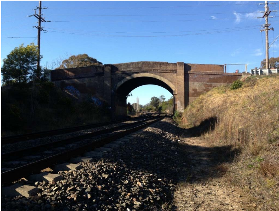
Fig. 6.4 Wellers Road Overbridge at 101.162 km
