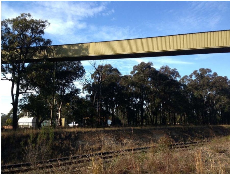
Fig. 6.3 Tahmoor Mine Overhead Coal Conveyor over the Main Southern Railway near 98.160 km
