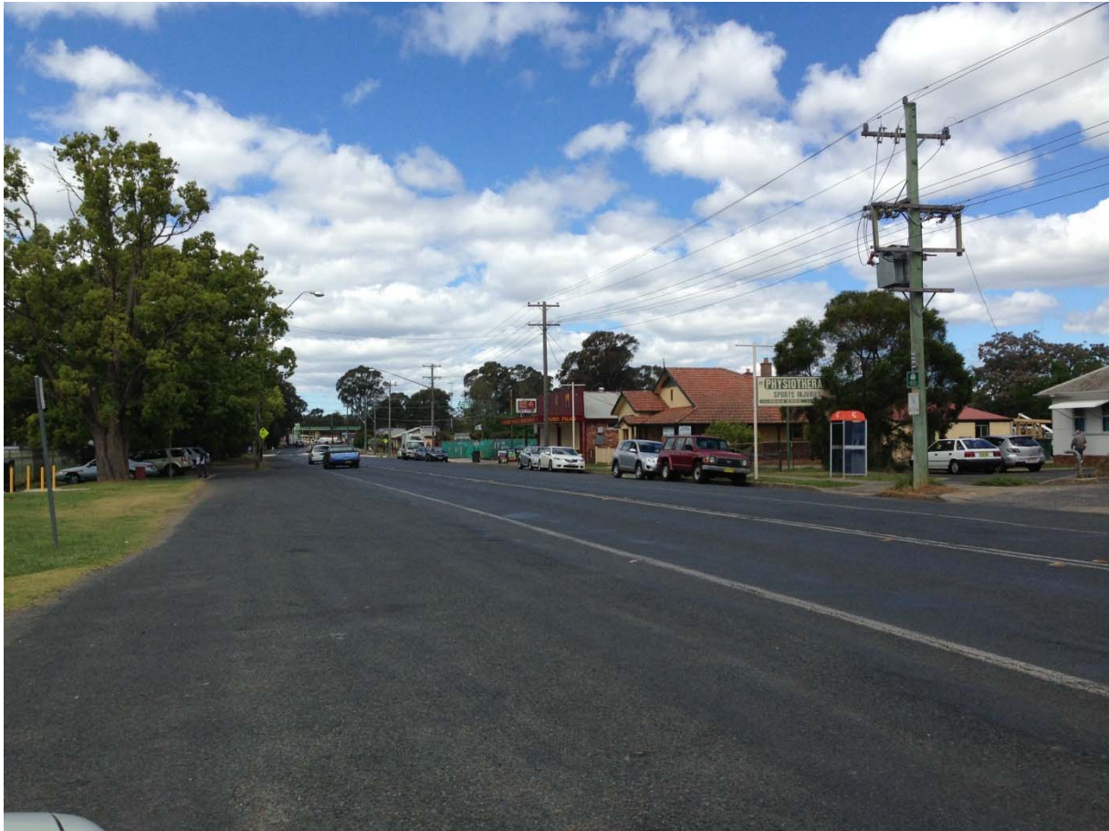
Fig. 6.16 Photograph of Remembrance Drive
