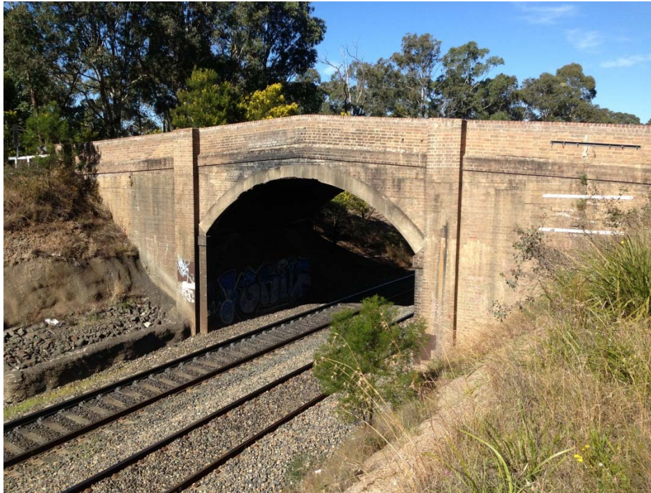
Fig. 6.6 Lupton Road Overbridge at 105.771 km
