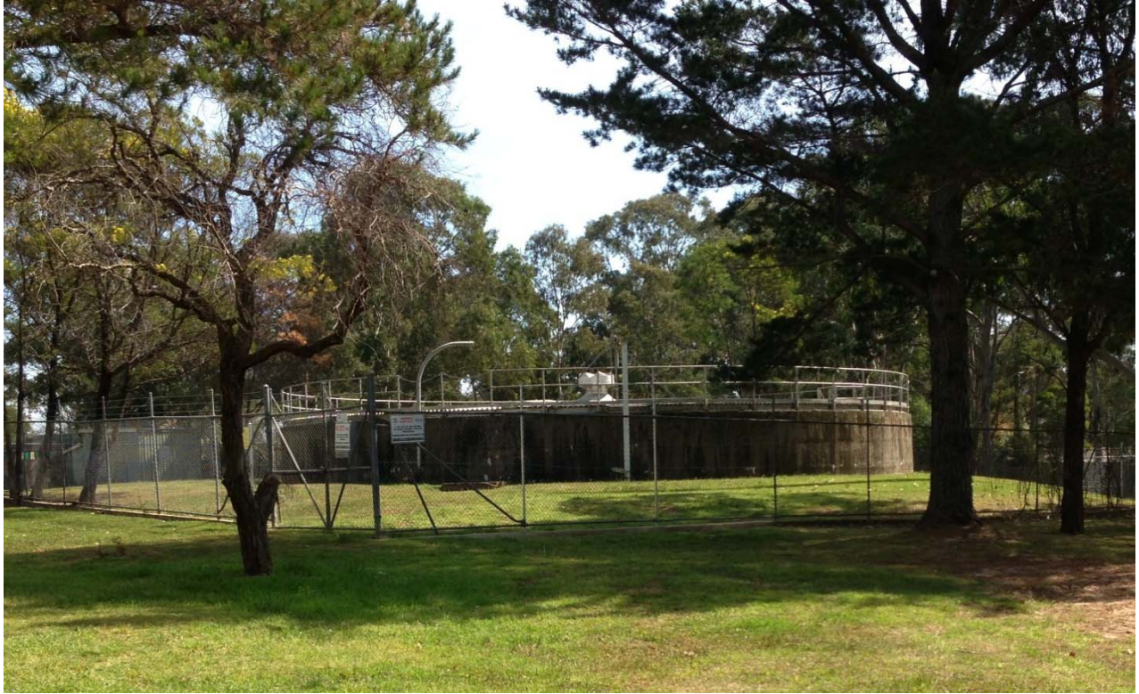
Fig. 6.19 Decommissioned Sydney Water Reservoir at Radnor Road, Bargo
