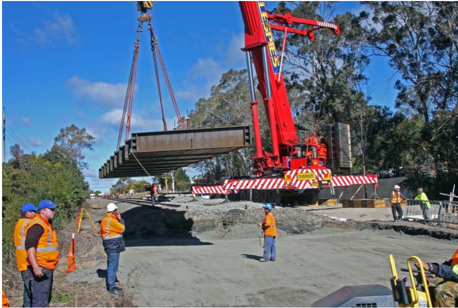
Photographs courtesy Pidgeon Civil Engineering
