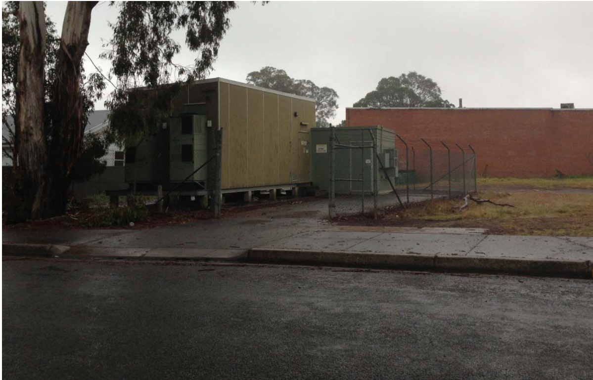
Fig. 6.24 Telstra Exchange at Bargo
