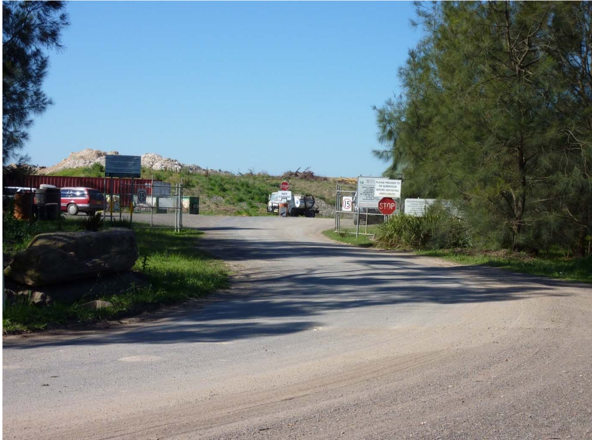
Fig. 9.1 Bargo Waste Management Centre
