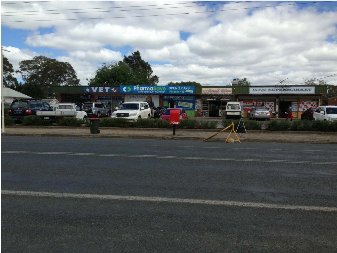
Fig. 7.2 Shops on Remembrance Drive at Bargo
