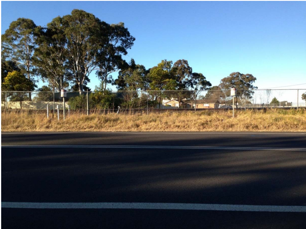
Fig. 6.20 Warning markers showing position of buried gas and ethane pipelines beneath Remembrance Drive and Main Southern Railway
