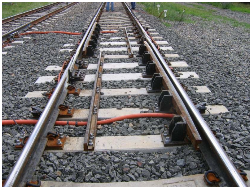
Fig. 6.2 Rail Expansion Switch
