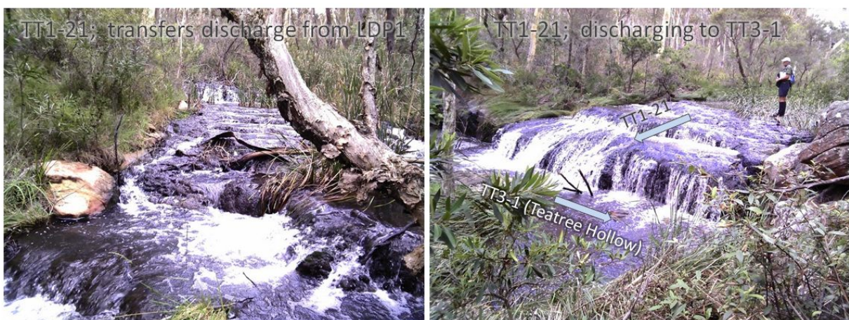
Figure 43. TT1-21 in the vicinity of where it transfers discharge from LDP1 to Teatree Hollow. Exposed bedrock and boulders in the bed were covered by a layer of dark-coloured precipitate. Photographed on 6 February 2013.
