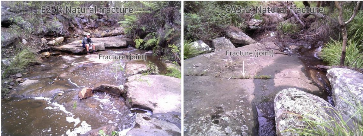
Figure 24. Examples of natural fractures in exposed bedrock. Photographed on 11 February 2013 for E2-1, and 30 January 2013 for CA3-1.
