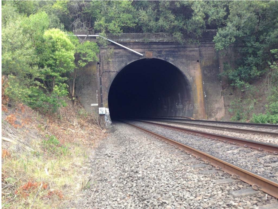
Fig. 6.8 Picton Rail Tunnel
