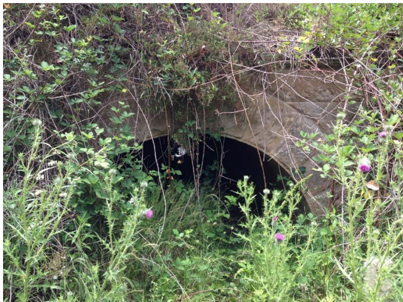
Fig. 6.4 Loop line culvert at 88.400 km
