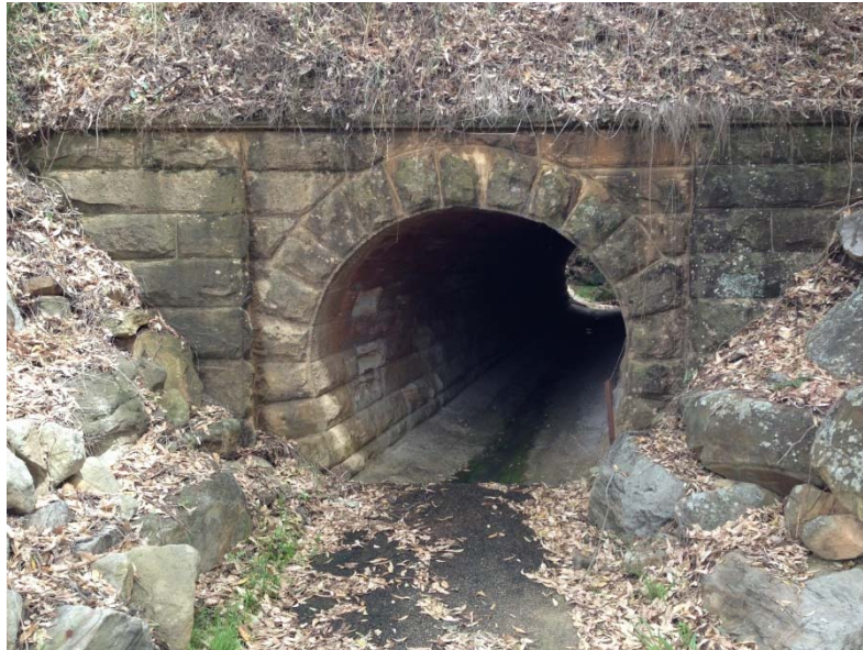
Fig. 6.5 Loop line culvert at 88.980 km
