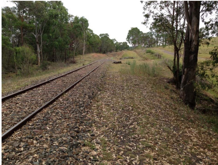
Fig. 6.1 Picton to Mittagong Loop Line at 88.980 km (looking north)
