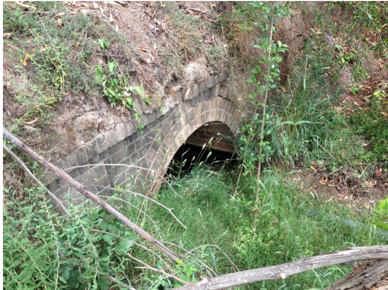
Fig. 6.3 Loop line culvert at 87.850 km
