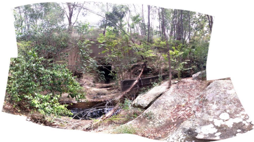
Fig. 5.19 Rumker Gully upstream of Picton to Mittagong Loop Line
