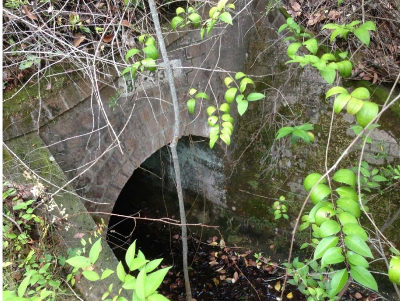
Fig. 6.2 Loop line culvert at 87.330 km
