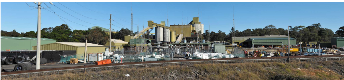
Plate 10 – Existing surface facilities and coal handling preparation plant
