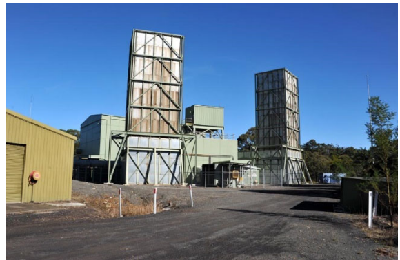
Plate 4 - View toward existing T2 up-cast shaft
