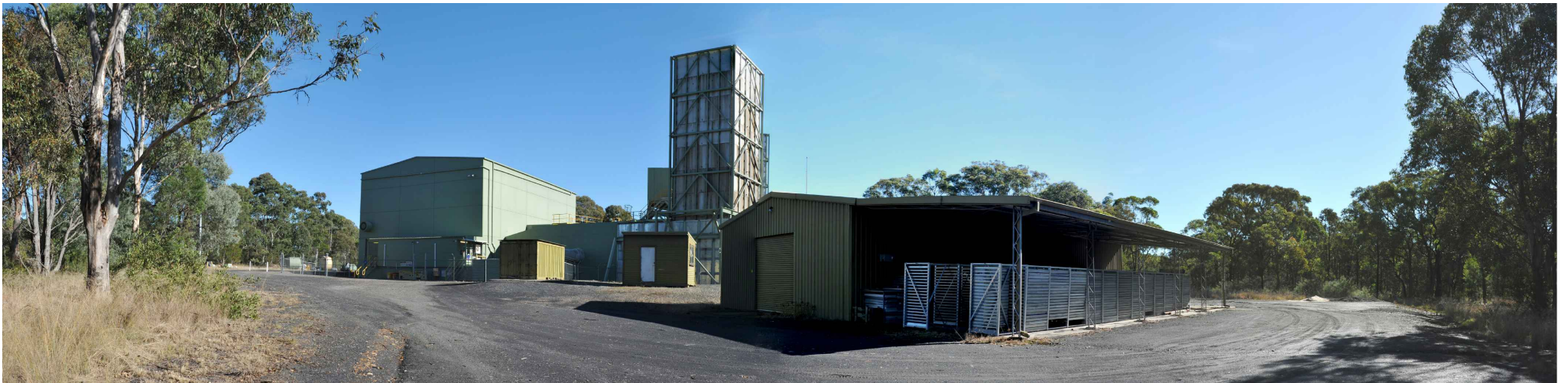
Existing T2 up-cast ventilation shaft (off Rockford Road) - East elevation
