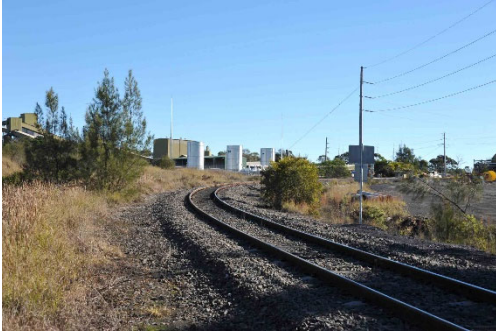
Plate 9 – Rail loop entering surface facilities area
