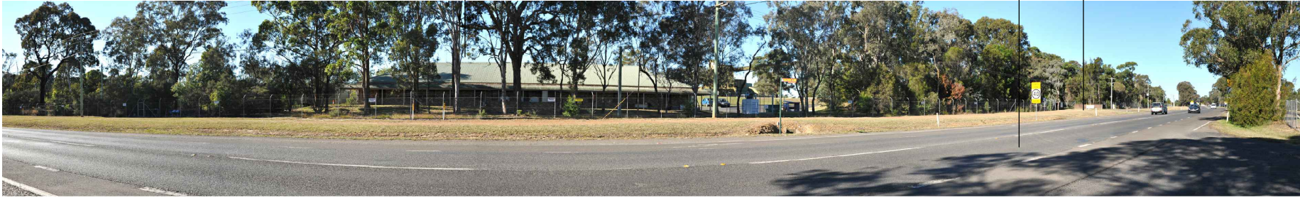
Photo Location P4 - View north east to south east from Olive Lane intersection with Remembrance Drive
