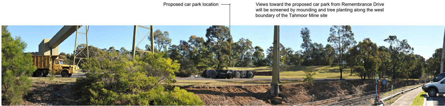
Photo Location P17 - View west across Tahmoor Coal mine rail loop toward proposed car park location
