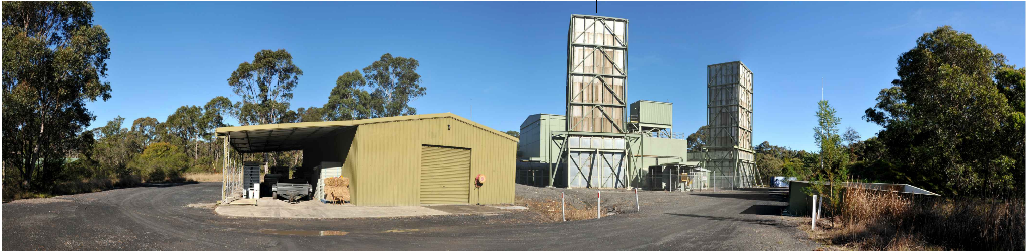
Existing T2 up-cast ventilation shaft (off Rockford Road) - South elevation
