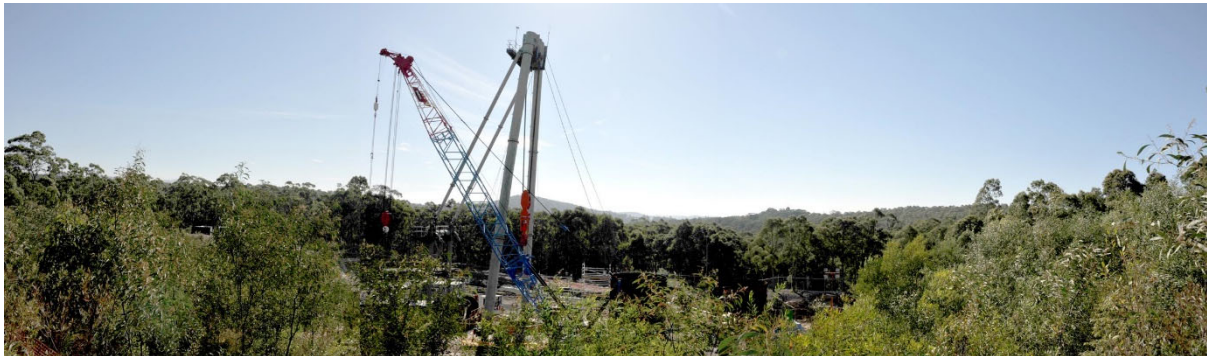
Plate 6 – Typical view toward an up-cast vent shaft installation site
