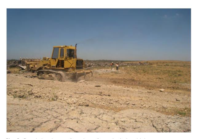
Plate 5 – Deep ripping prior to seeding and spreading previously cleared timber
