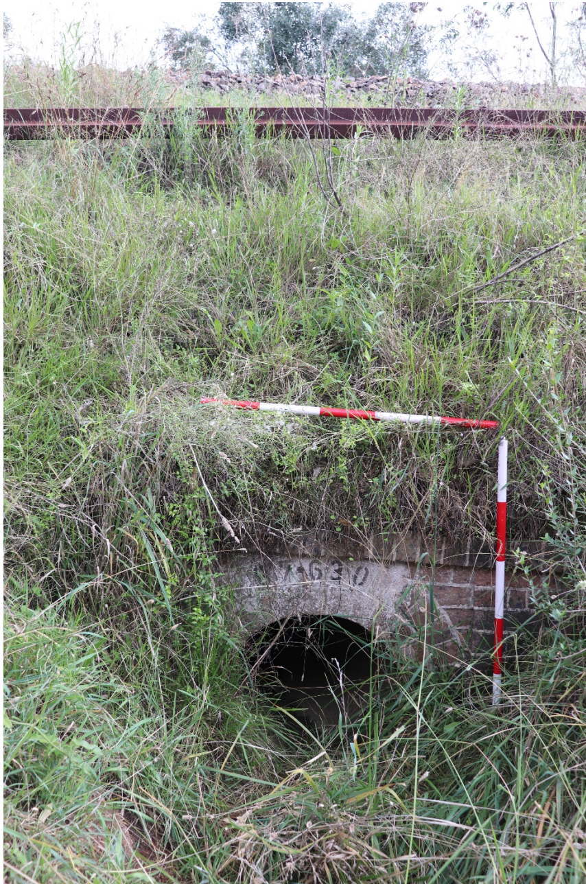
Plate 3.2 Brick culvert (chainage 87.630). View north west.
