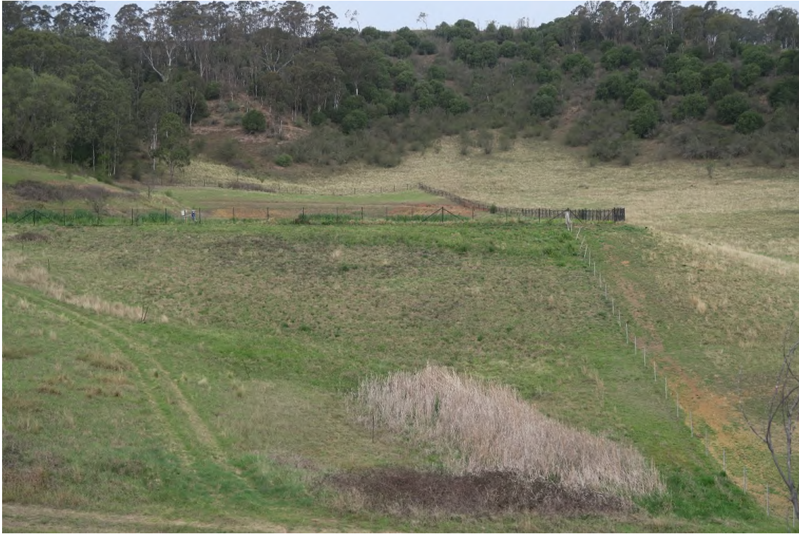
Figure 3-1 View of Stonequarry Wastewater Treatment Dam from Embankment at 87.850 km
