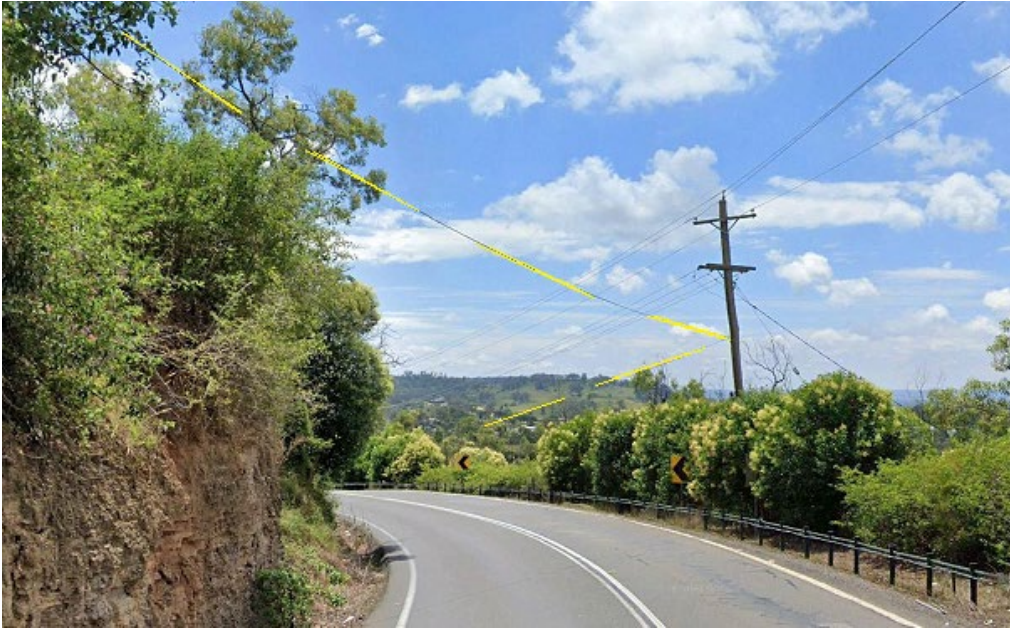
Plate 5: View of NBNC Co Local aerial cable along Thirlmere Way crossing the road to property north side of Thirlmere Way on the southern edge of the Study Area
