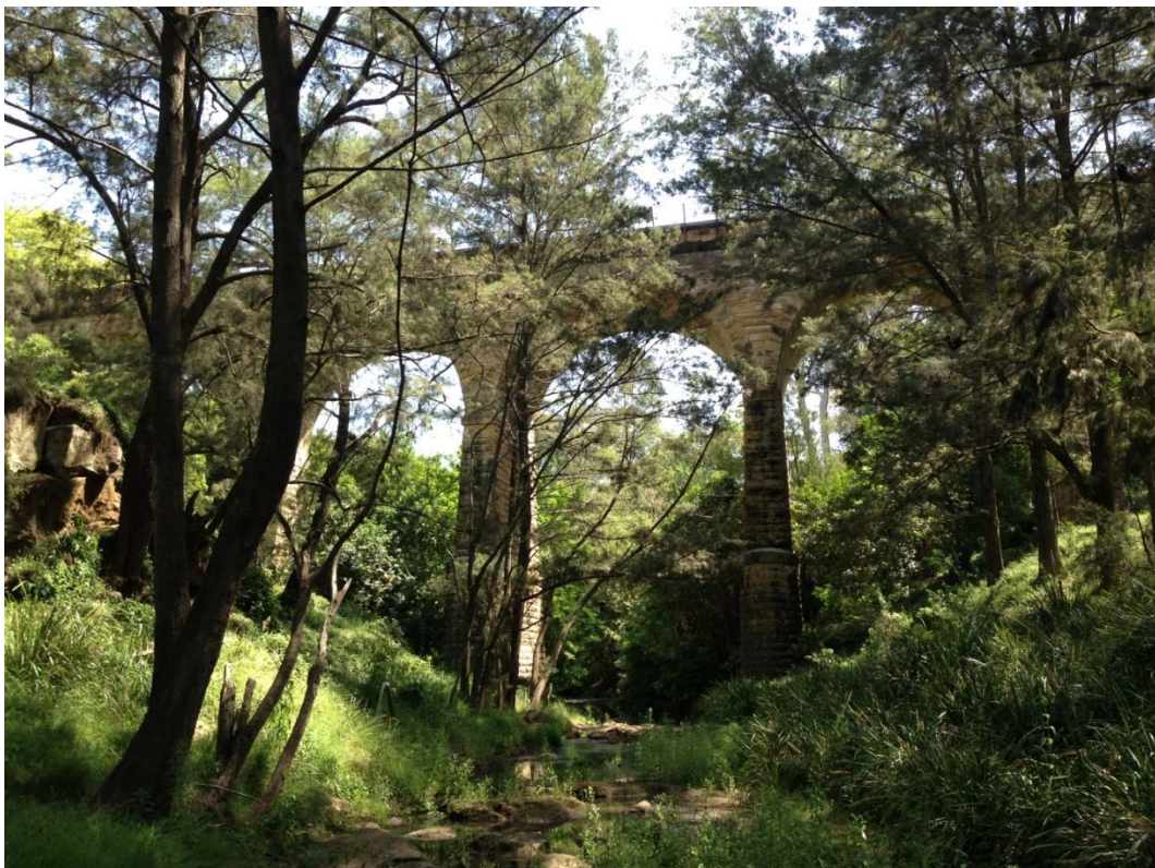
Fig. 2.31 Picton Viaduct at 85.42 km over Stonequarry Creek
