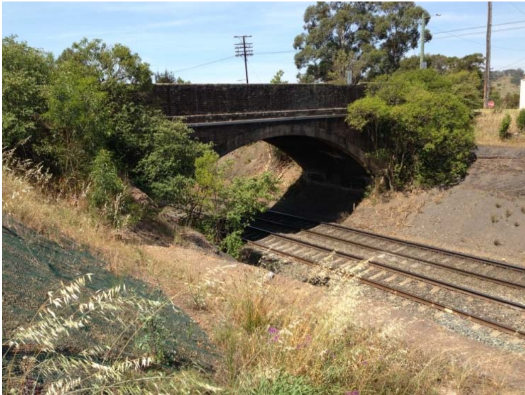
Fig. 2.21 Connellan Crescent Railway Overbridge at 89.080 km
