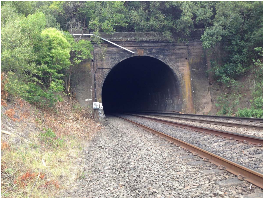
Fig. 2.24 Picton Railway Tunnel – Southern Portal
