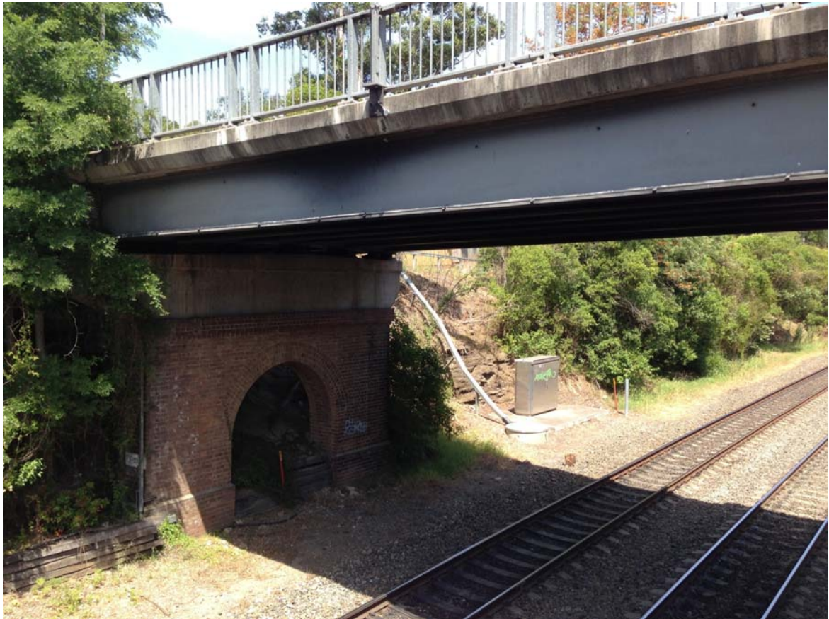
Fig. 2.36 Prince Street Overbridge at 85.17 km
