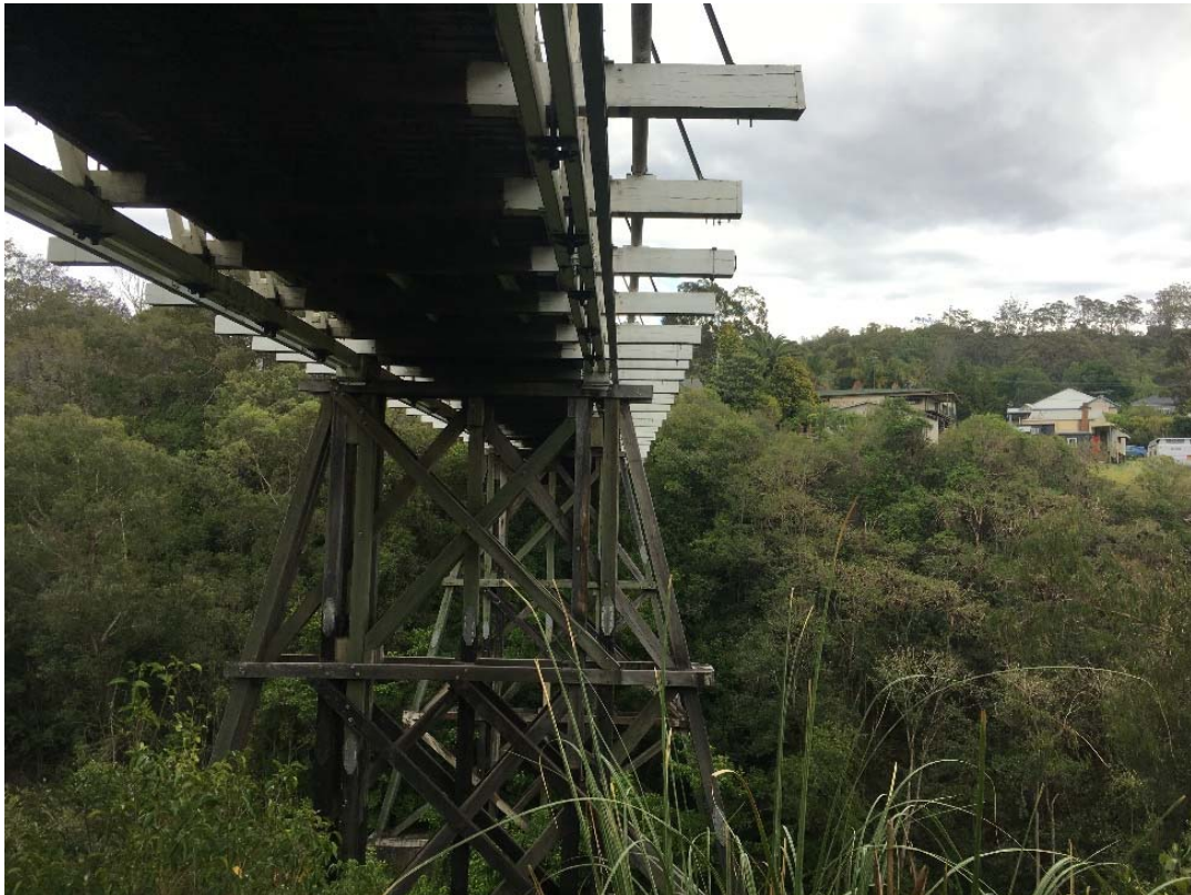
Fig. 2.41 Victoria Bridge timber trestles
