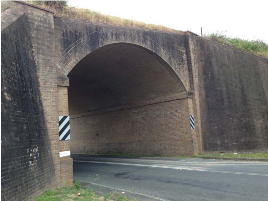
Fig. 2.18 Thirlmere Way Rail Underbridge at 89.326 km
