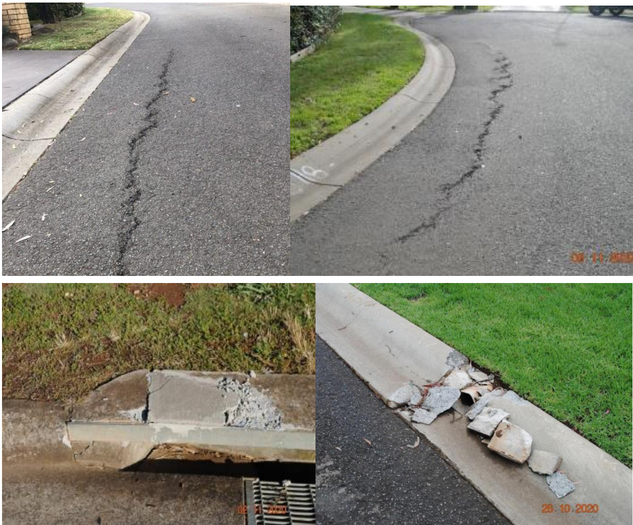
Fig. 3.11 Impacts on local roads and kerbs during LW W1
