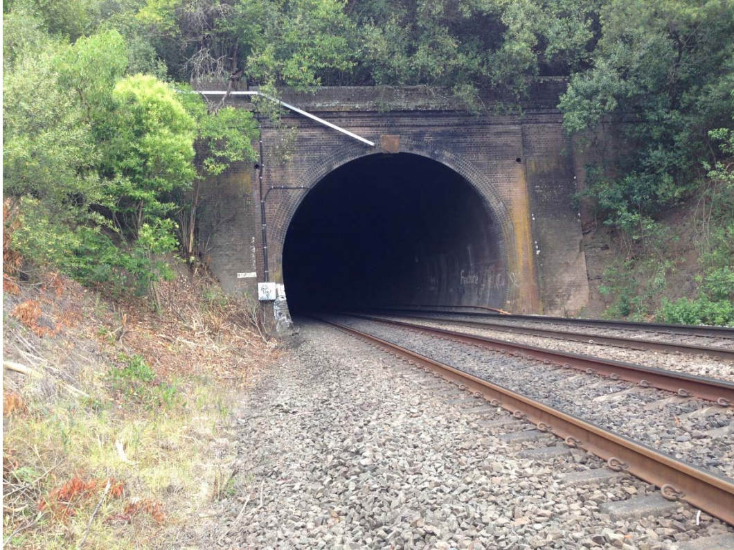
Fig. 2.25 Picton Railway Tunnel – Southern Portal
