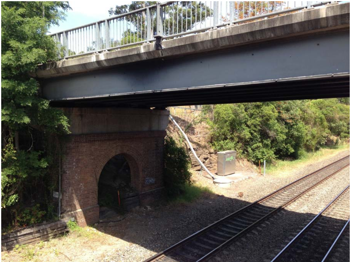
Fig. 2.33 Prince Street Overbridge at 85.17 km
