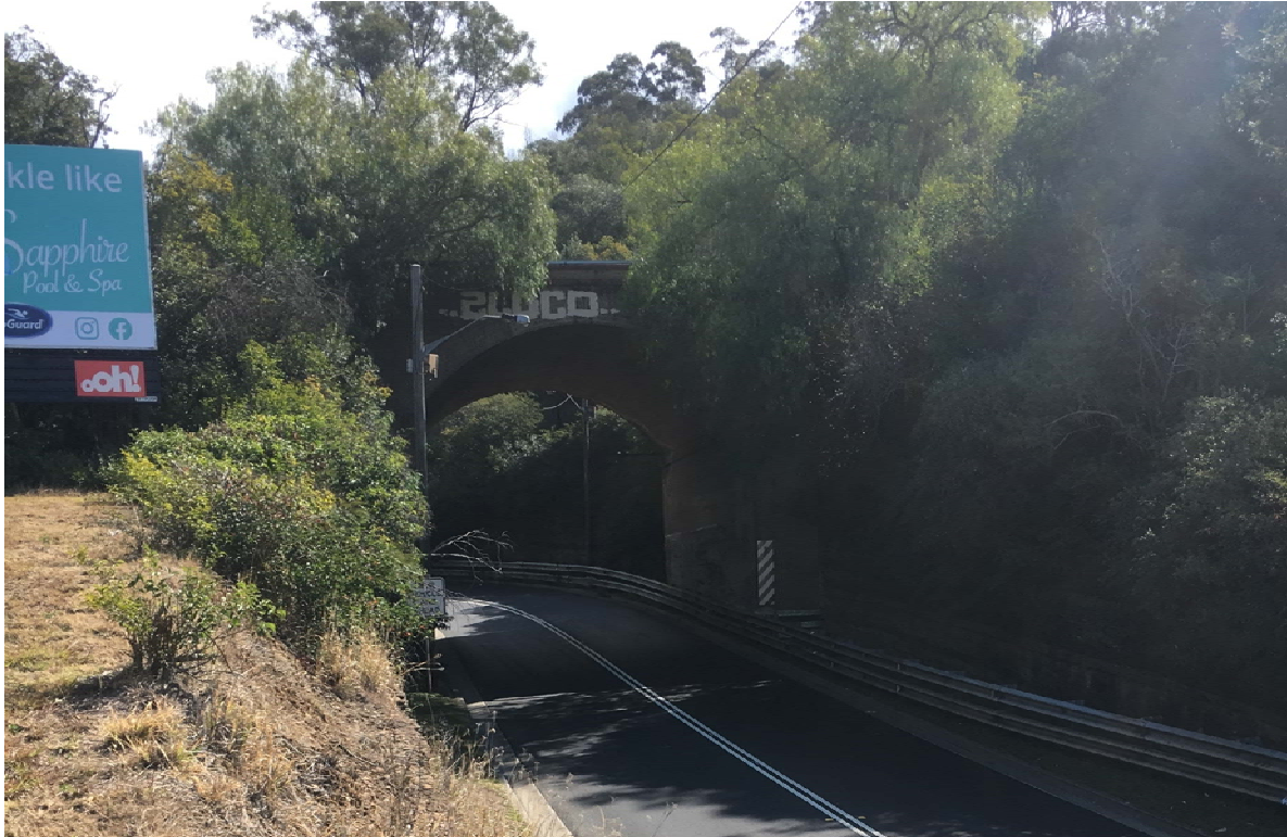
Fig. 2.27 Argyle Street Rail Underbridge at 86.160 km
