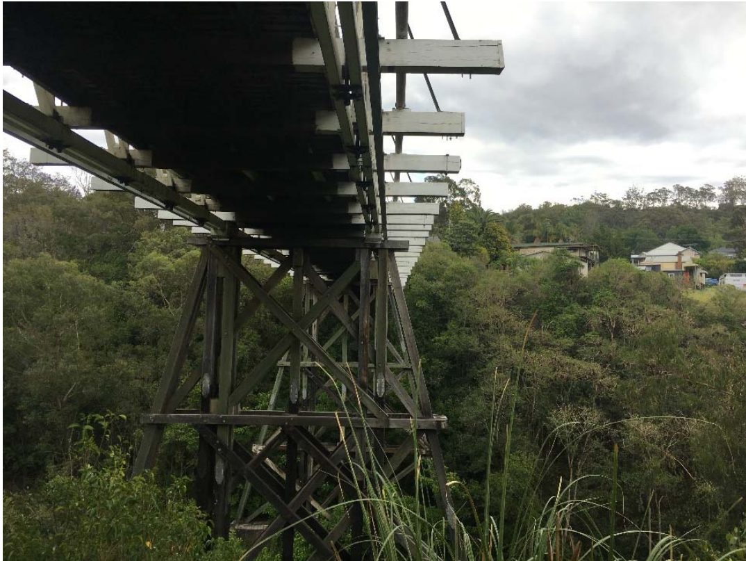
Fig. 2.37 Victoria Bridge timber trestles
