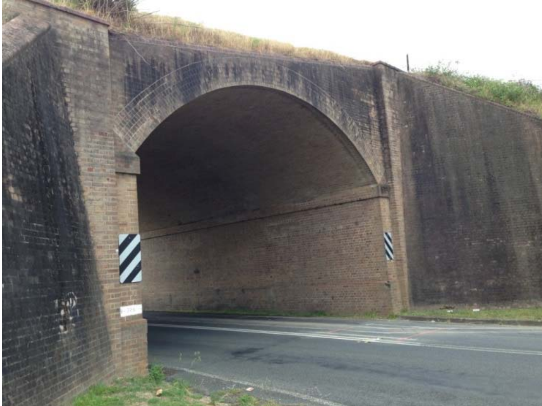
Fig. 2.21 Thirlmere Way Rail Underbridge at 89.326 km
