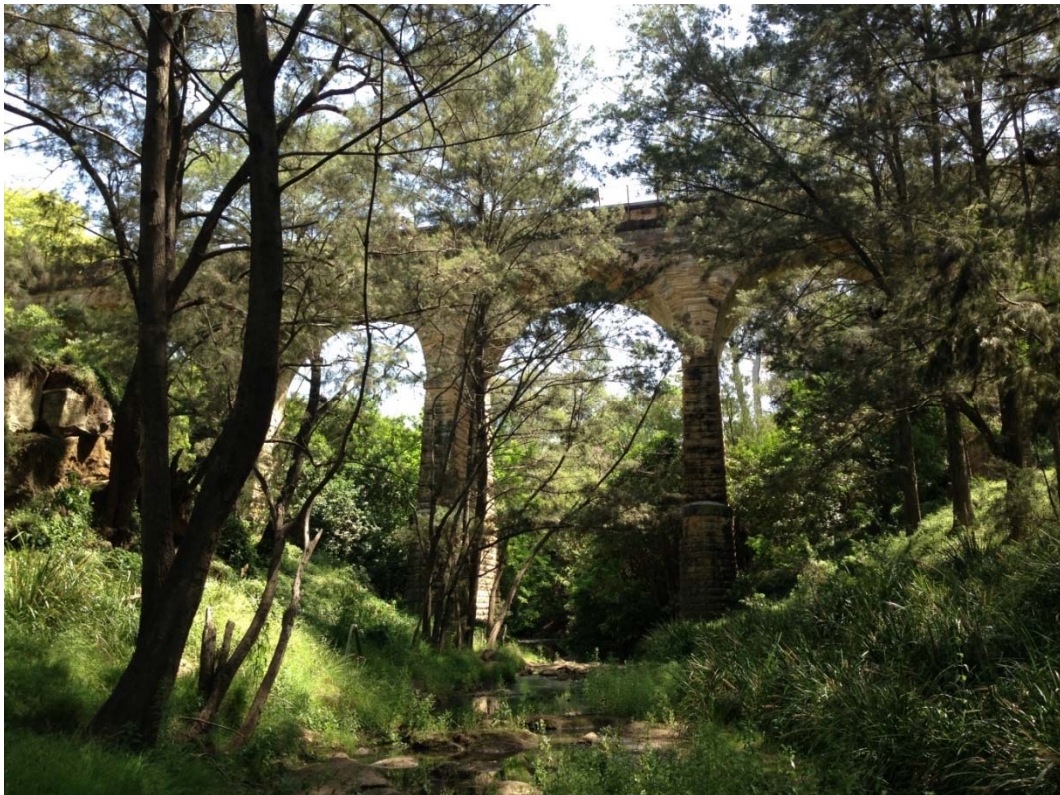
Fig. 2.29 Picton Viaduct at 85.42 km over Stonequarry Creek
