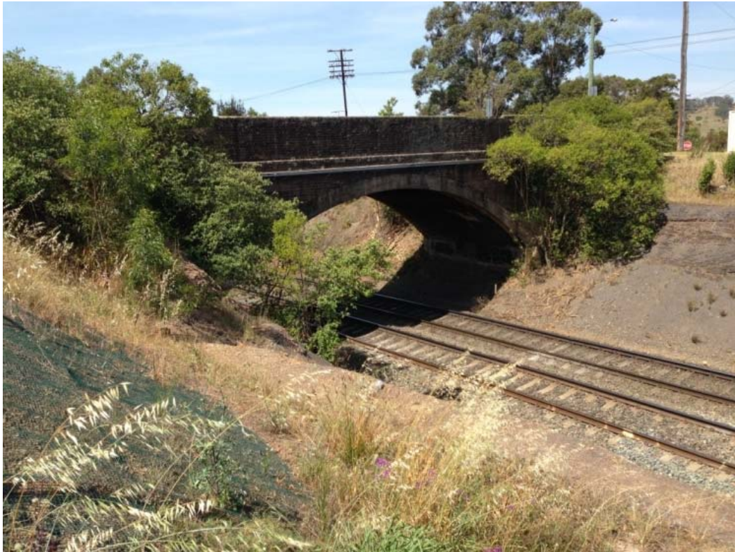
Fig. 2.23 Connellan Crescent Railway Overbridge at 89.080 km
