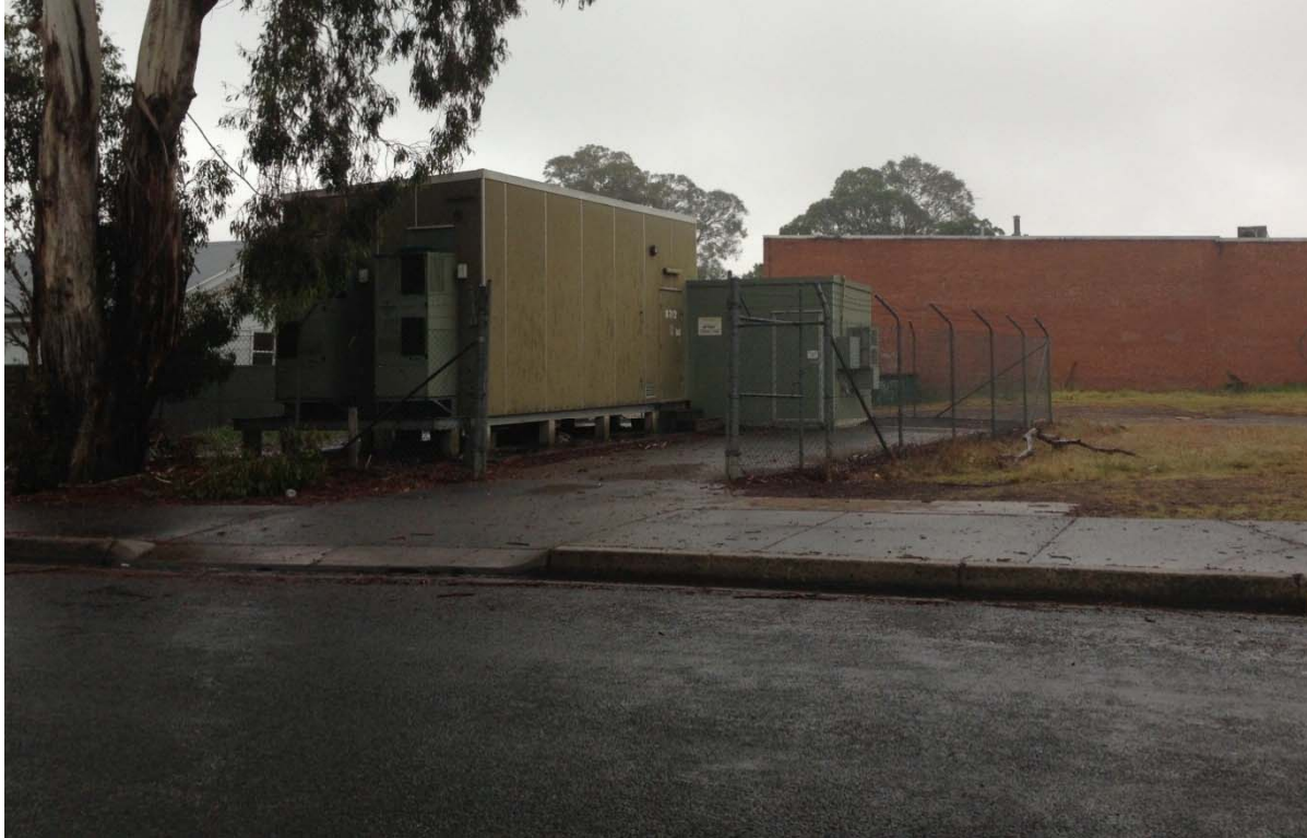
Fig. 6.24 Telstra Exchange at Bargo
