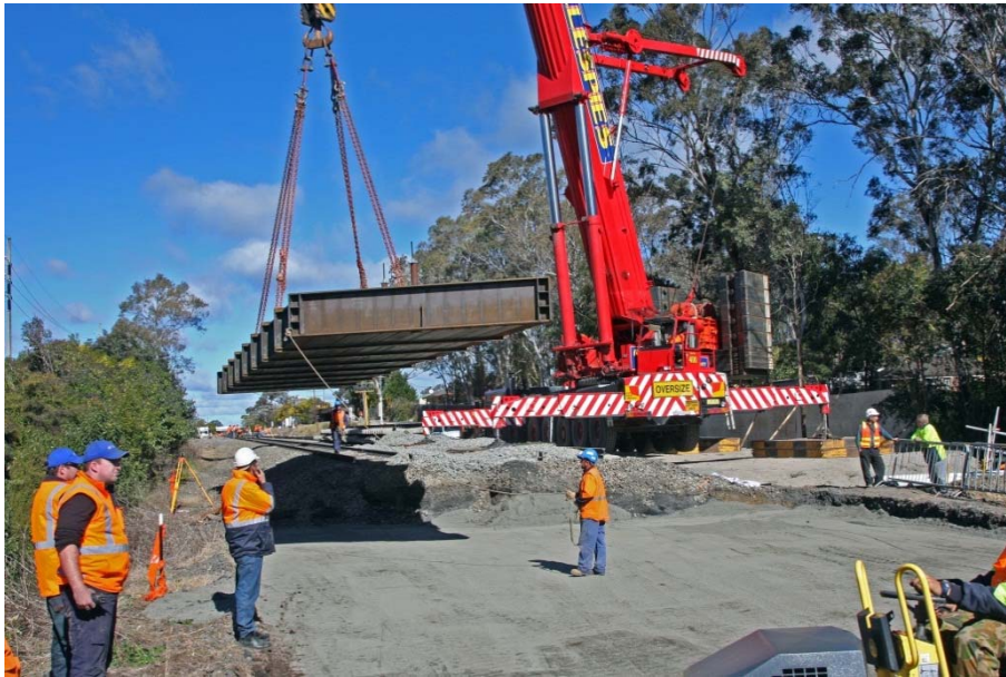
Photographs courtesy Pidgeon Civil Engineering
