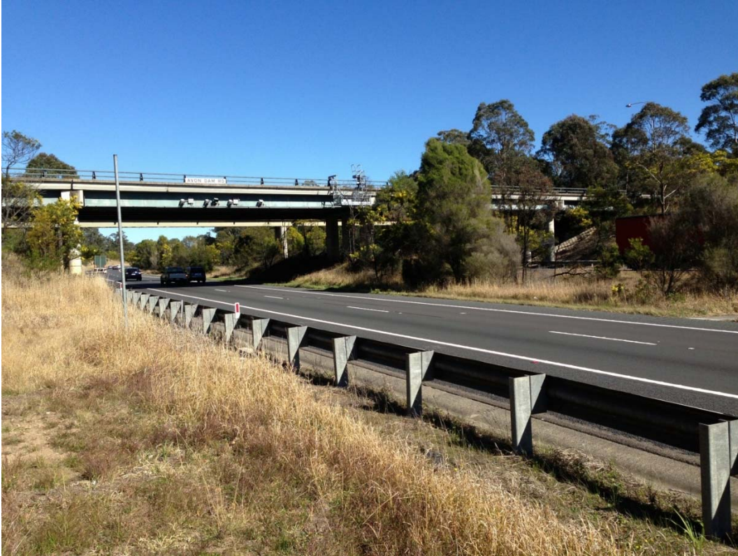
Fig. 6.12 Avon Dam Road Bridge over M31 Hume Motorway
