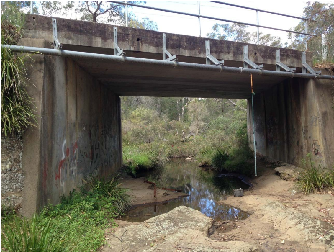
Fig. 6.17 Bargo Road Bridge over Dog Trap Creek
