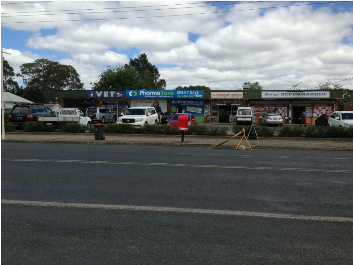
Fig. 7.2 Shops on Remembrance Drive at Bargo
