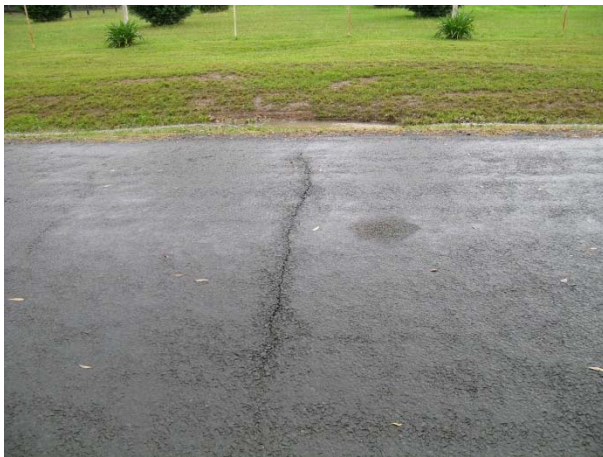
Fig. 6.18 Previously observed impacts on local roads above Tahmoor Mine
