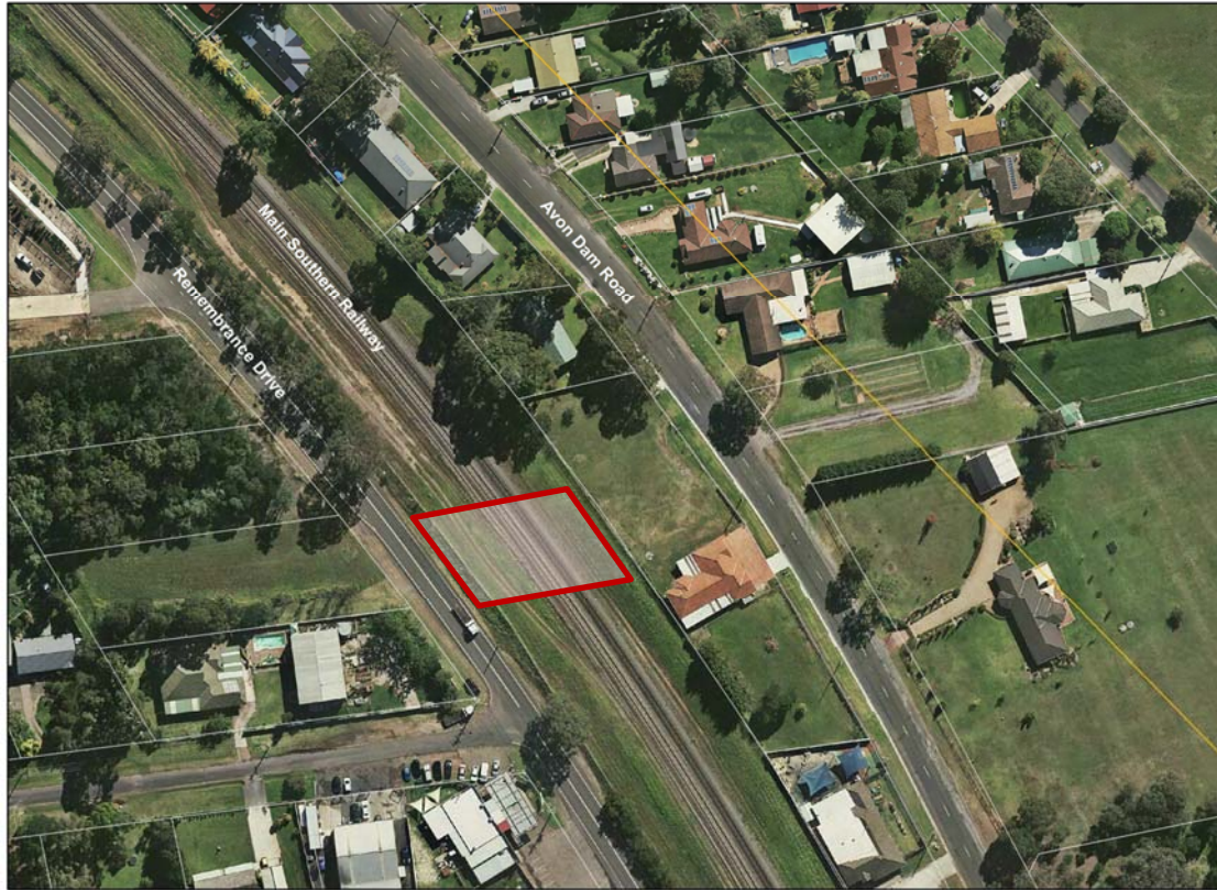
Fig. 6.21 Aerial photo, marked to show the position of buried gas and ethane pipelines beneath Remembrance Drive and Main Southern Railway
