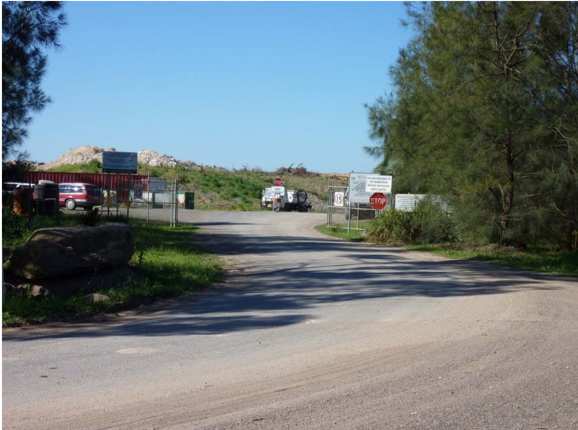
Fig. 9.1 Bargo Waste Management Centre
