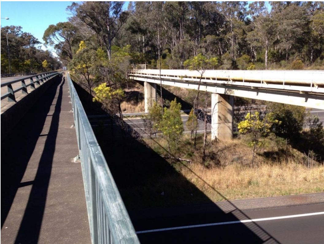
Fig. 6.13 Water pipe bridge over M31 Hume Motorway adjacent to Avon Dam Road
