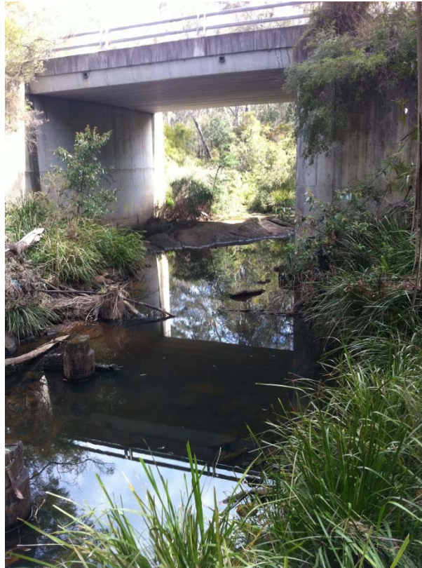
Fig. 5.7 Ponded water in Dog Trap Creek near bridge over Arina Road above previously extracted Longwall 13
