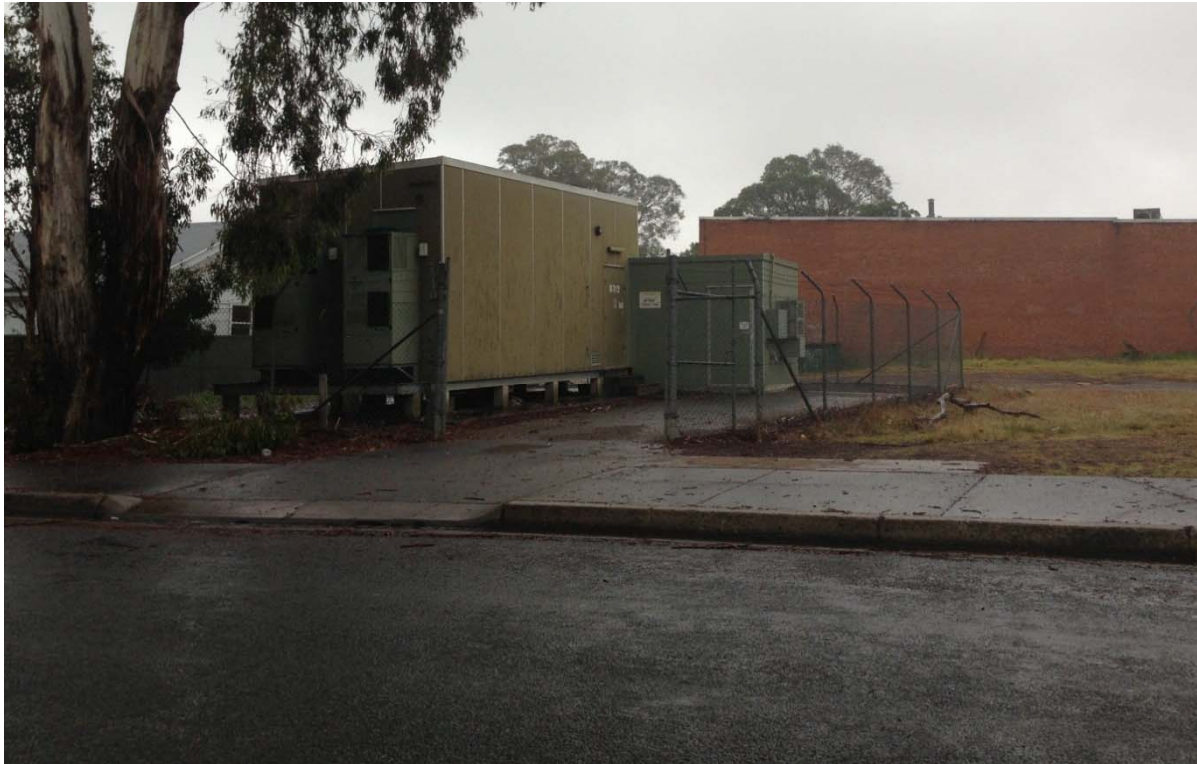
Fig. 6.23 Telstra Exchange at Bargo
