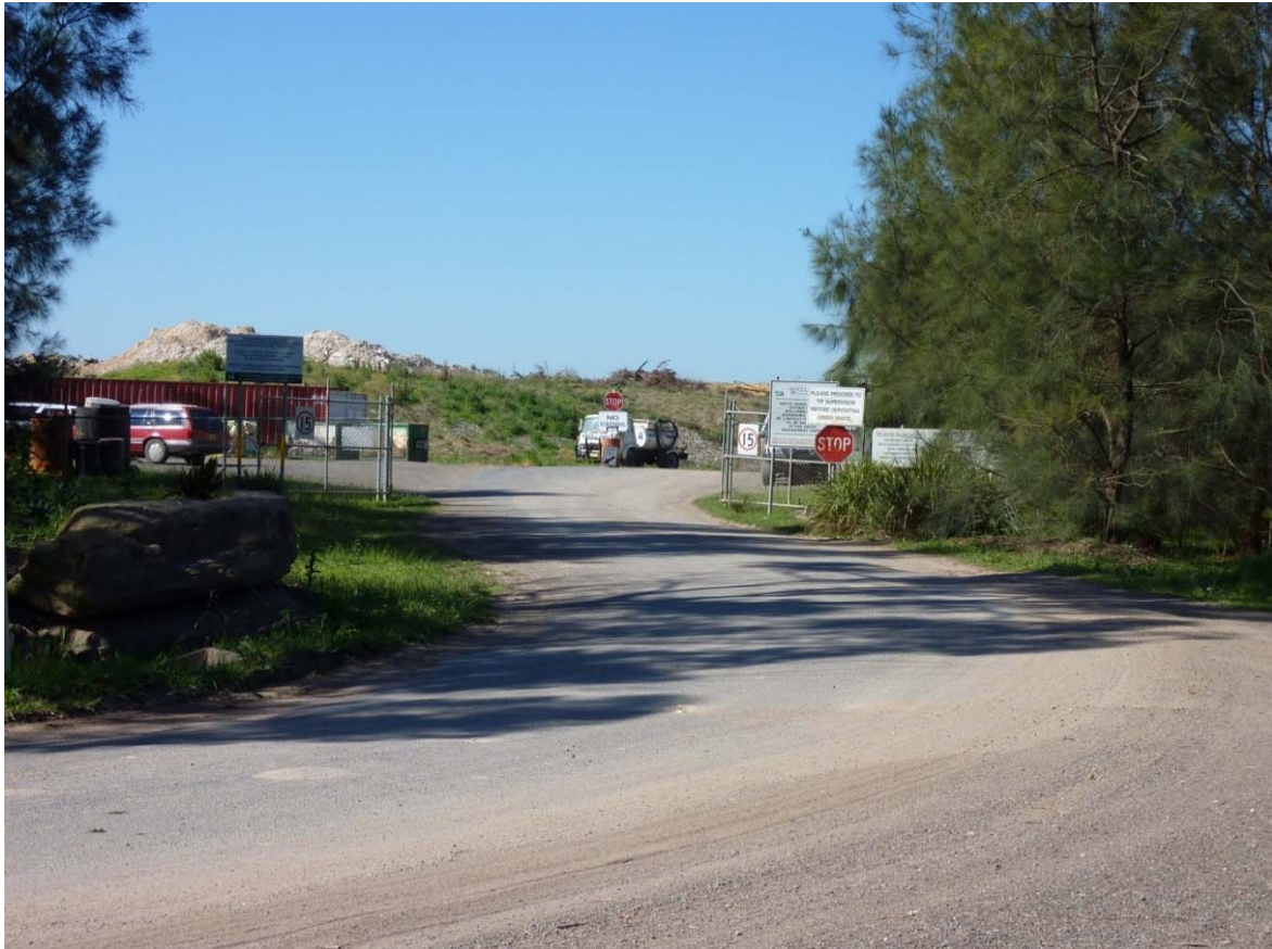
Fig. 9.1 Bargo Waste Management Centre
