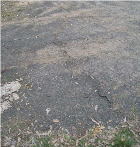
Fig. 4.9 Surface compression buckling observed in a pavement
