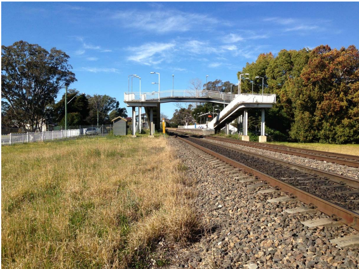
Fig. 6.1 Main Southern Railway at Bargo Station and pedestrian overbridge at 102.873 km
