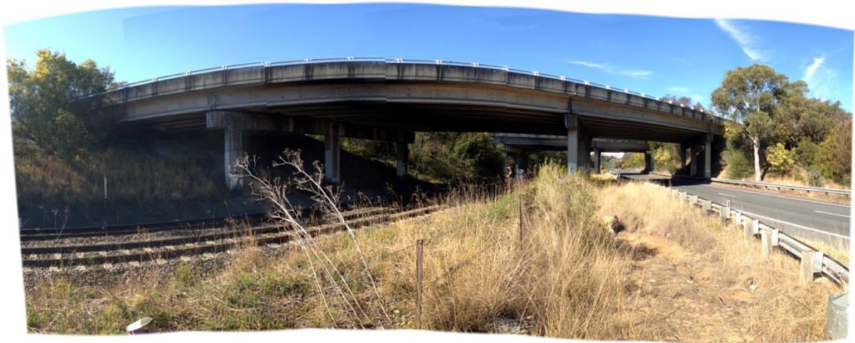
Fig. 6.14 M31 Hume Motorway Overbridge at 107.507 km
