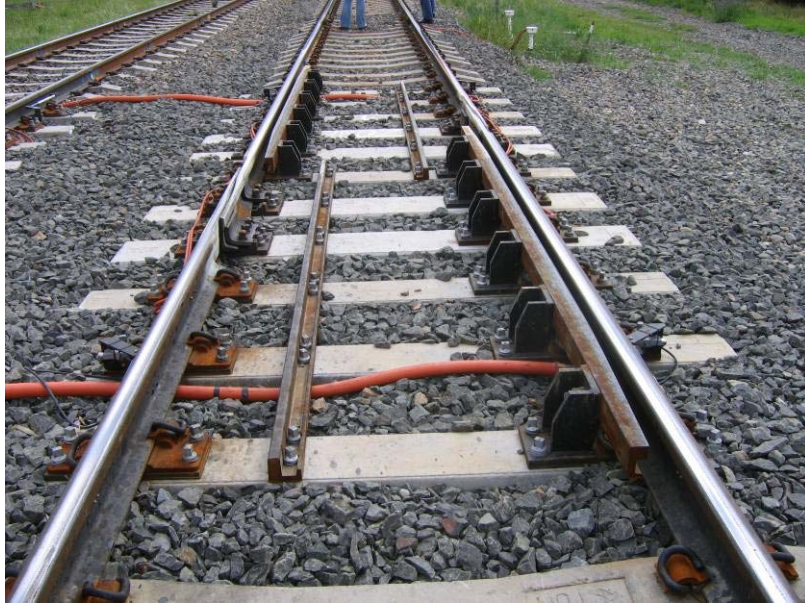
Fig. 6.2 Rail expansion switch
