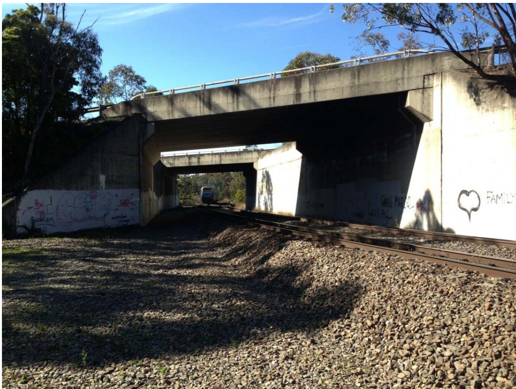
Fig. 6.15 M31 Hume Motorway Overbridge at 108.784 km
