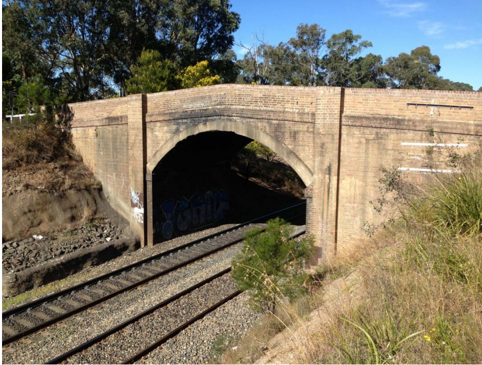
Fig. 6.6 Lupton Road Overbridge at 105.771 km
