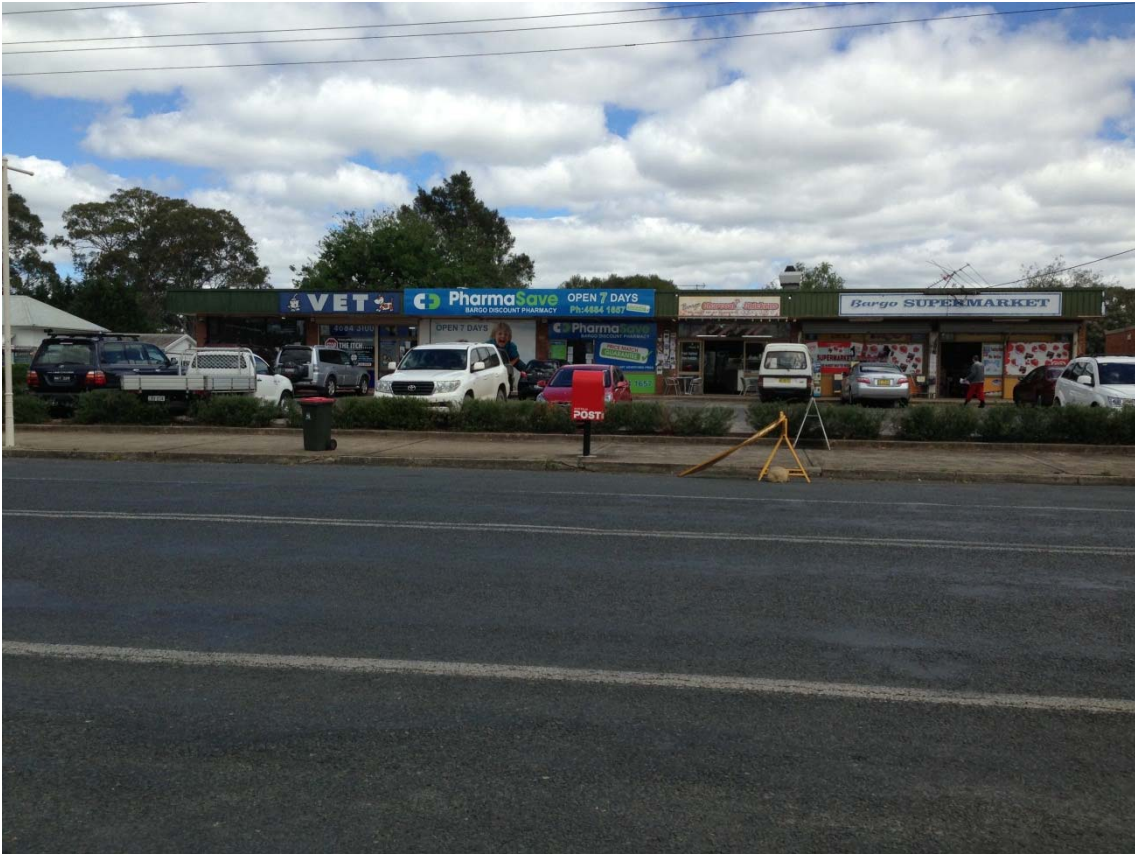
Fig. 7.2 Shops on Remembrance Drive at Bargo
