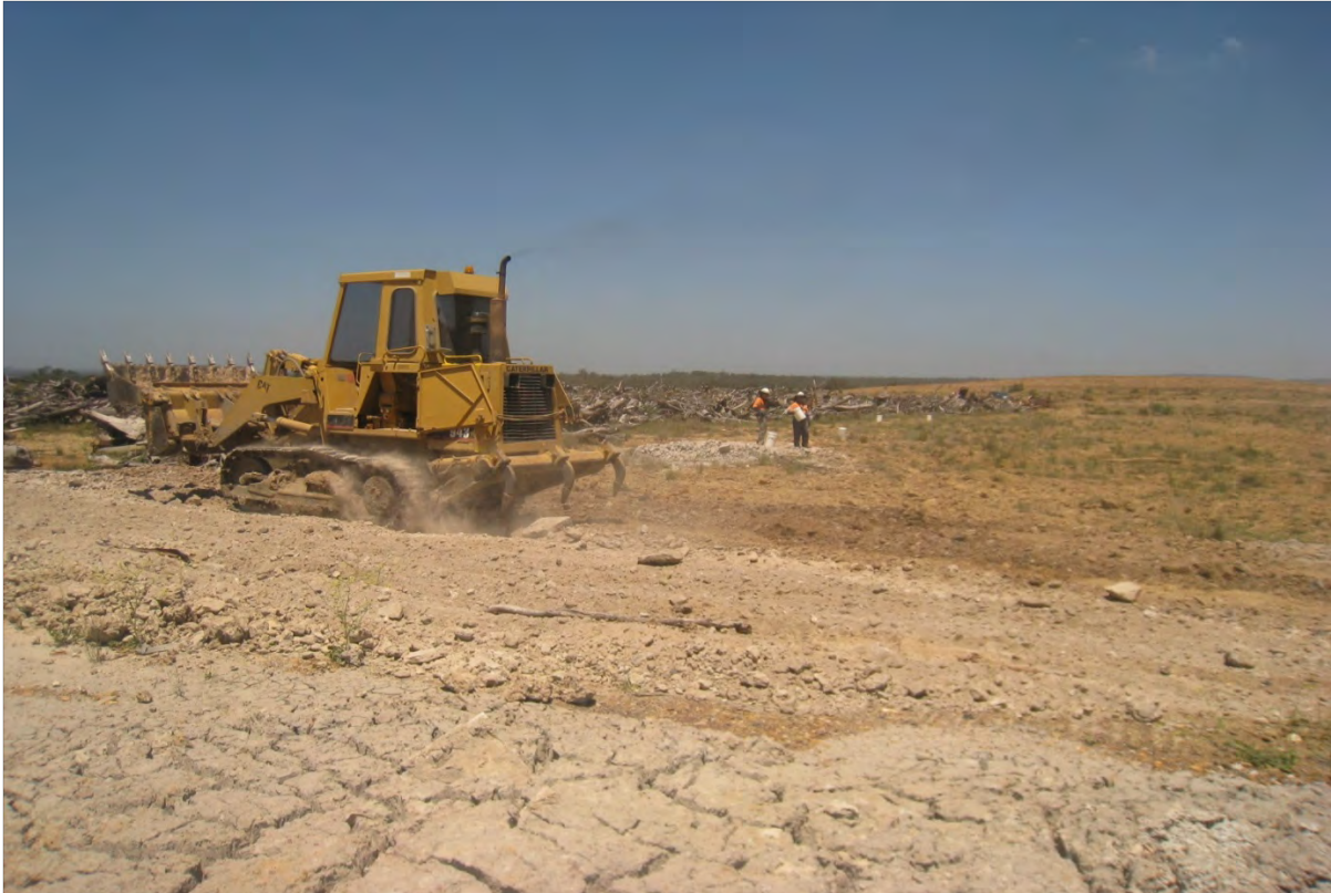
Plate 5 – Deep ripping prior to seeding and spreading previously cleared timber
