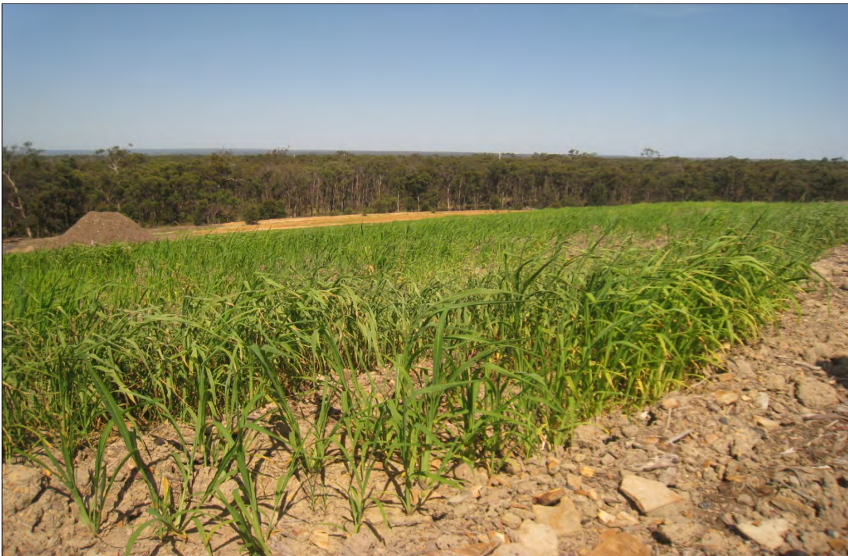
Plate 6 – Temporary REA batter stabilisation through planting with millet
