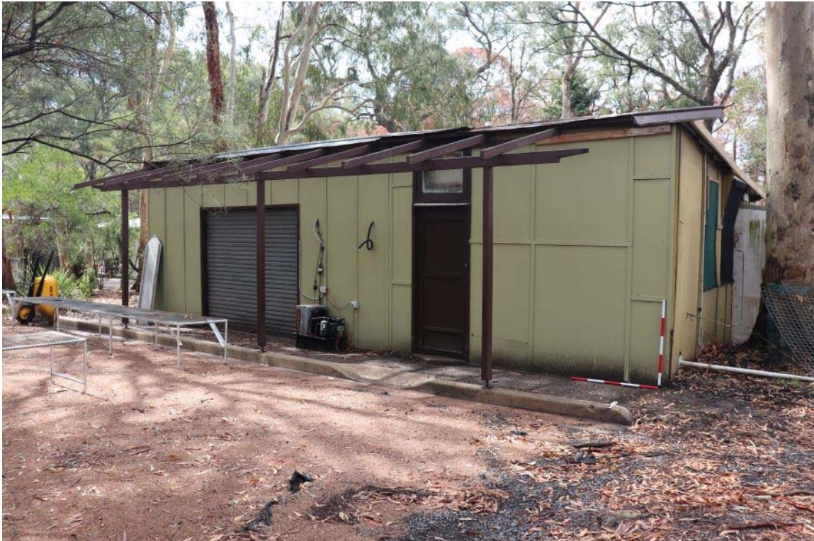
Plate A.6 Workshop/store, south elevation (BRE_600_pa04). View north-west.
