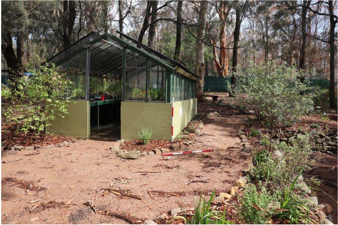
Plate A.5 Glasshouse (BRE_600_pa06). View south-west.
