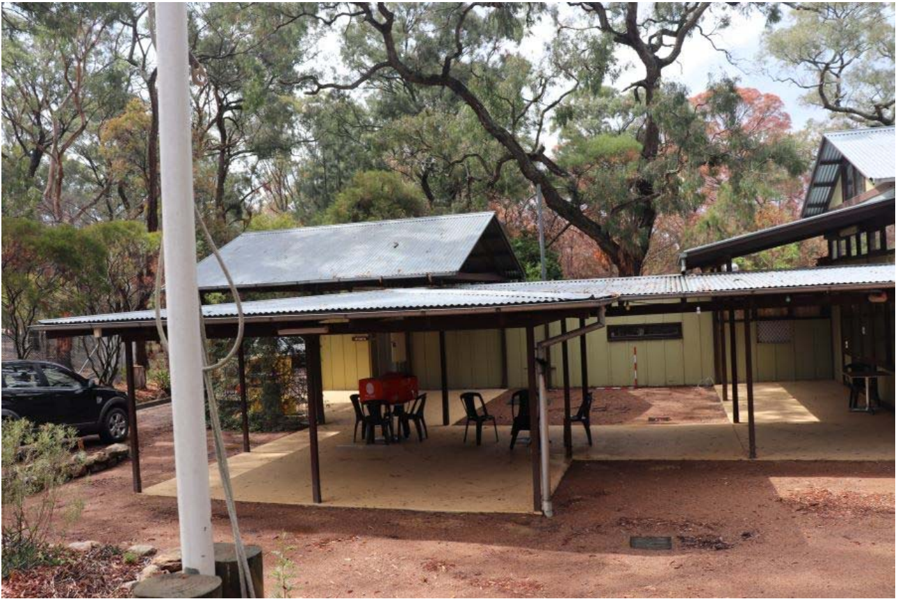
Plate 5.4 Visitor's Centre, south elevation, west. View north.
