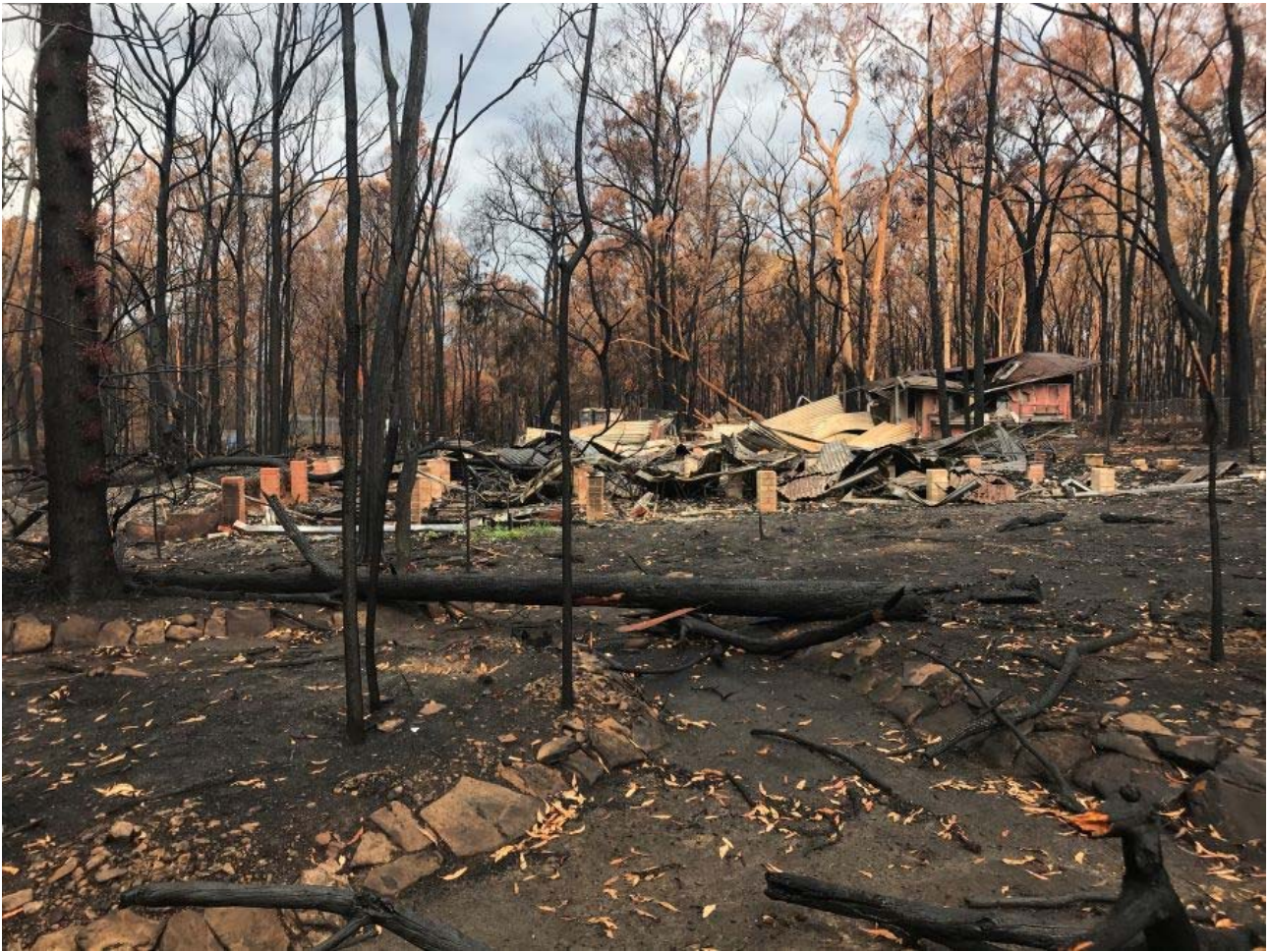
Plate 5.2 Fire damaged buildings in south of Wirrimbirra Sanctuary (BRE_580_pa01-05). View east.
