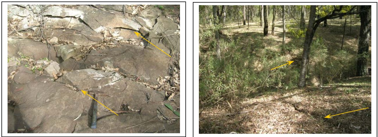
PHOTOGRAPH 9 Myrtle Creek Cracks
