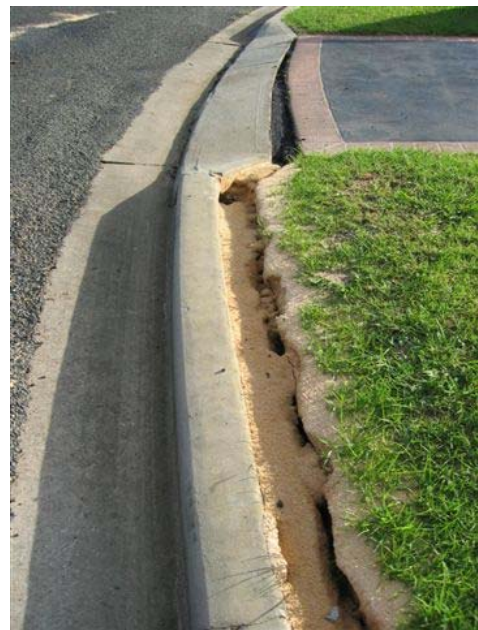
Gap formed between behind kerb on Winpara Close. Size of gap not seen above longwalls in other locations (Impact possibly due to anomalous non-systematic movement)
