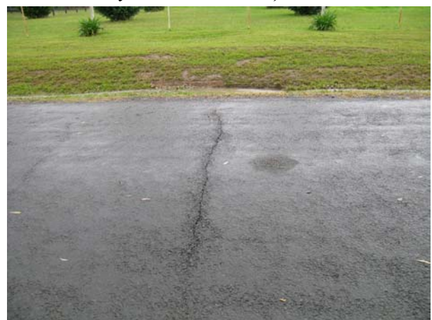
Impact to pavement on Brundah Road (Impact possibly due to anomalous non-systematic movement)
