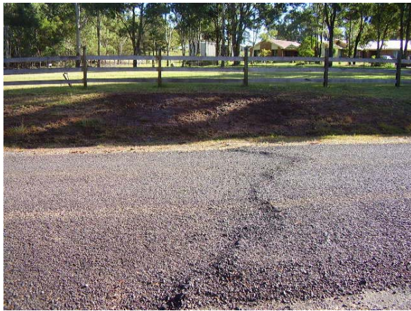
Impact to pavement on Glenanne Place. Repaired fence and water main beneath bare patch in grass beyond. Only water main damage above longwalls to date. (Impact possibly due to anomalous non-systematic movement)
