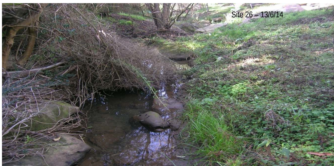
Figure 13 Site 20, 25 and 26 Subsidence Effects after Longwall 28 Extraction
