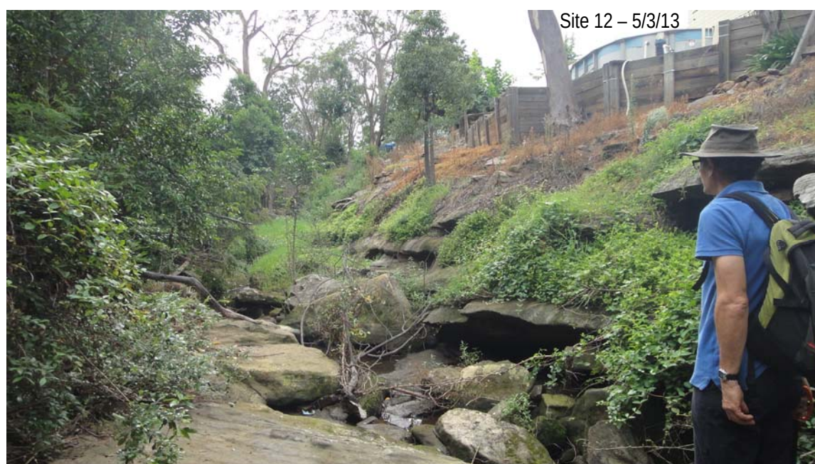
Figure 6 Site 9 and 12 Subsidence Effects after Longwall 26 Extraction
