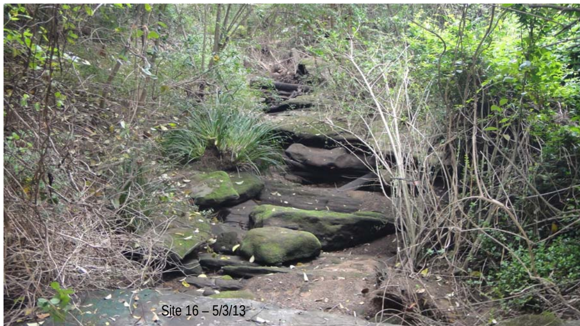
Figure 8 Site 15 and 16 Subsidence Effects after Longwall 26 Extraction
