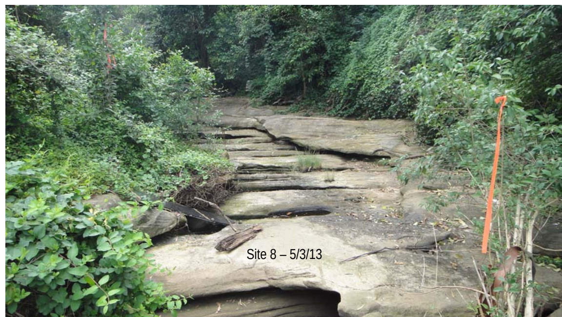
Figure 5 Site 7 and 8 Subsidence Effects after Longwall 26 Extraction
