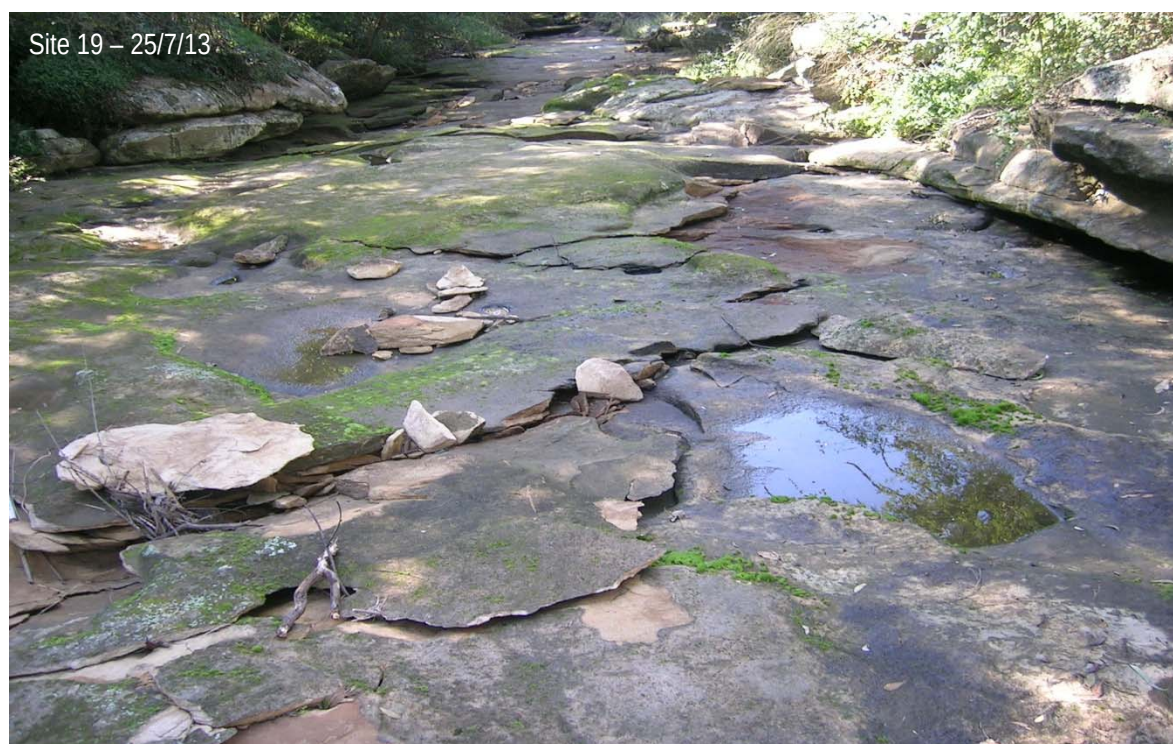
Figure 11 Site 18 and 19 Subsidence Effects after Longwall 27 Extraction
