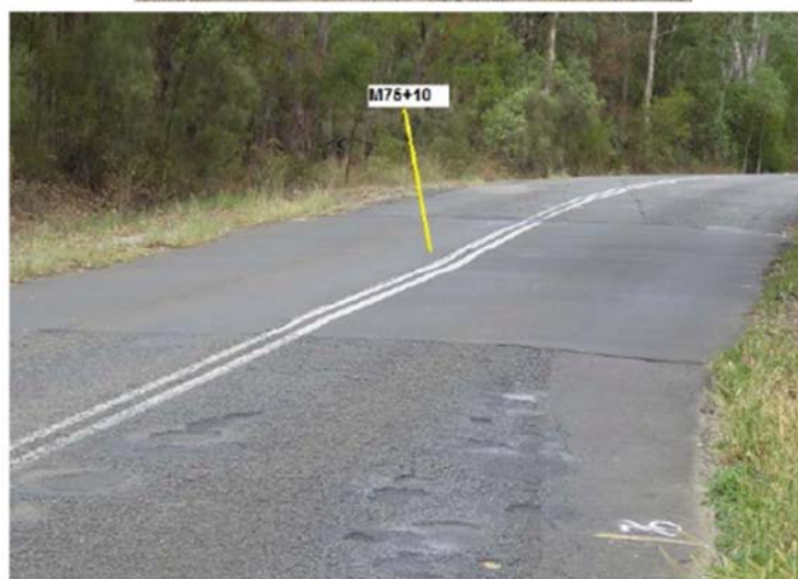
Fig. 4.1 Photographs of Impacts to Road Pavements and Kerbs during Longwall 29
