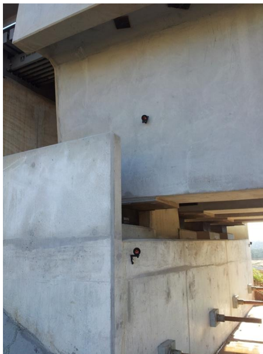
Fig. 2.9 Survey prisms located on abutment and bridge deck of Deviation Overbridge at 92.400 km
