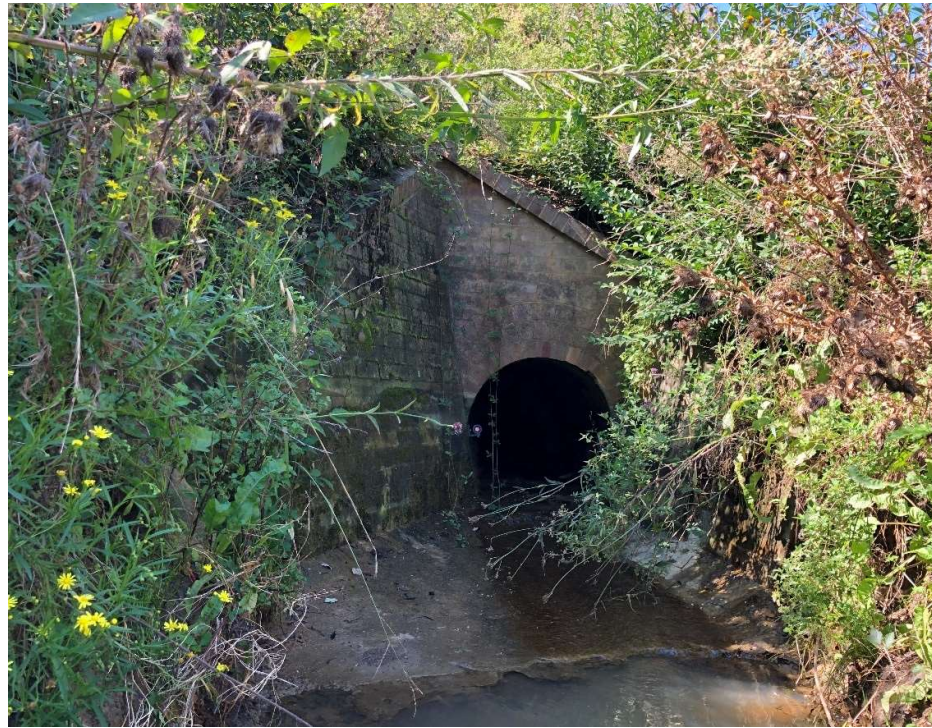
Western portal. In sound condition.
