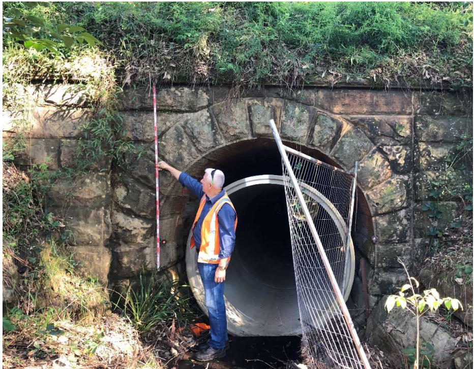
Eastern portal, generally in good condition.
