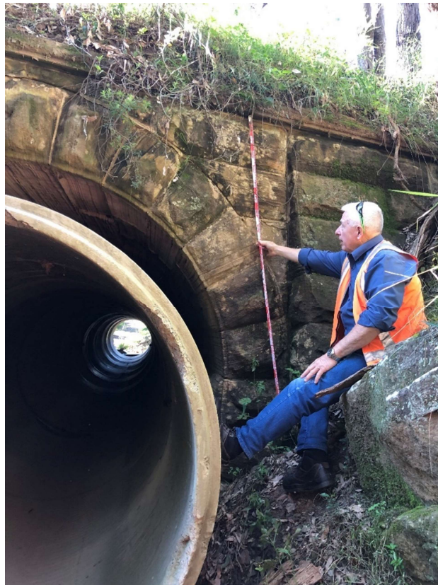
Western portal. Cracking around arch stones that was first noted during extraction of LW W2 has not worsened during LW W3.
