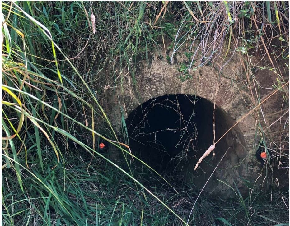
Eastern portal. Overgrown but appears to be in sound condition.
