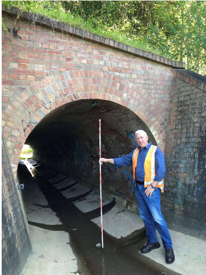
Eastern portal. Culvert is in good condition.
