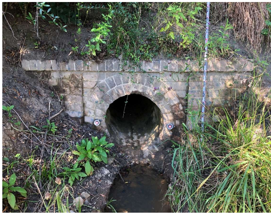
Western portal. In sound condition
