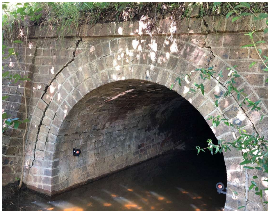
Northern portal. Difficult to access due to water and weeds. Pre-existing cracking around the arch, mostly through mortar.
