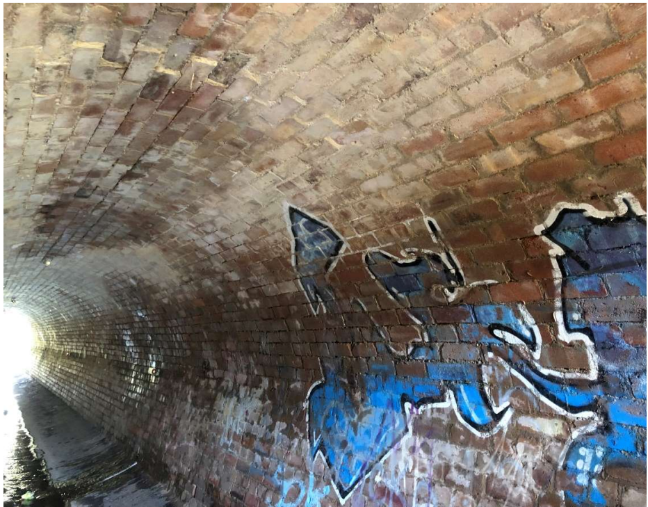
Roof of culvert. View west
