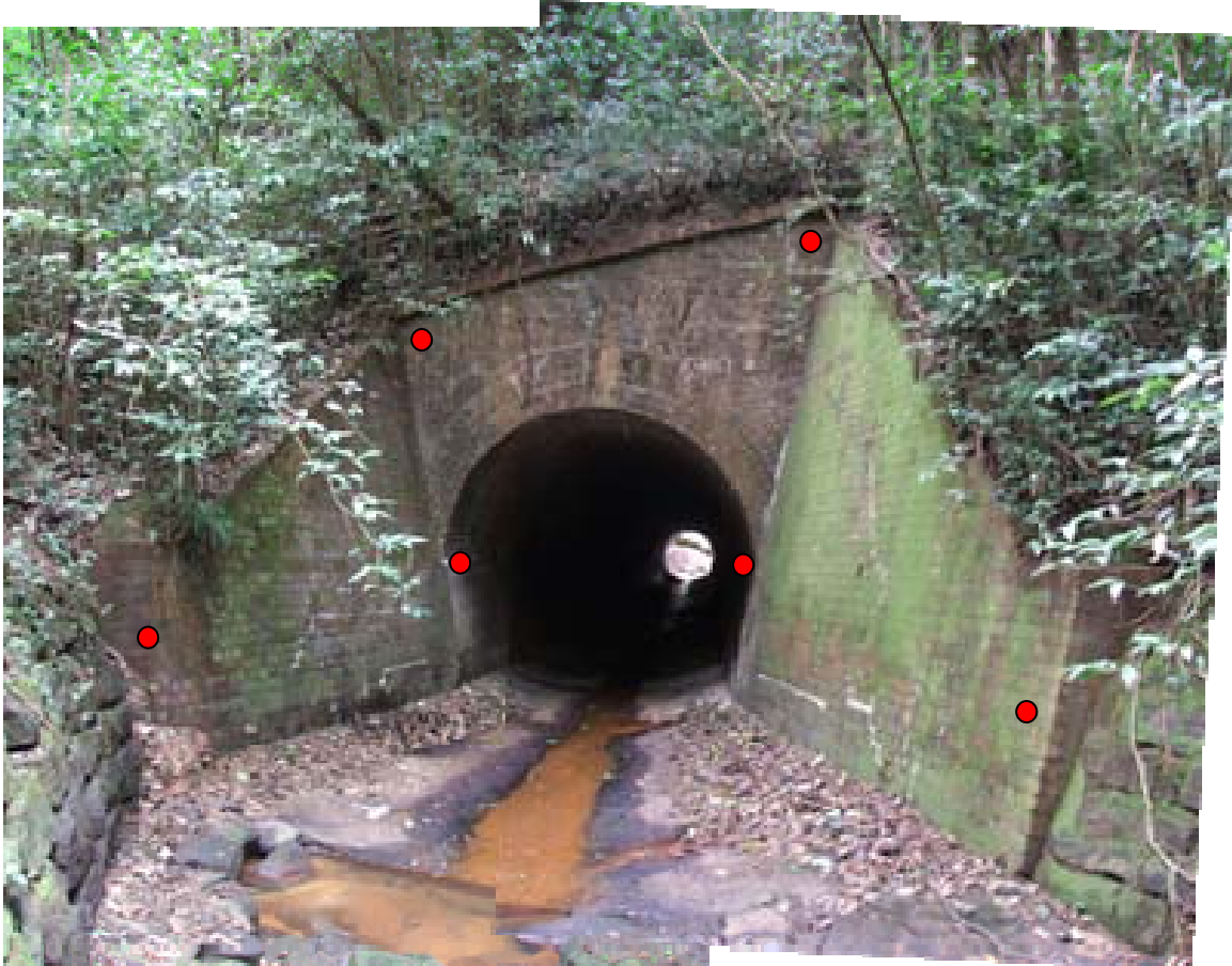
Fig. 2.4 Proposed locations of monitoring points at downstream headwall and wingwalls of the Redbank Creek Culvert
