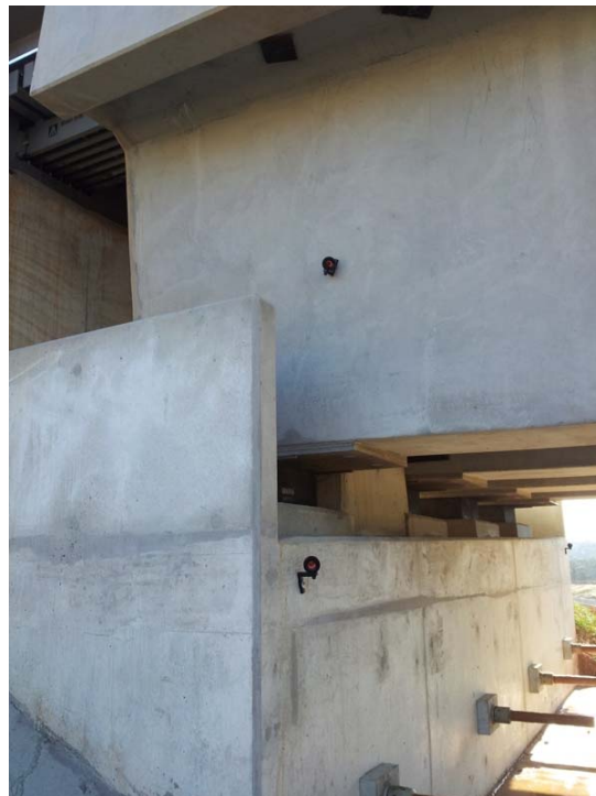
Fig. 2.3 Survey prisms located on abutment and bridge deck of Deviation Overbridge at 92.400 km
