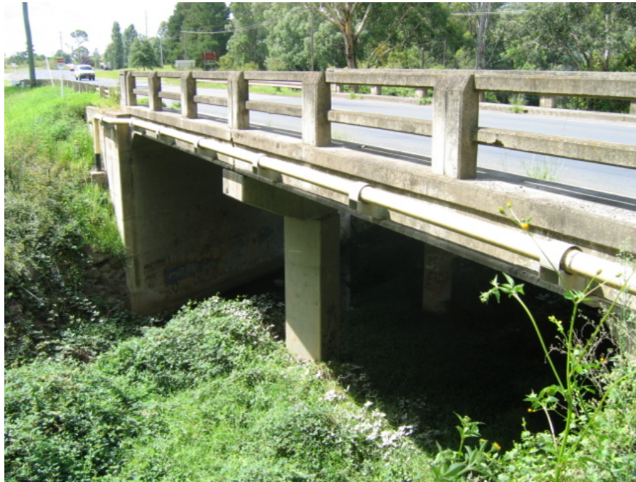
Fig. 3.12 Remembrance Drive Road Bridge over Myrtle Creek
