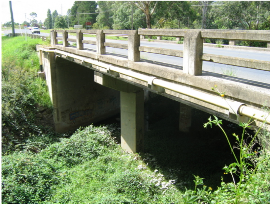
Fig. 3.15 Remembrance Drive Road Bridge over Myrtle Creek
