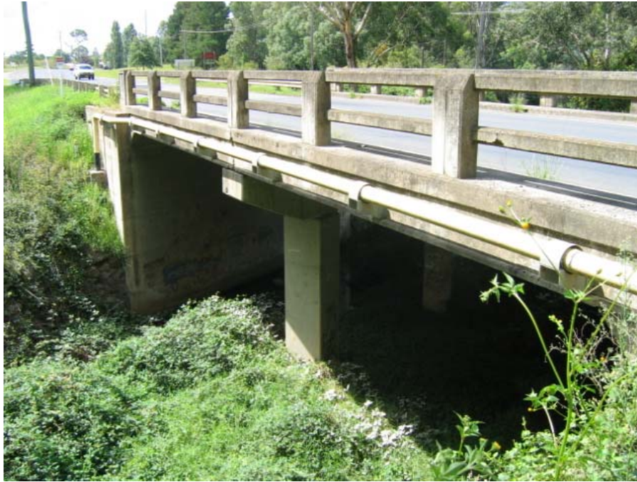
Fig. 3.8 Remembrance Drive Road Bridge over Myrtle Creek
