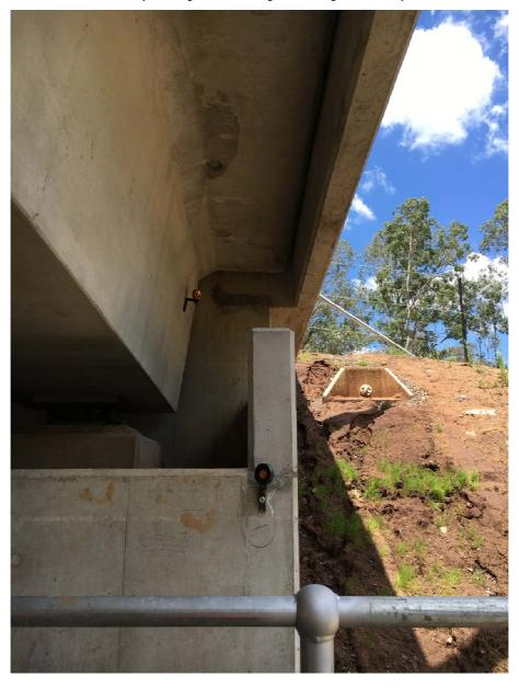
Fig. 2.12 Survey prisms located on abutment and bridge deck of Deviation Overbridge at 92.400 km
