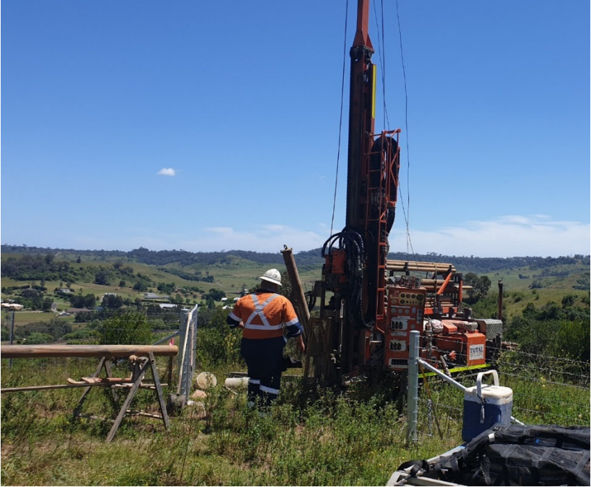
Fig. 3.7 Drilling of borehole at Picton Tunnel
