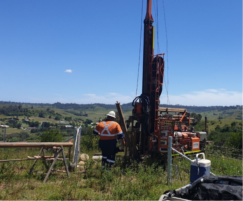
Fig. 3.7 Drilling of borehole at Picton Tunnel
