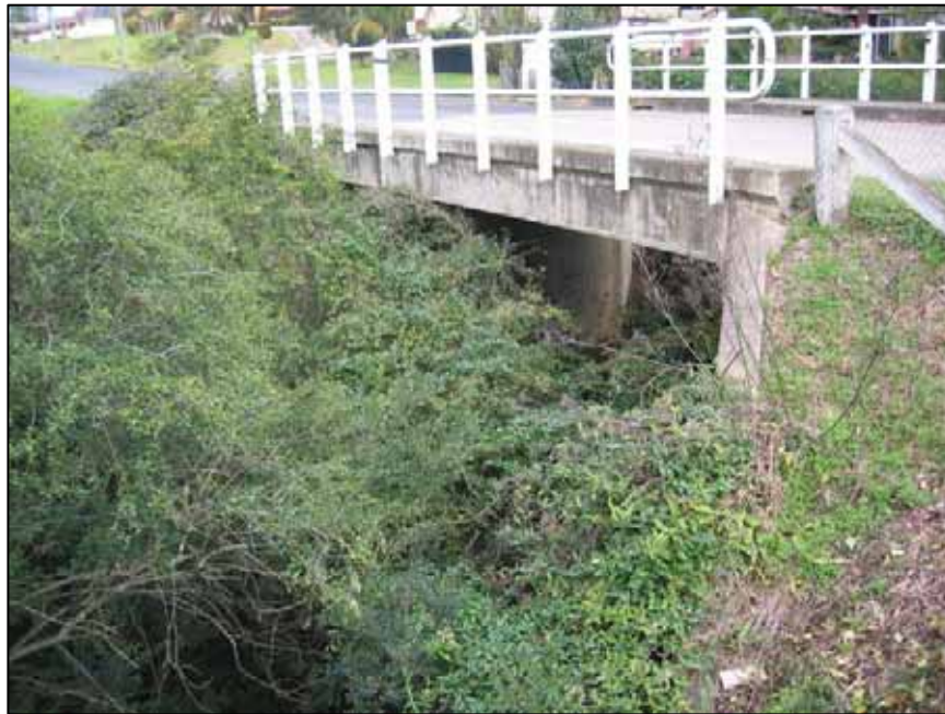
Fig. 4.4 Castlereagh Street Road Bridge over Myrtle Creek
