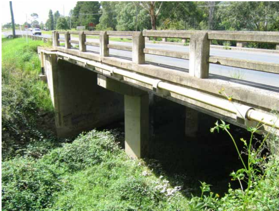
Fig. 4.11 Remembrance Drive (Myrtle Creek) Road Bridge
