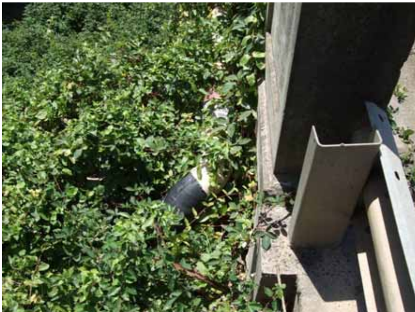
Figure 10 Gas pipeline emerging from the ground next to the southwest corner of bridge
