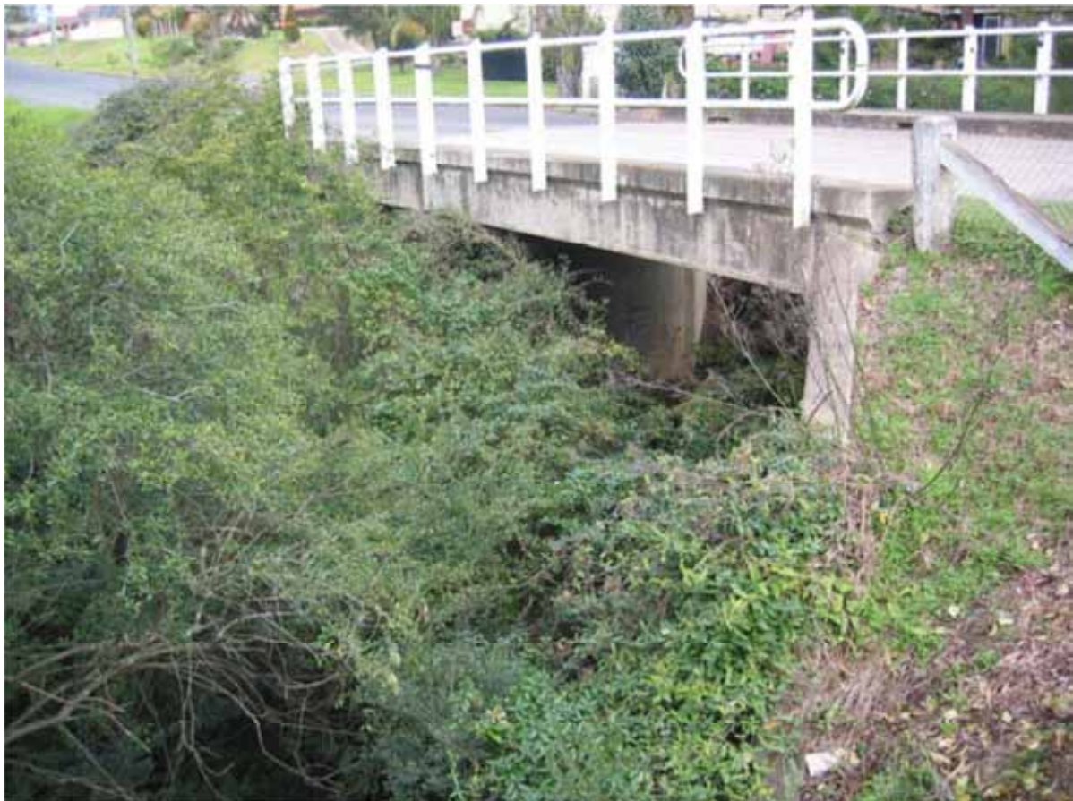
Figure 1 – Castlereagh Street Bridge over Myrtle Creek.
