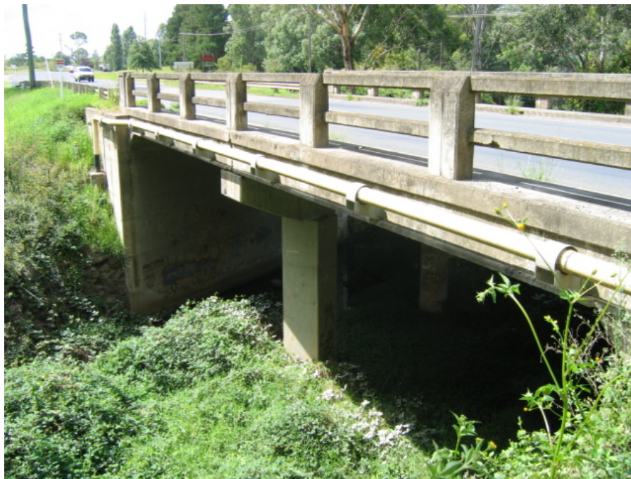
Fig. 3.10 Remembrance Drive Road Bridge over Myrtle Creek
