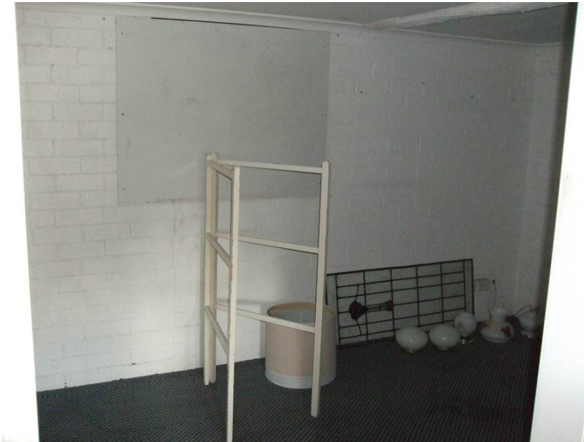
Figure 23 Underside of roughhewn hardwood beam, which is supported by the new brickwork
