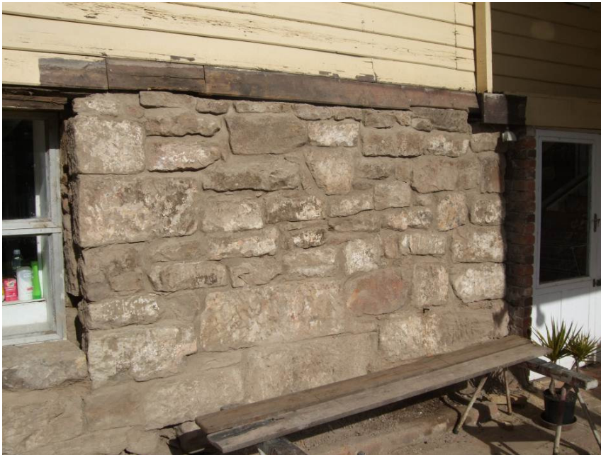
Figure 11 Repaired foundation wall outside laundry at the northwestern corner of the dwelling contrast with the damage evident in figure 50 in Appendix D after the brick veneer wall was demolished
