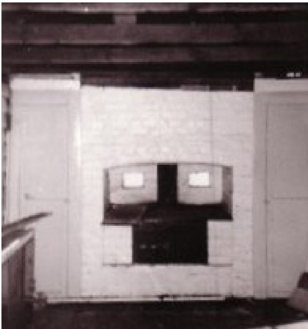
Figure 51 Exposed ceiling joists in kitchen located in the northwestern corner of the dwelling taken during the restoration than began in 1972.
