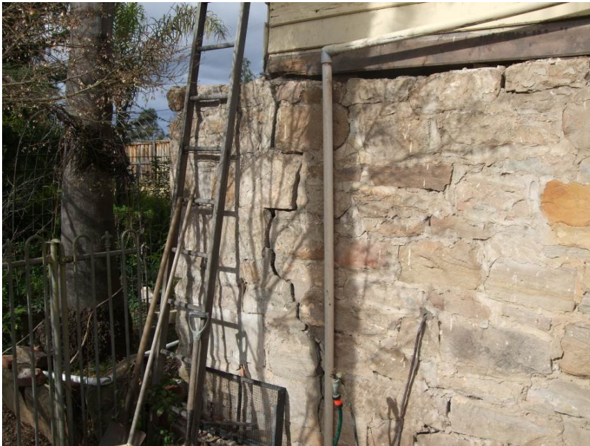
Figure 9 the northwestern corner of the foundation wall outside the laundry prior to repair
