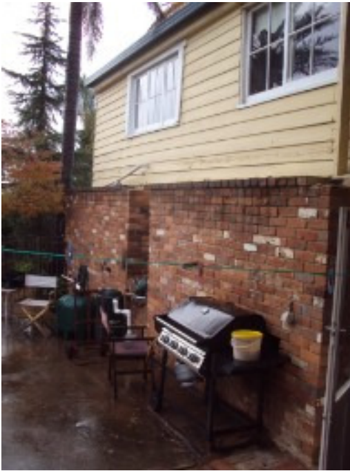
Figure 48 looking back towards northwestern corner of dwelling before recent renovations began
