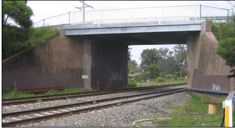
Fig. 3.3 Thirlmere Way Railway Overbridge
