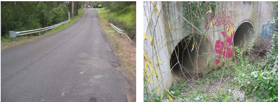
Fig. 3.11 Photographs of Elphin Street Road Culvert at Myrtle Creek
