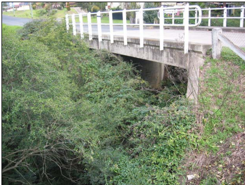
Fig. 3.4 Castlereagh Street Road Bridge over Myrtle Creek
