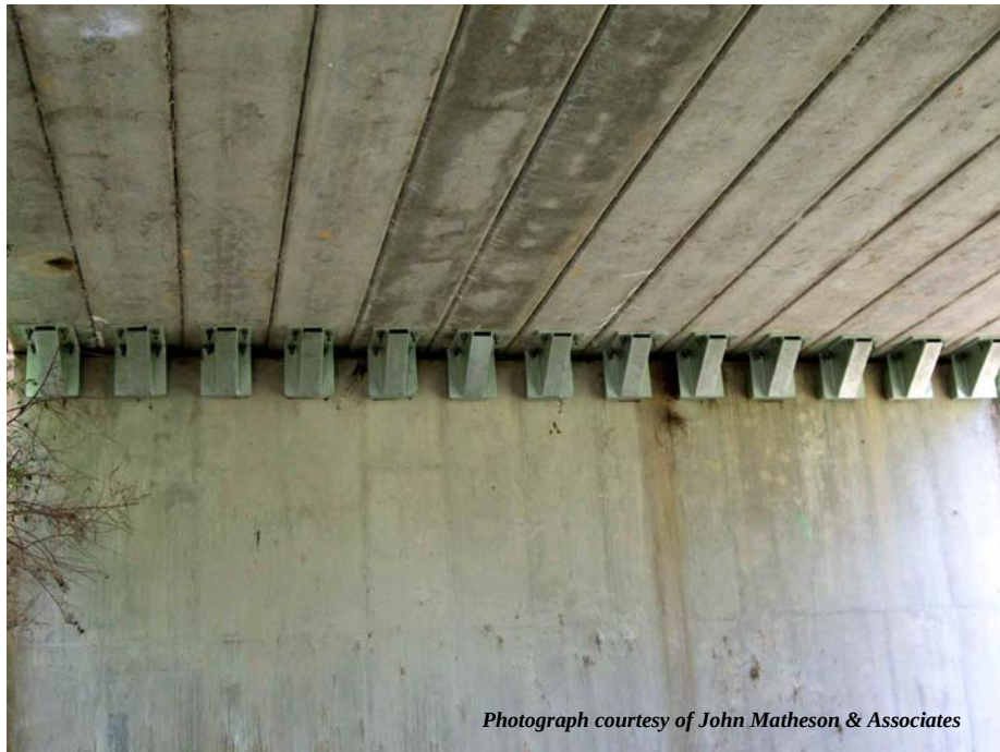
Fig. 3.13 Photograph of Installed Brackets at Castlereagh Street Bridge
