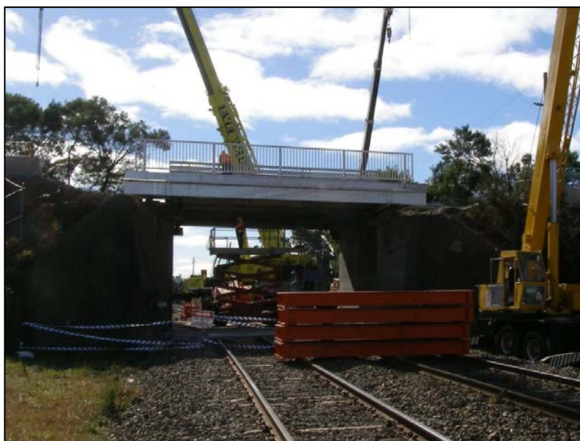
Fig. 3.4 Thirlmere Way Railway Overbridge
