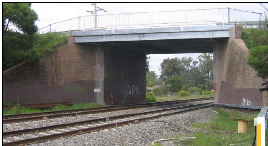
Fig. 1.1 Thirlmere Way Railway Overbridge
