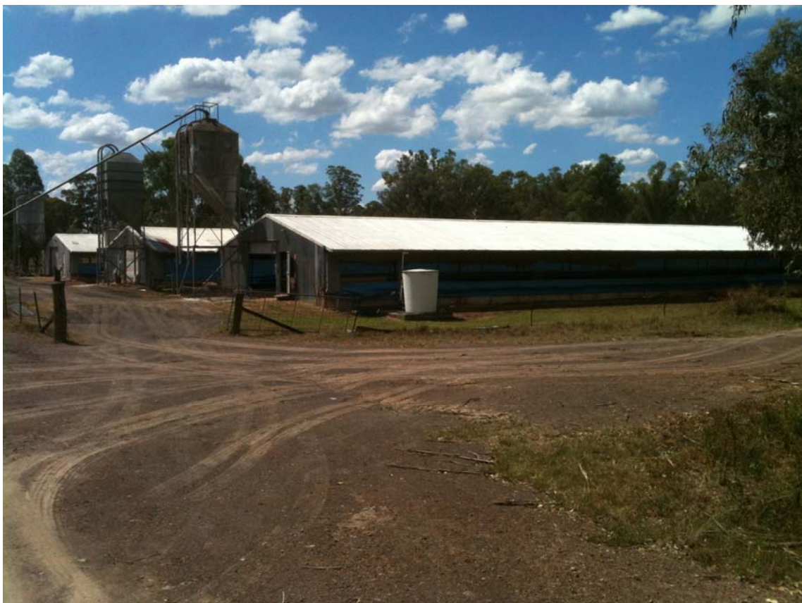
Fig. 1.3 Duck sheds viewed from south
