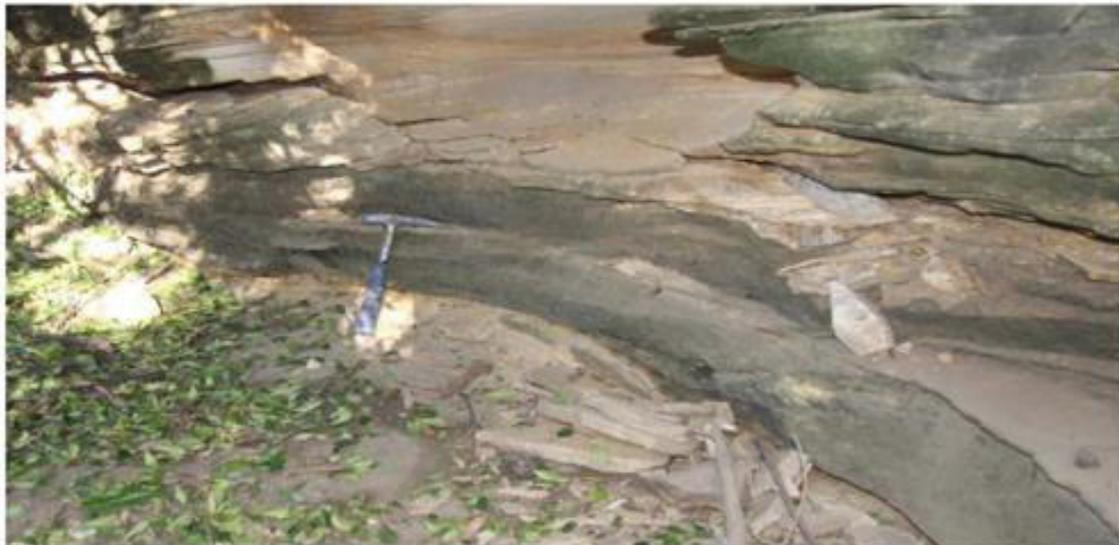
Figure 30 Myrtle Creek over LW25 – cracking
