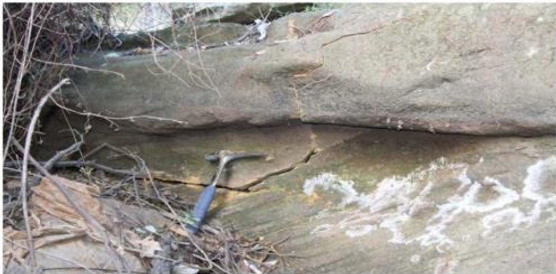
*Figure 29 Myrtle Creek over LW25 – cracking*
