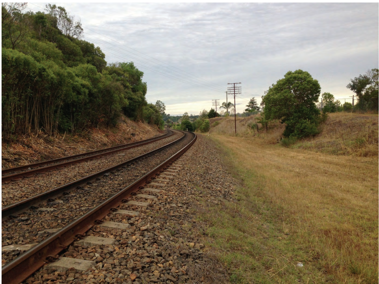
Fig. 6.19 Railway Cutting 89.470 km to 89.650 km above Longwall 32 looking north
