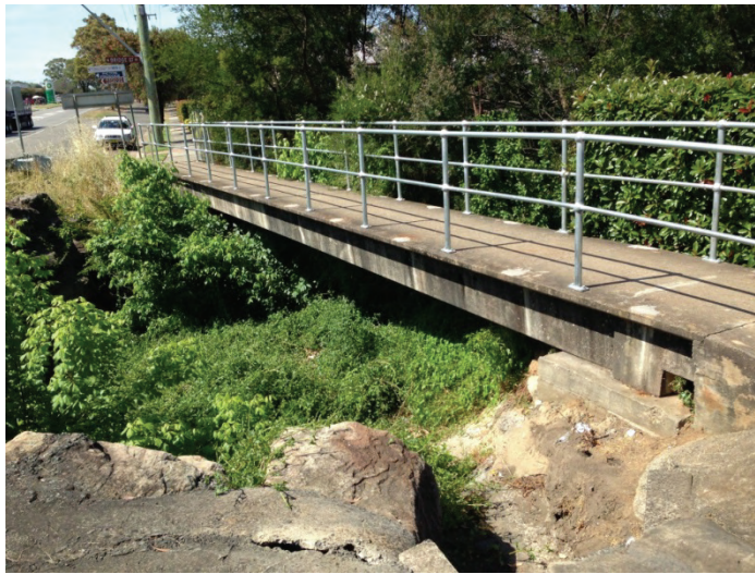
Fig. 6.32 Remembrance Footbridge over Redbank Creek
