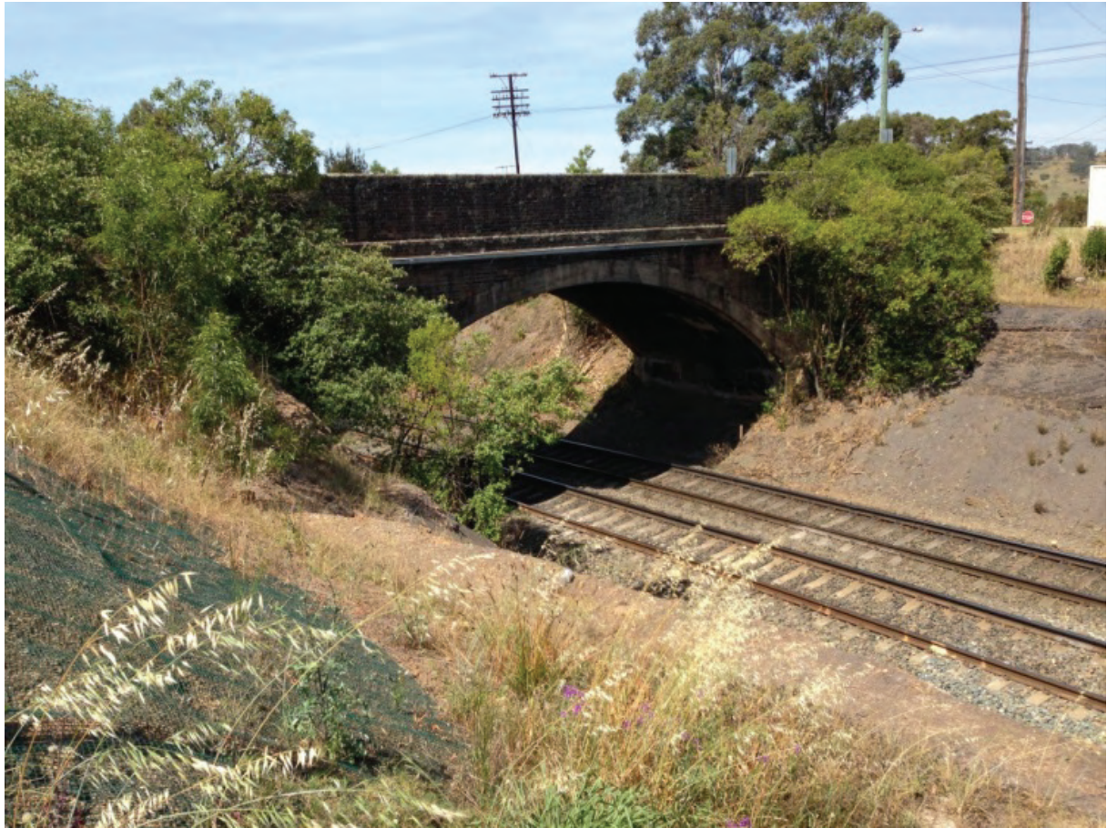
Fig. 6.7 Connellan Crescent Railway Overbridge at 89.080 km
