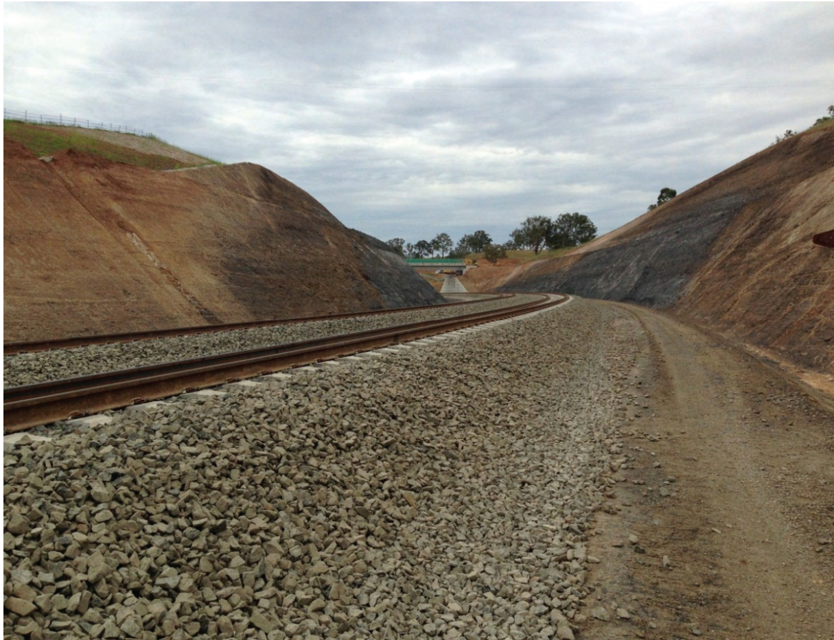
Fig. 6.22 Deviation cutting looking north, prior to the installation of flexible erosion protection measures
