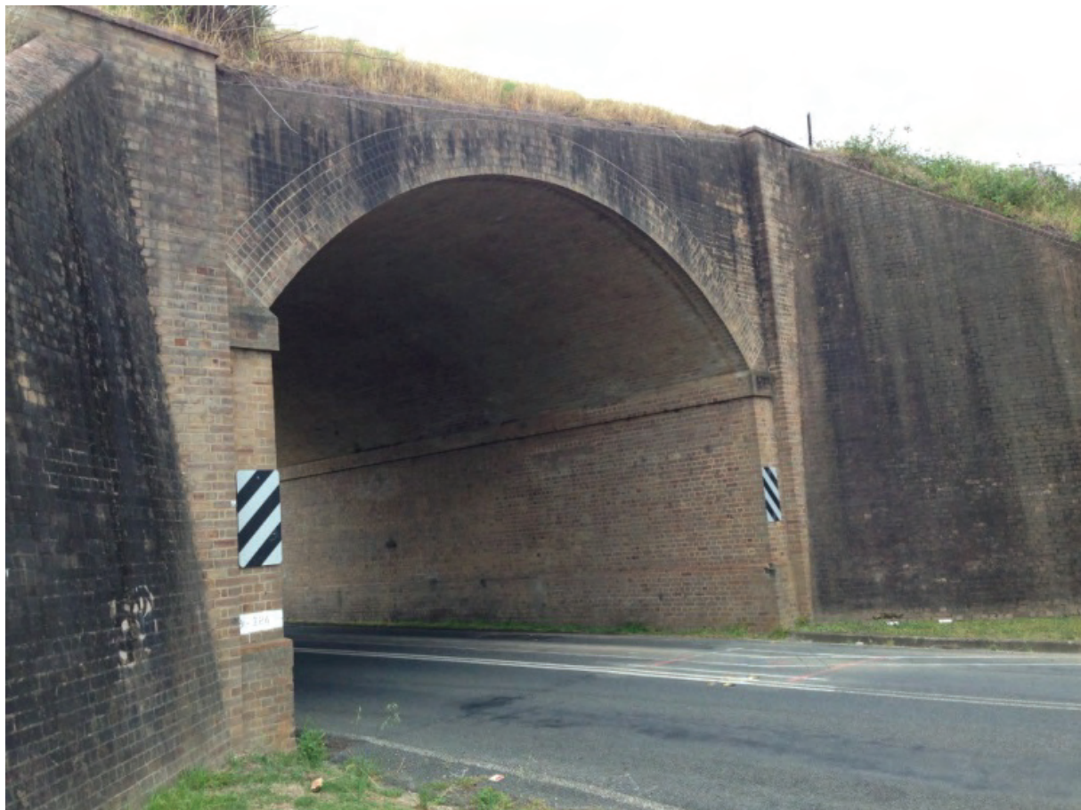
Fig. 6.6 Thirlmere Way Rail Underbridge at 89.326 km
