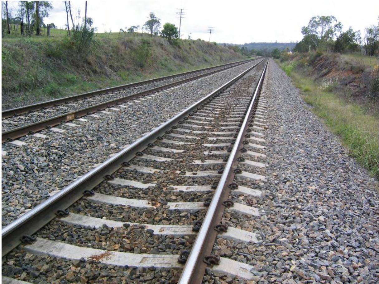
Fig. 6.20 Railway Cutting 90.370 km to 90.500 km above Longwall 31 looking north
