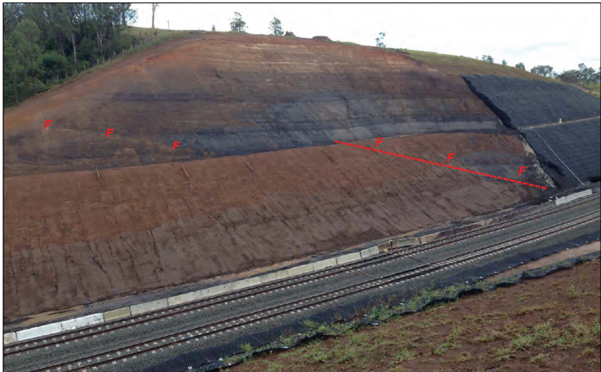
Fig. 6.22 Deviation cutting looking north, prior to the installation of flexible erosion protection measures
