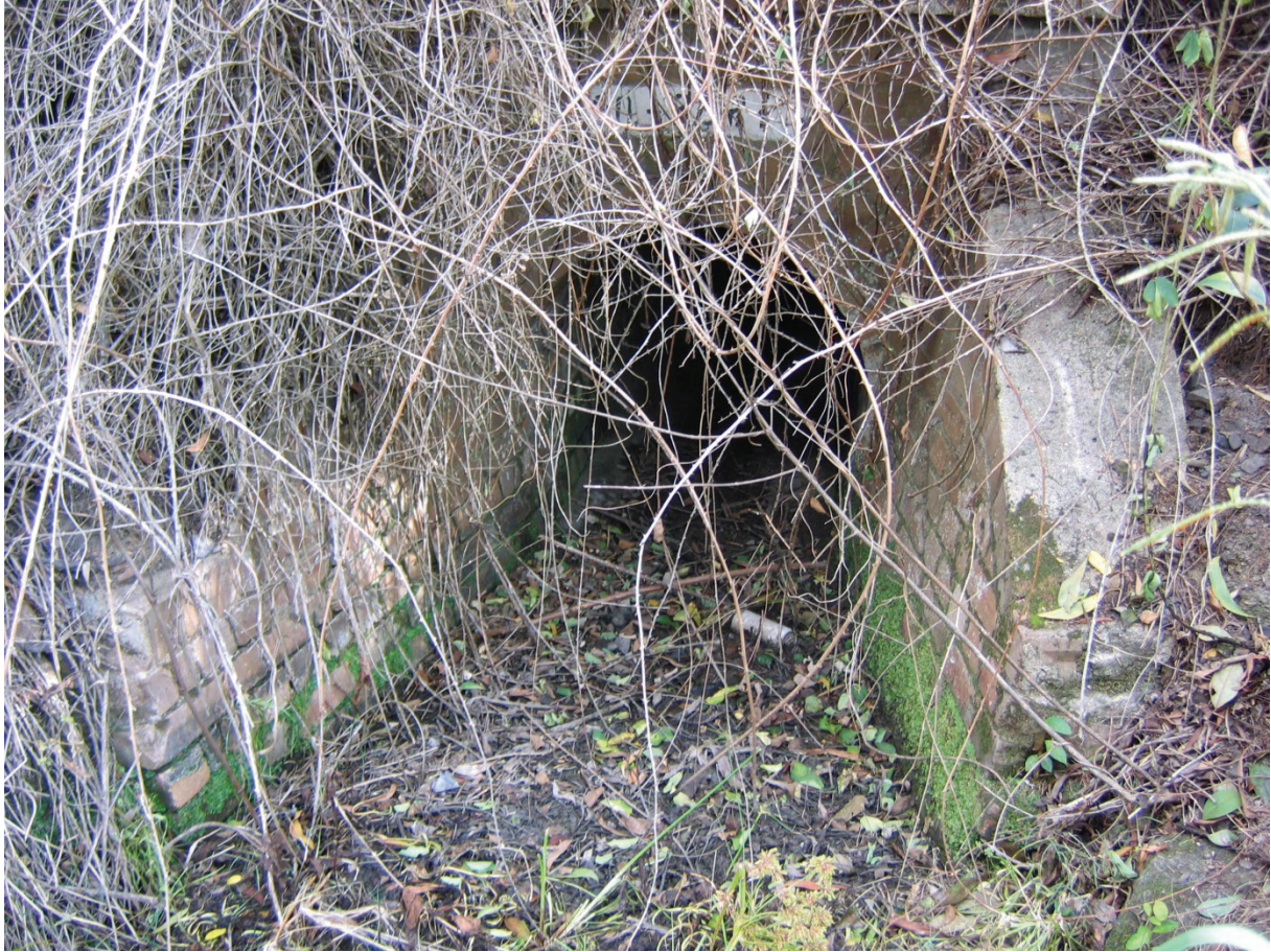
Fig. 6.11 Culvert at 90.252 km above proposed Longwall 32
