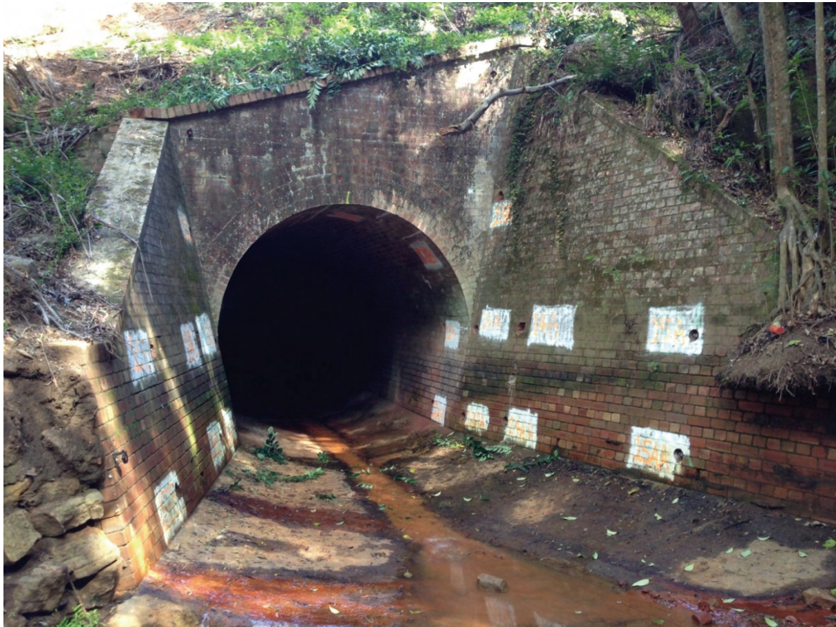
Fig. 6.10 Redbank Creek Railway Culvert at 91.265 km
