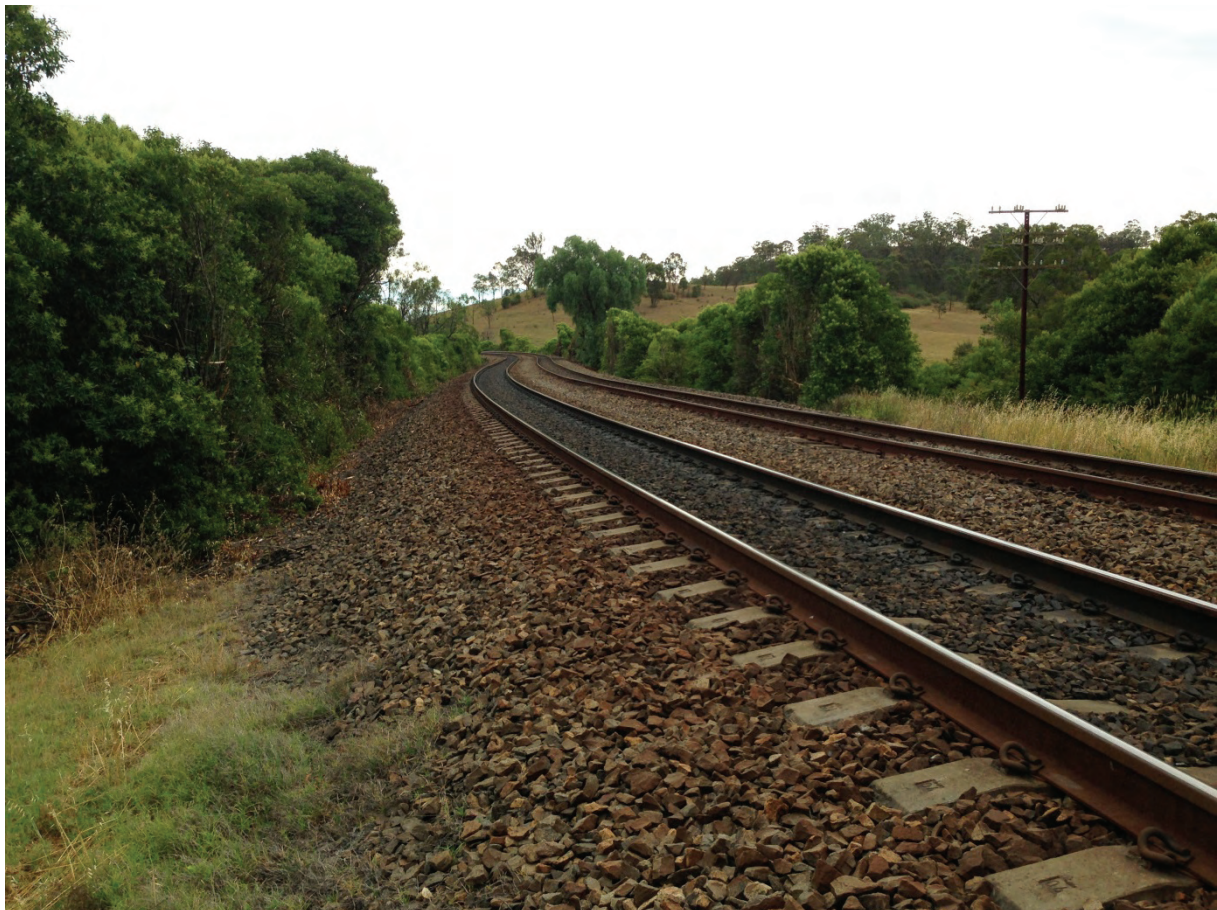
Fig. 6.1 View of Main Southern Railway looking south from 89.785 km
