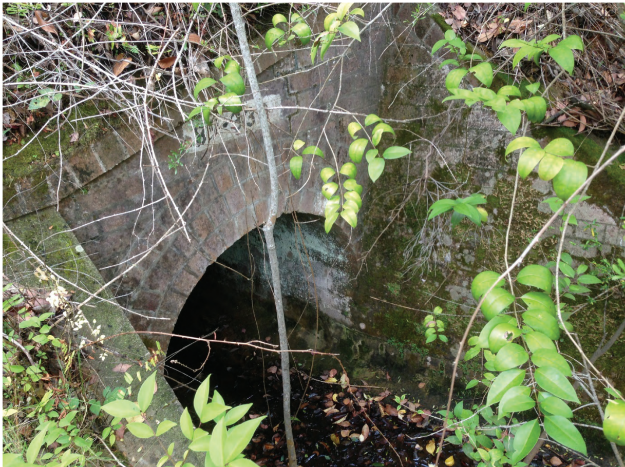
Fig. 6.25 Loop Line Culvert at 87.330 km
