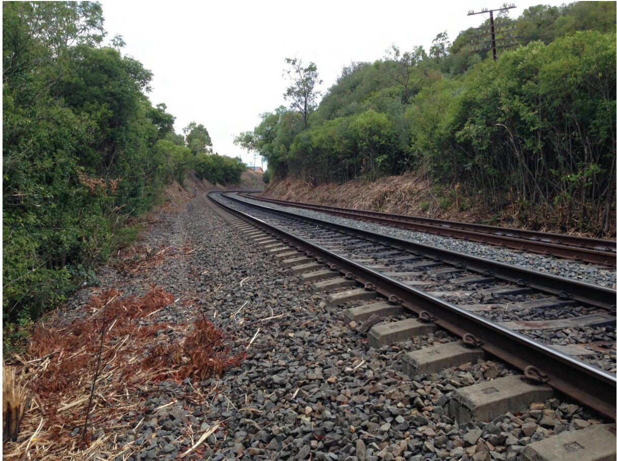
Fig. 6.18 Connellan Crescent Overbridge Railway Cutting 89.740 km to 89.040 km looking south
