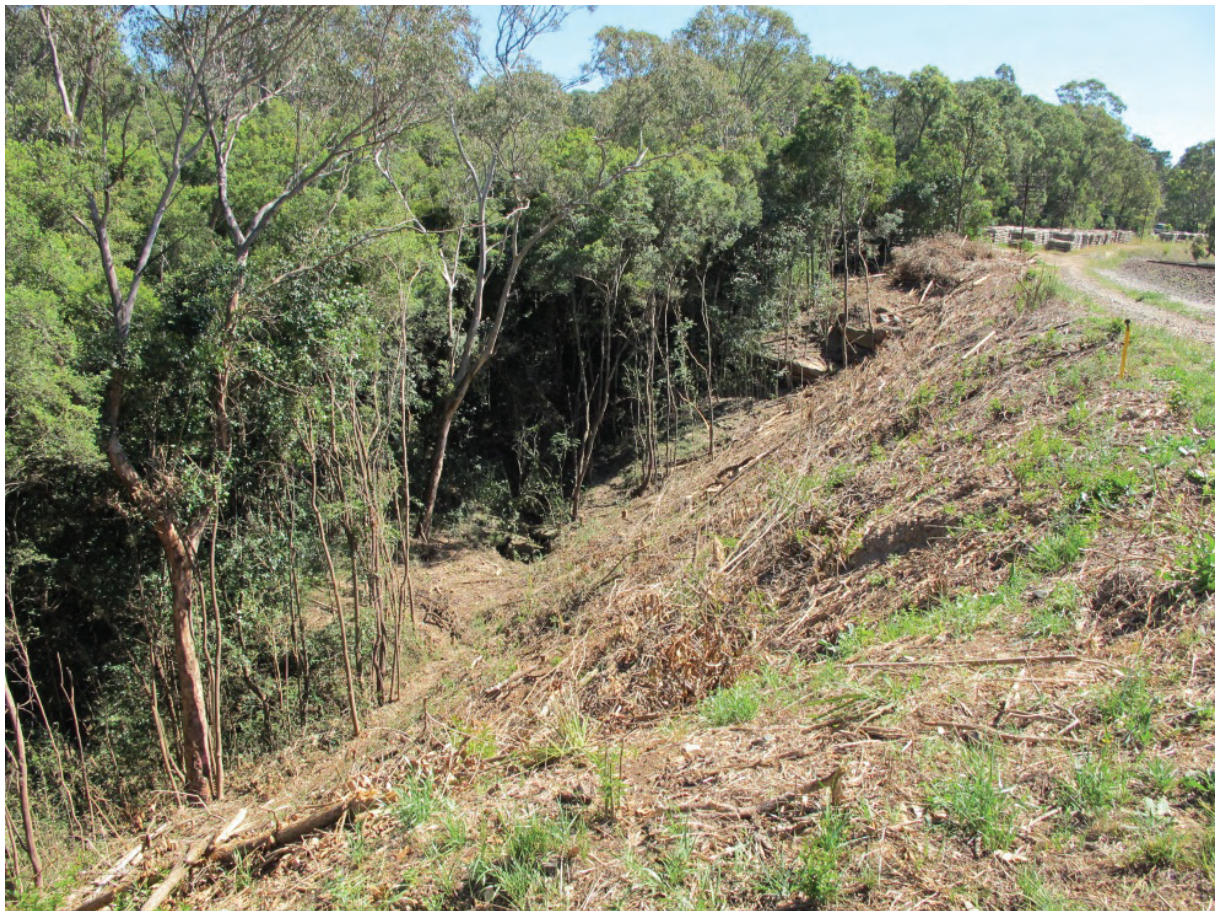
Fig. 6.16 Embankment on Up side (upstream side) of Redbank Creek embankment at 91.265 km
