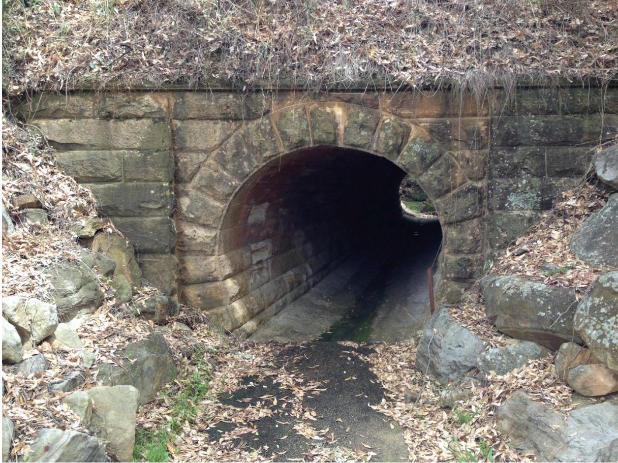
Fig. 6.28 Loop Line Culvert at 88.980 km
