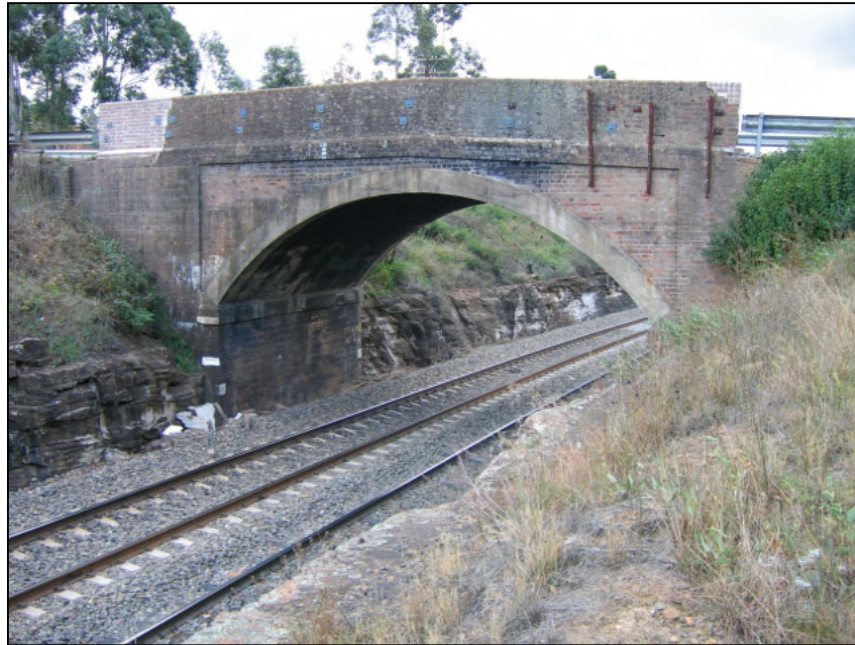
Fig. 6.5 Bridge Street Railway Overbridge at 91.000 km
