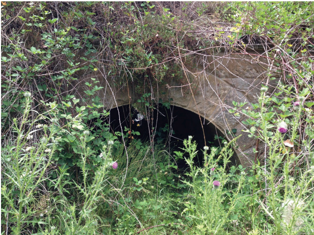
Fig. 6.27 Loop Line Culvert at 88.400 km
