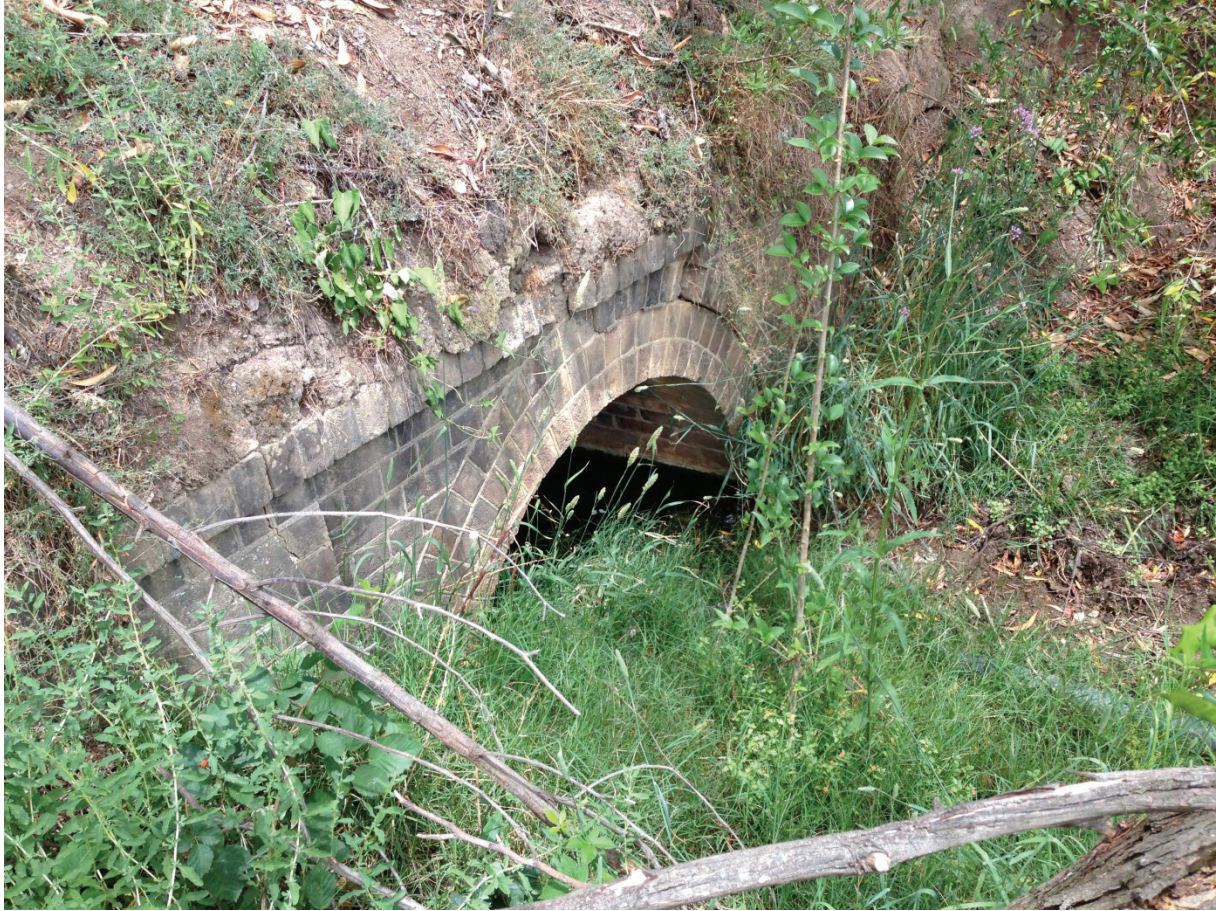
Fig. 6.26 Loop Line Culvert at 87.850 km
