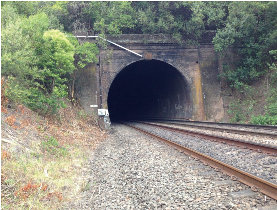
Fig. 6.35 Picton Rail Tunnel
