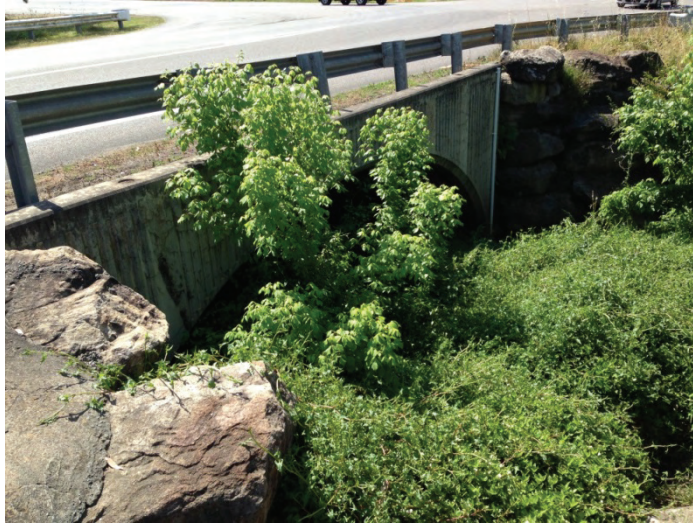
Fig. 6.31 Remembrance Drive Road Bridge over Redbank Creek (RE-B1)
