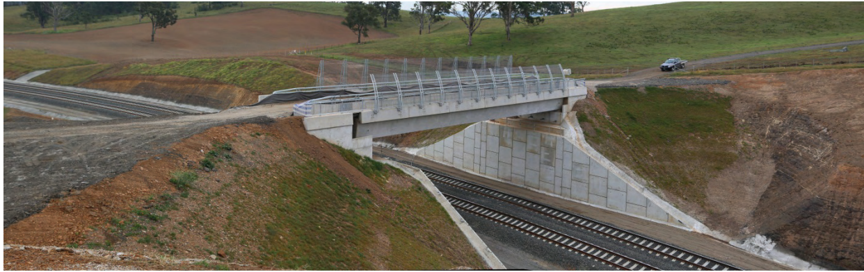
Fig. 6.4 Photograph of the Railway Deviation Overbridge at 92.410 km and the Reinforced Soil Wall Viewed from the Western Side
