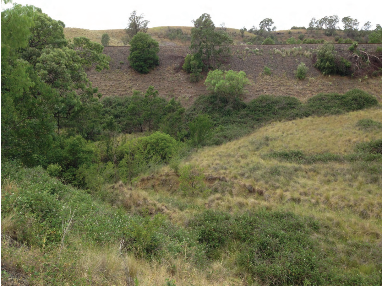
Fig. 6.13 Embankment on Up side (downstream side) of embankment at 87.331 km
