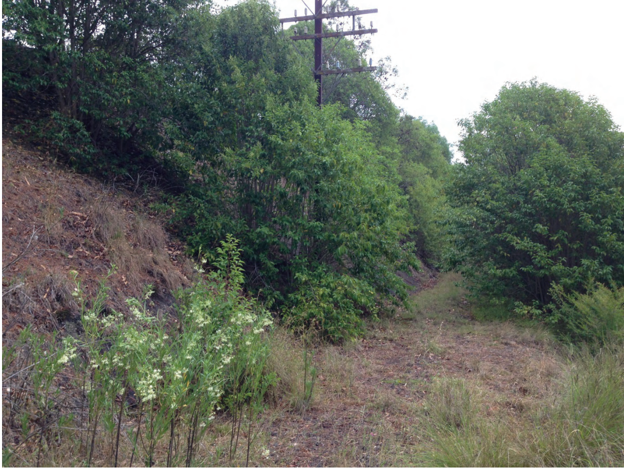
Fig. 6.15 Embankment on Up side (upstream side) of embankment at 89.785 km
