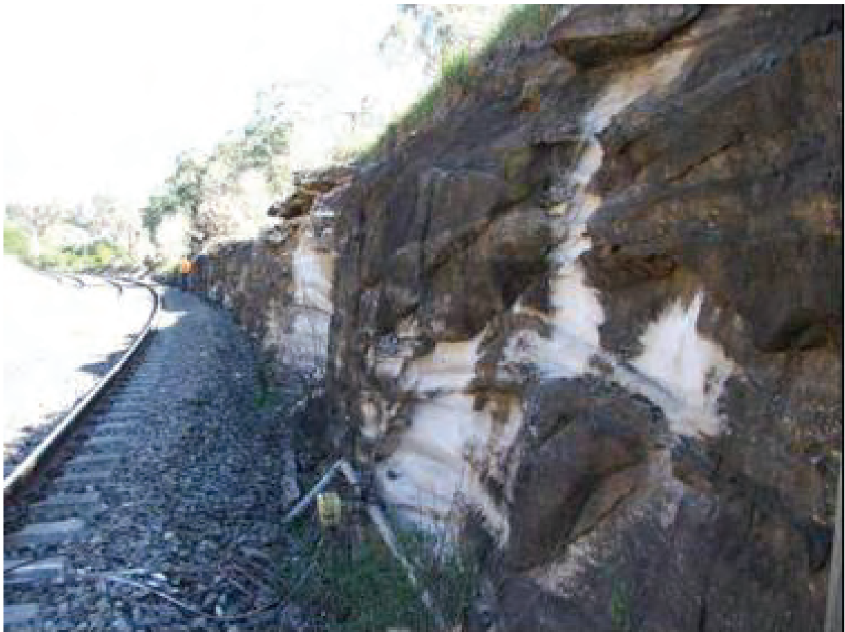
Fig. 6.21 Railway Cutting beneath Bridge St Overbridge at 91.000 km looking south
