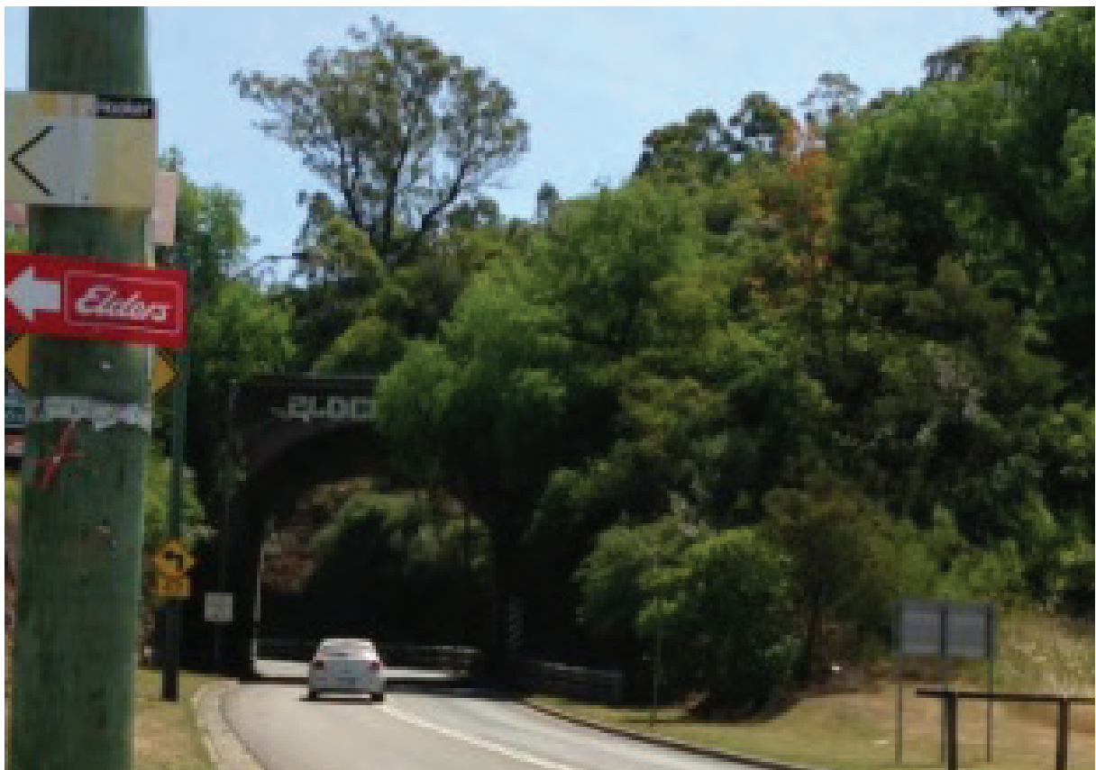
Fig. 6.8 Argyle Street Rail Underbridge at 86.13 km
