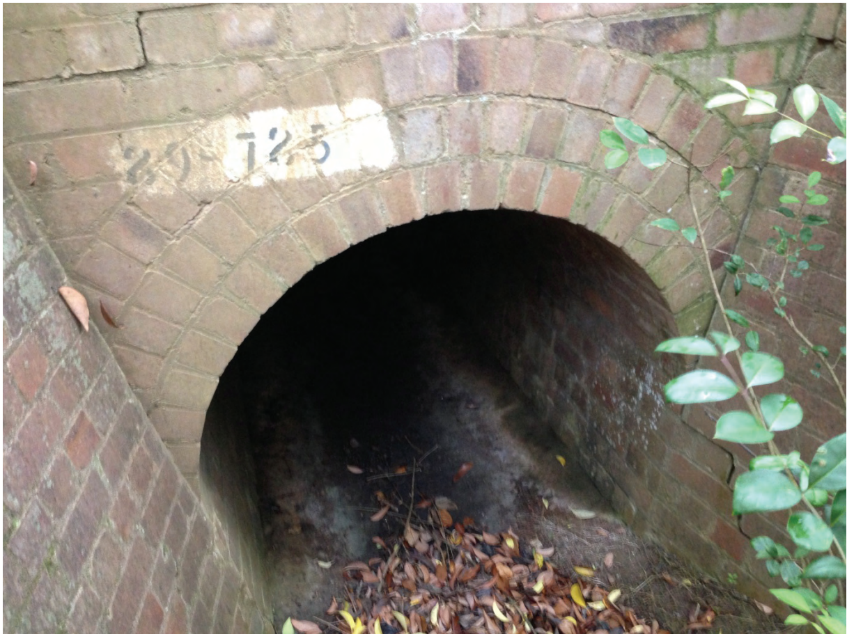
Fig. 6.12 Culvert at 89.785 km adjacent to proposed Longwall 32
