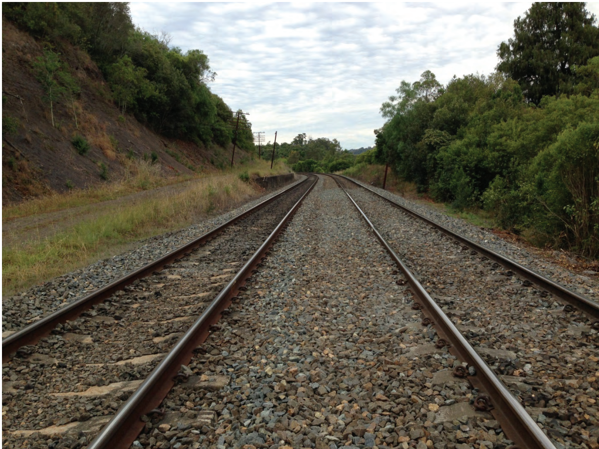
Fig. 6.17 Railway Cutting 88.290 km to 88.430 km looking north to disused concrete platform
