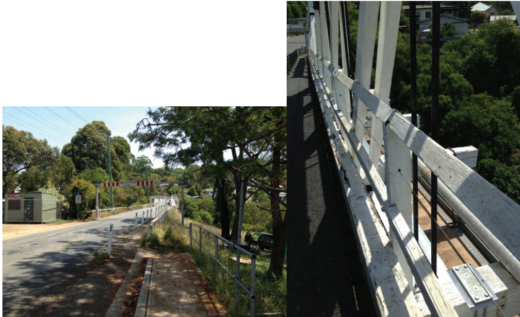
Fig. 6.33 Victoria Bridge over Stonequarry Creek
