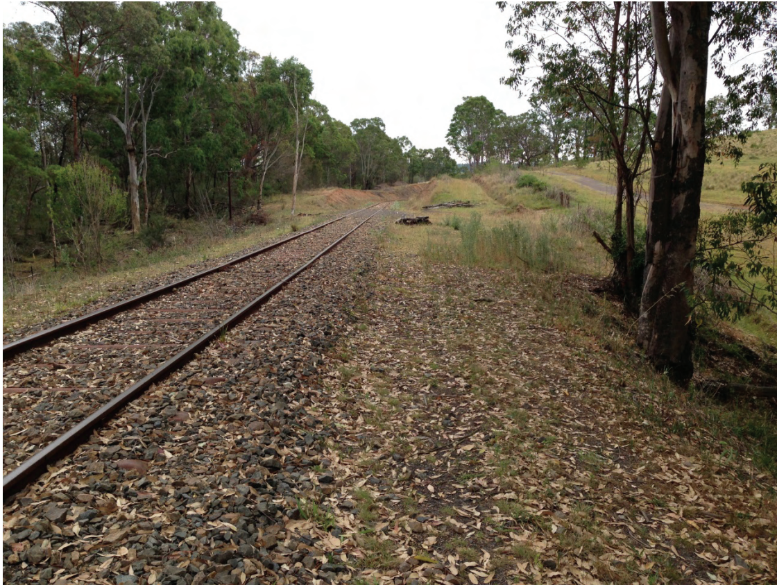
Fig. 6.24 Picton to Mittagong Loop Line at 88.980 km looking north
