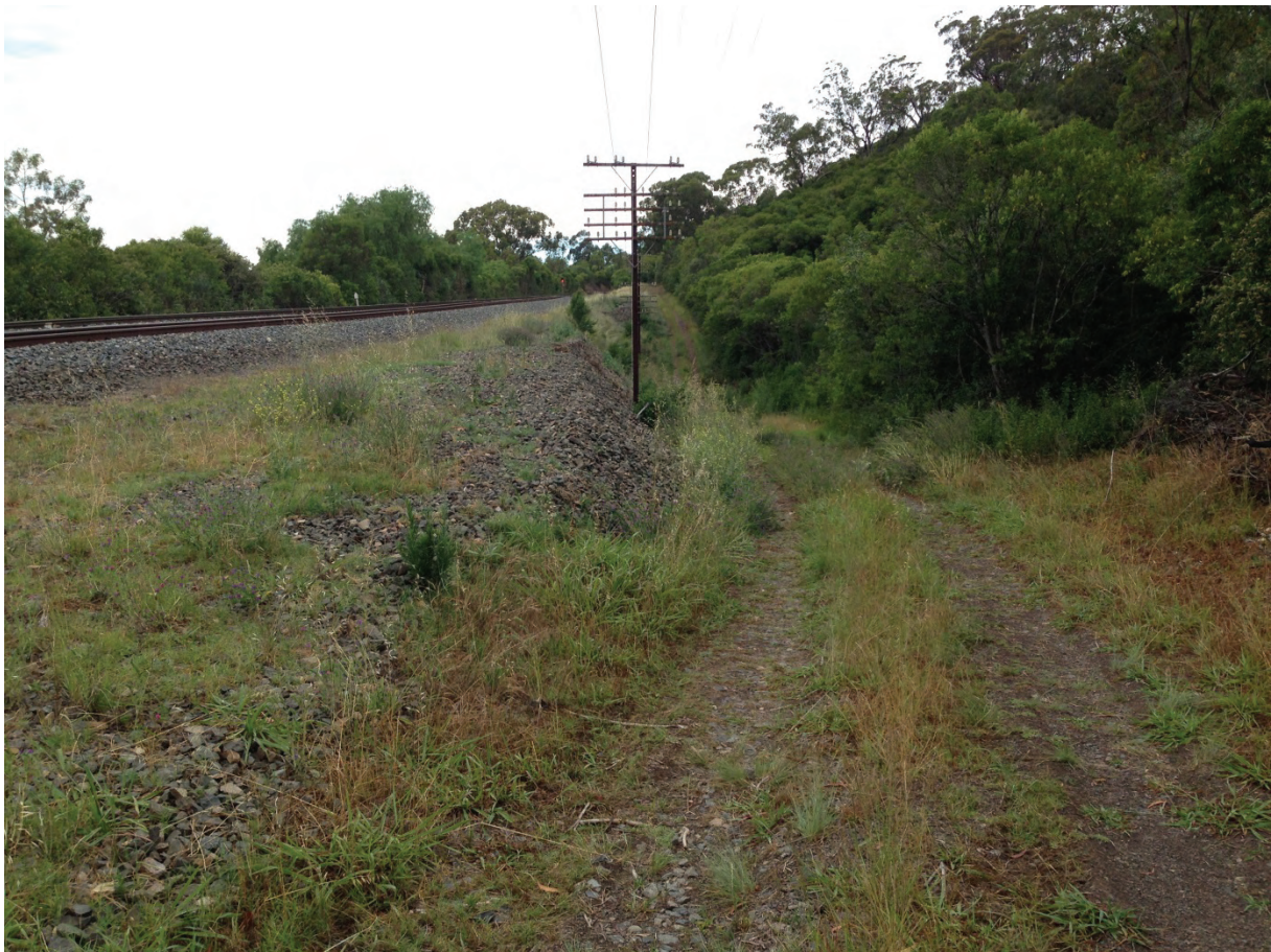
Fig. 6.14 Embankment on Up side (upstream side) of embankment at 88.496 km
