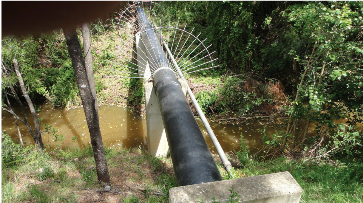
Fig. 6.39 Pipe Aqueduct for Thirlmere Carrier over Redbank Creek
