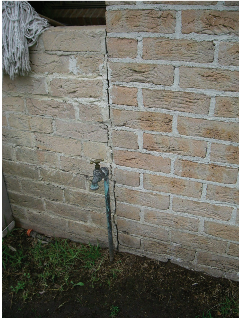
Fig. C.2 Example of crack in mortar only
