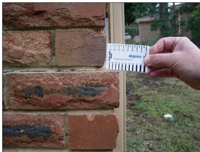
Fig. C.1 Example of slippage on damp proof course
