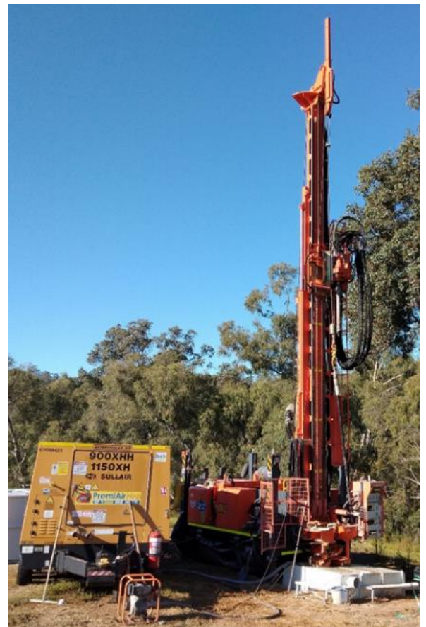
Typical Drill Rig for Characterisation Drilling
