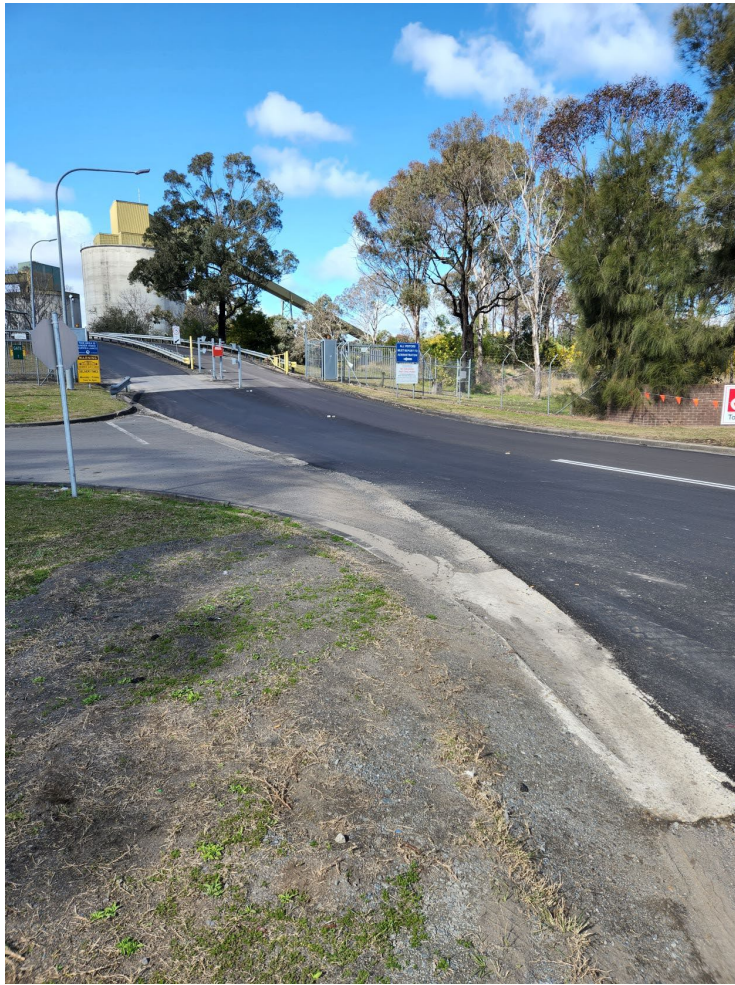
Photo 1 - Re-sealed mine access road with concrete drains
