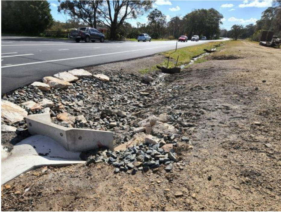
Photo 3 - Concrete and rock-lined drain with haybales for sediment control
