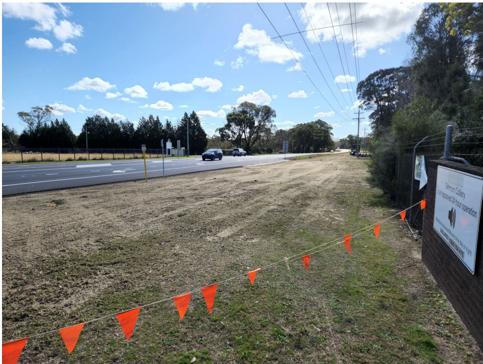
Photo 2 - Temporary stabilisation applied to exposed areas
