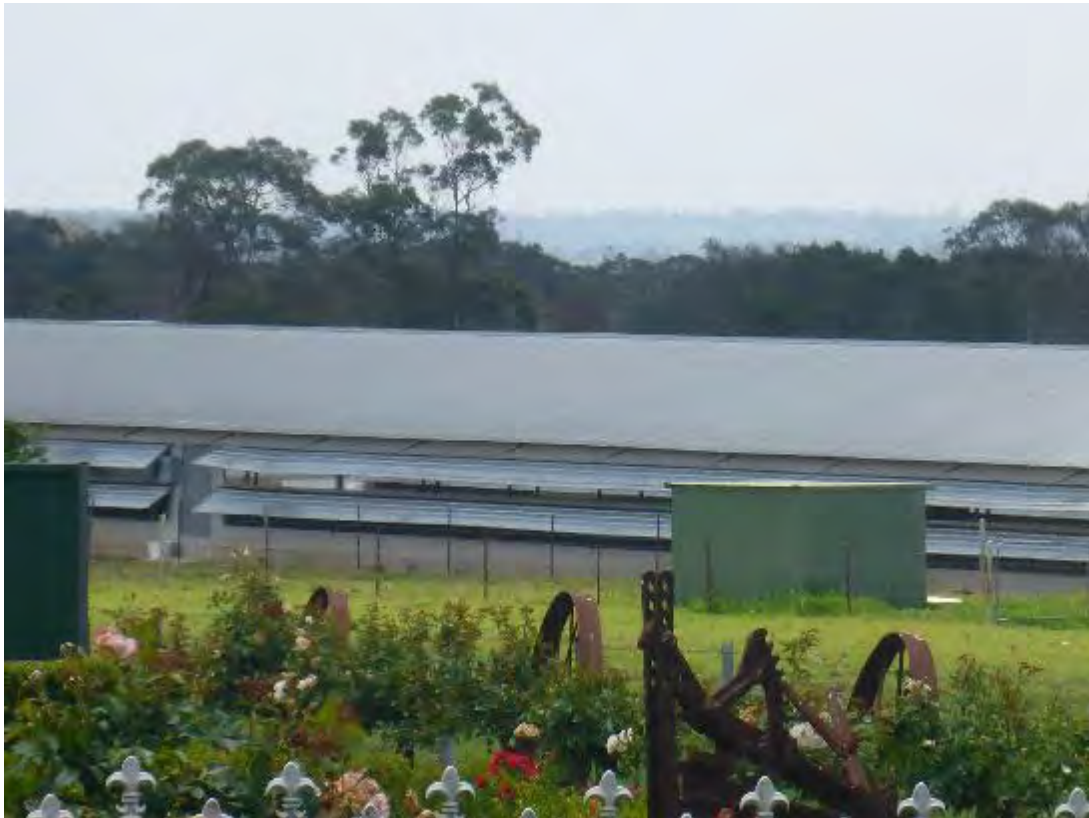
Plate 1 Poultry sheds at Site 55
