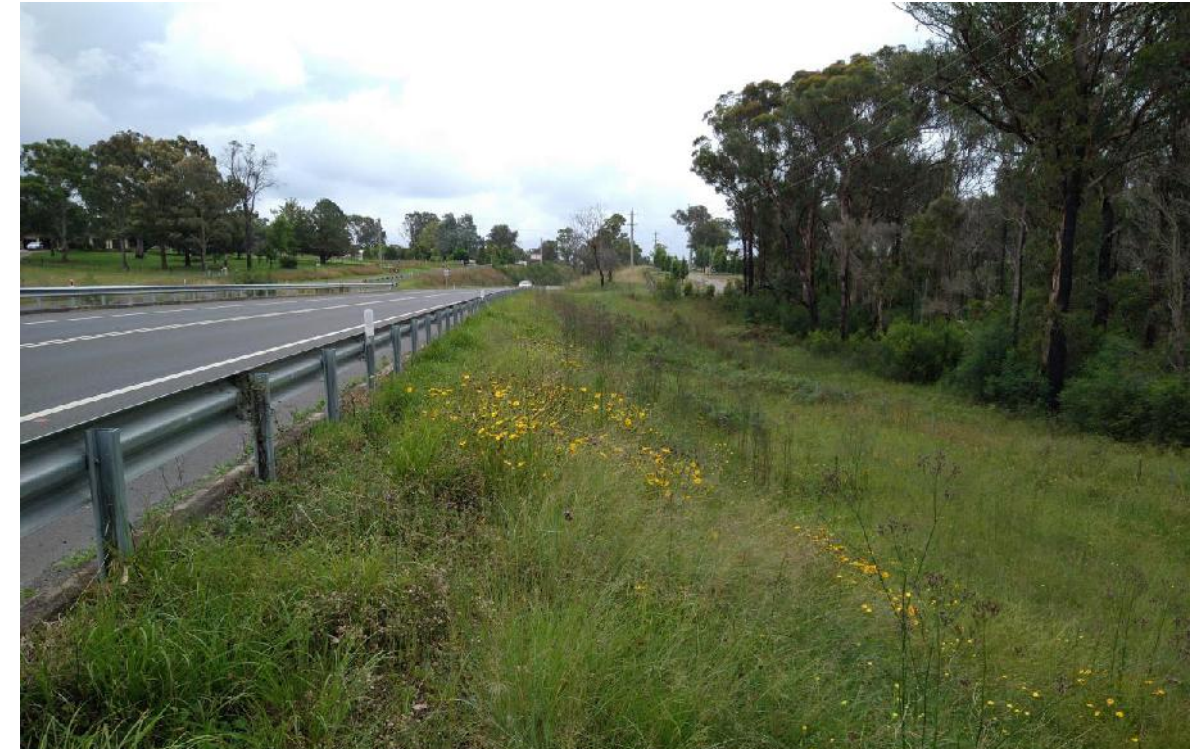
Photo 6: View looking north along the downstream face for RE3.
