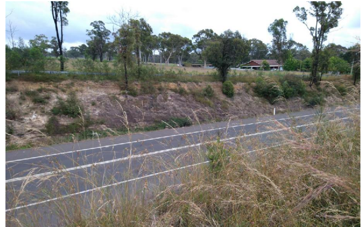
Photo 14: View looking north west towards the road cutting adjacent to No. 3116 Remembrance Drive. Note: the soil and weathered rock in the upper cut and medium to thickly bedded rock in the middle and lower.
