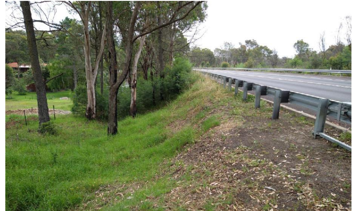
Photo 4: View looking north along the upstream face for RE2.
