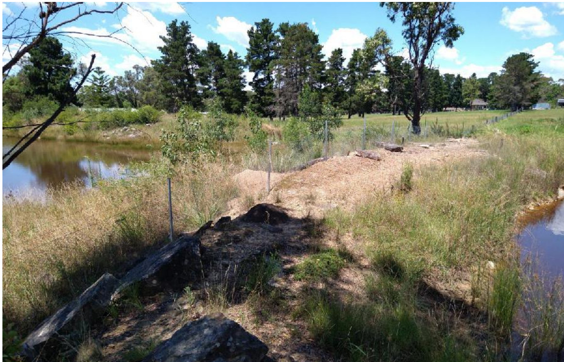
Photo 33: View looking south along the crest for FD9. Note: the sandstone cobbles and boulders placed embedded in the crest.
