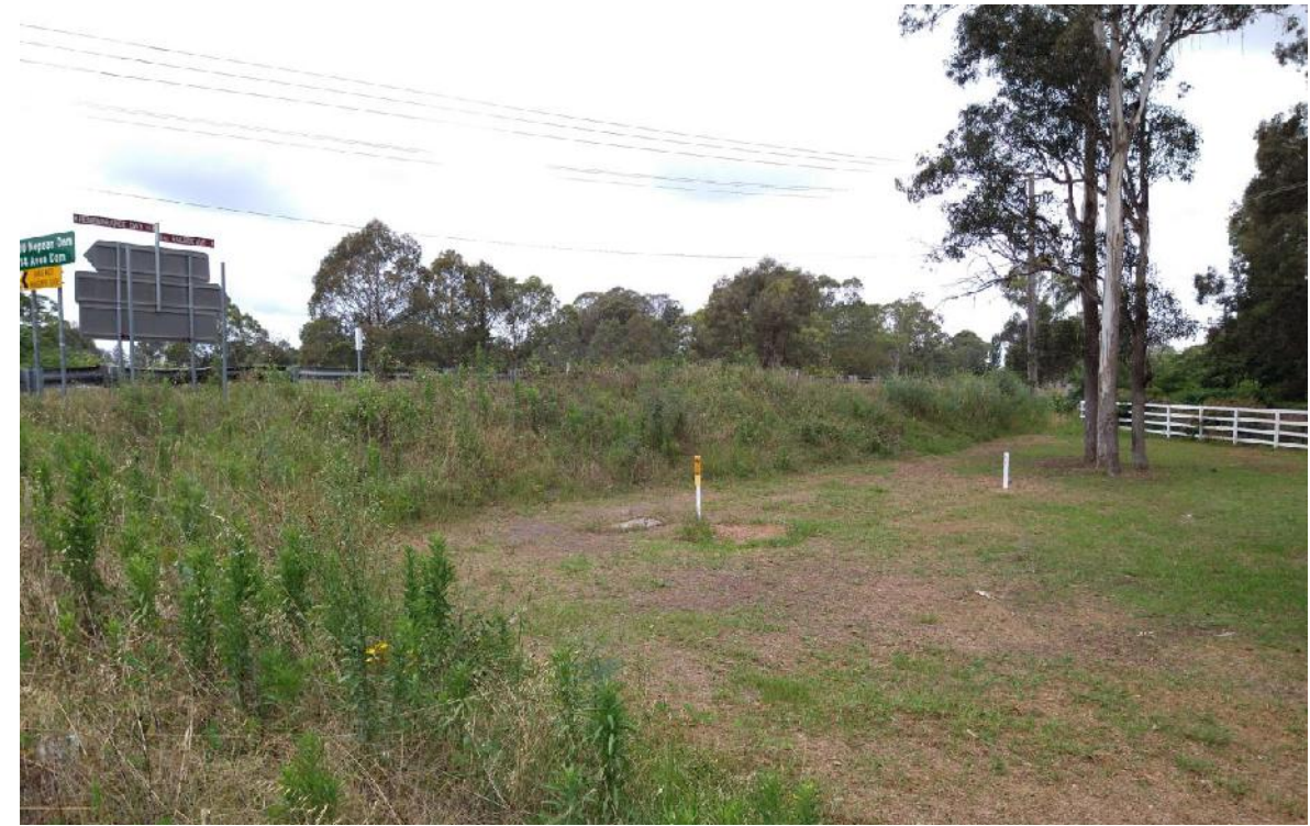
Photo 2: View looking south east across the south western corner of the RE1 road embankment.
