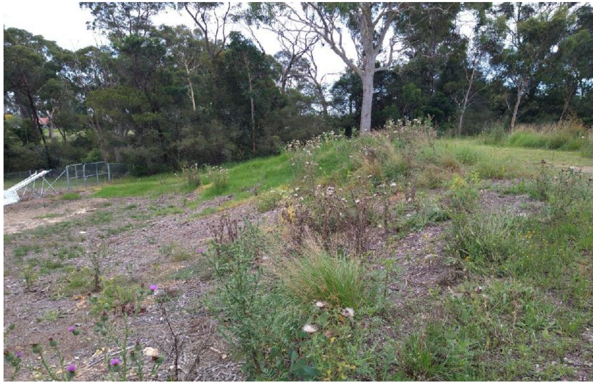
Photo 29: View looking north along the downstream embankment face of FD2.
