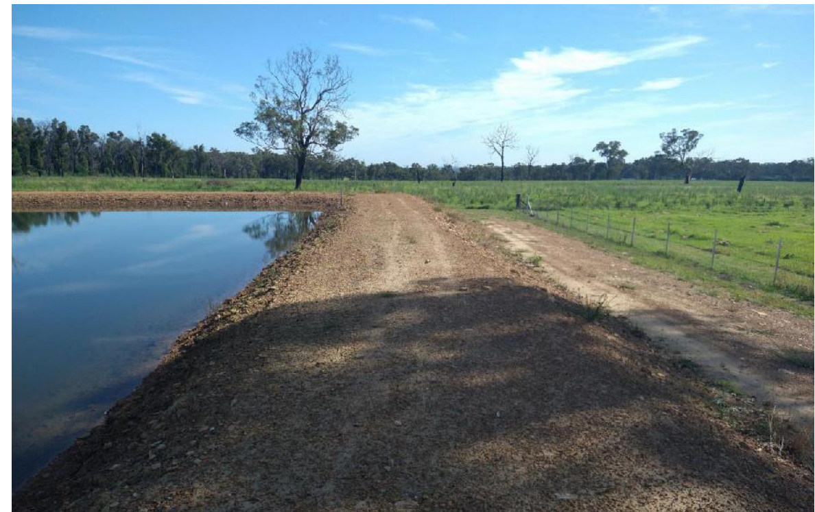
Photo 44: View looking along the eastern wall of FD45.
