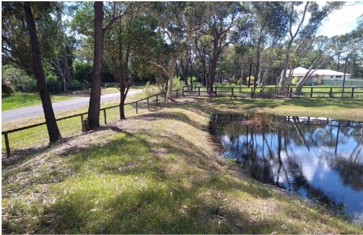
Photo 39: View looking east across the crest of FD39.
