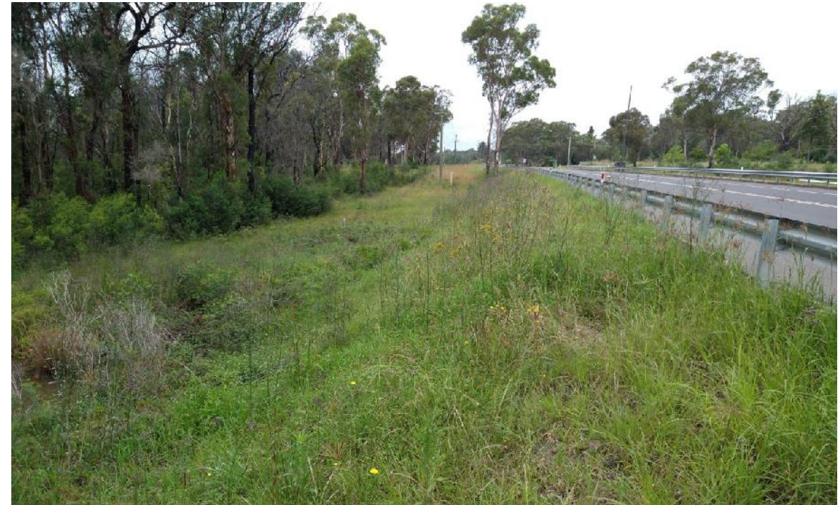
Photo 8: View looking south along the downstream face crest for RE3.
