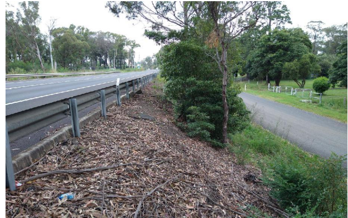
Photo 10: View looking along the crest of the upstream face for RE4.
