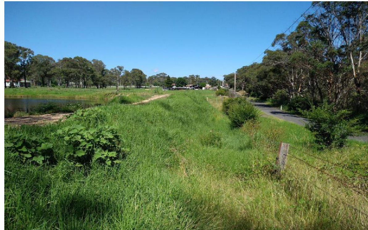
Photo 34: View looking west across the downstream embankment of FD15.
