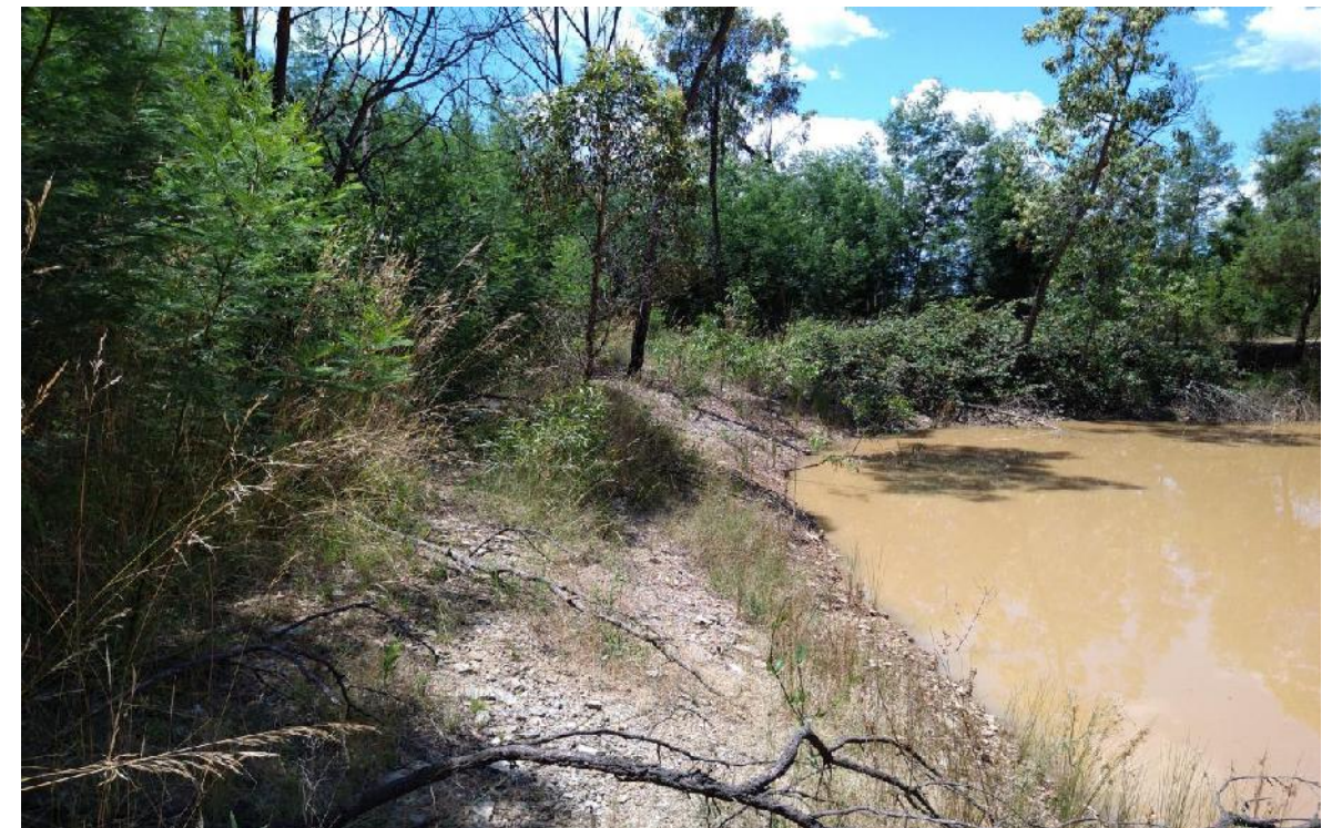
Photo 36: View looking east across the upstream embankment face of FD22.
