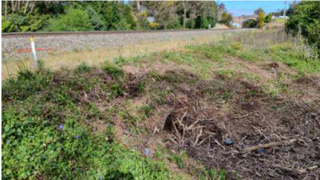
Photograph courtesy Newcastle Geotech
