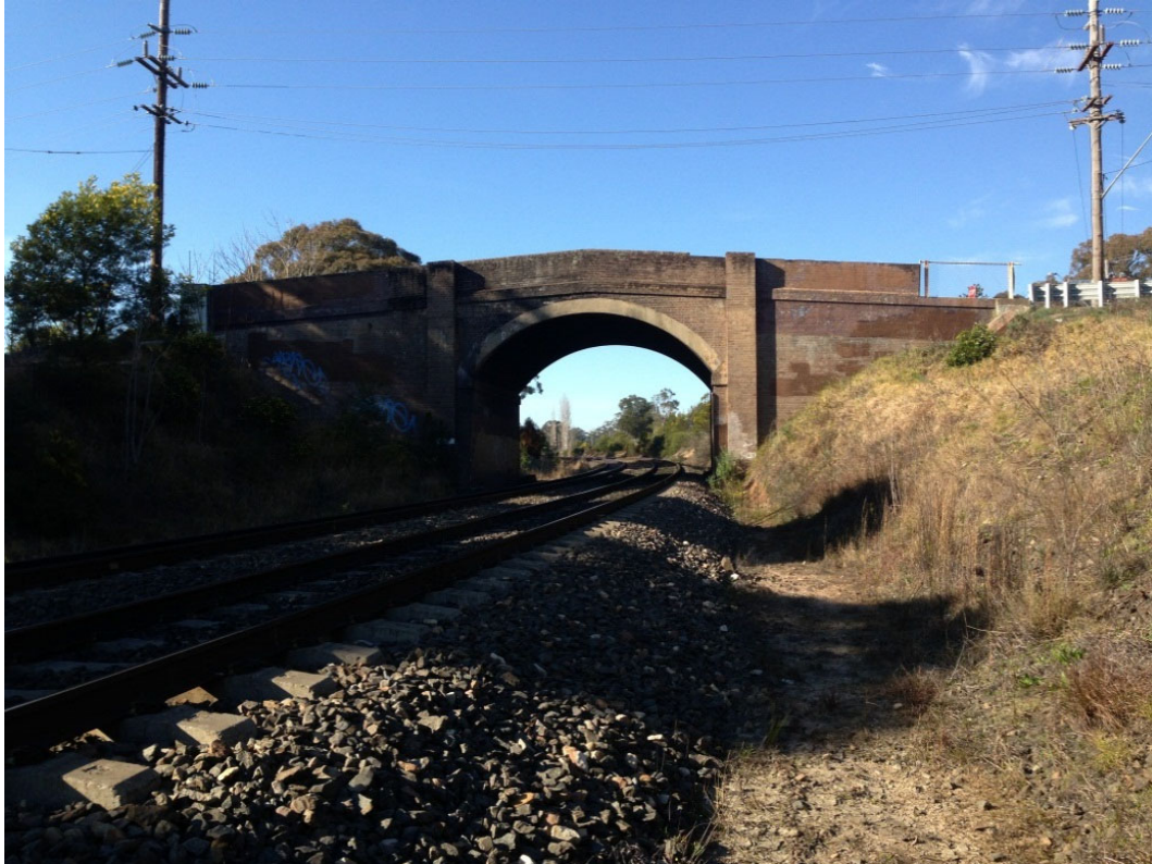
Fig. 3.38 Wellers Road Overbridge
