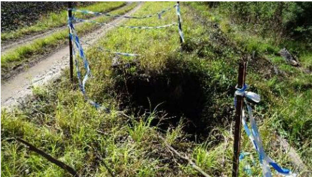
Fig. 3.18 Embankment at 99.035 km on Up side with piping hole above culvert on Down side
