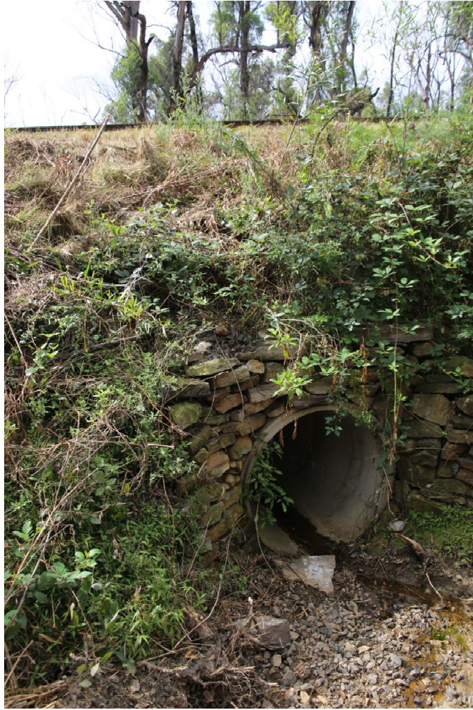
Photograph courtesy Robinson Rail
