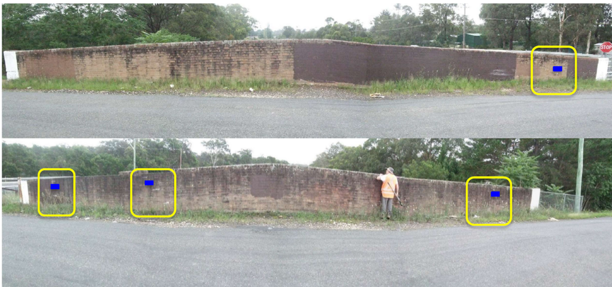
Photograph courtesy JMA Solutions (2022d) with blue lines where crack gauges are recommended
