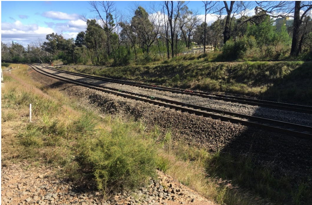
Fig. 1.2 Main Southern Railway at 98.2 km
