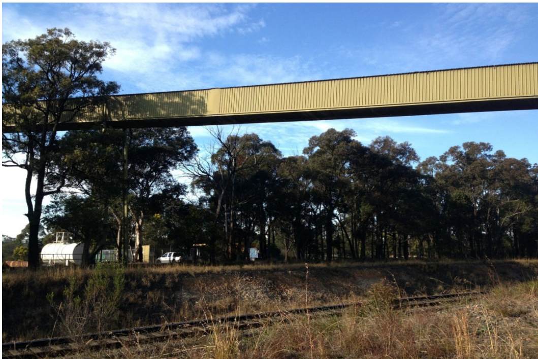
Fig. 3.40 Tahmoor Mine overhead coal conveyor 3R over the Main Southern Railway near 98.160 km
