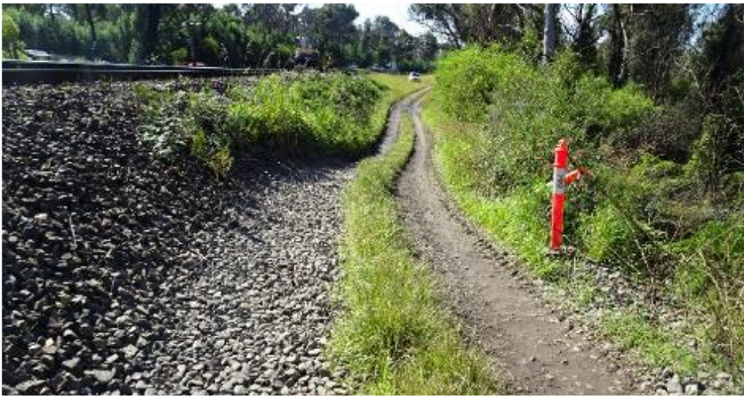
Fig. 3.19 Culvert at 99.338 km on Up side and Down side where concrete extension has washed away, resulting in steep batter slope / scarp
