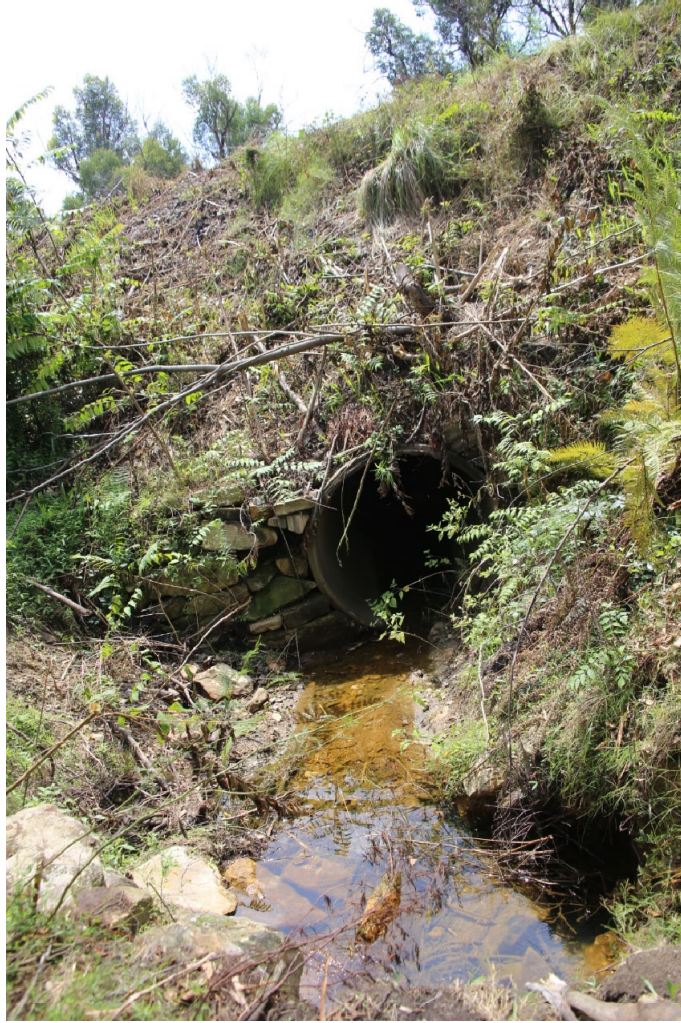
Photograph courtesy Robinson Rail
