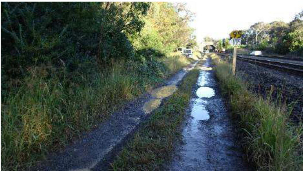
Photograph courtesy Newcastle Geotech
