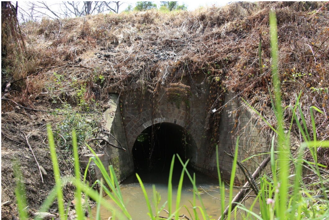
Photograph courtesy Robinson Rail
