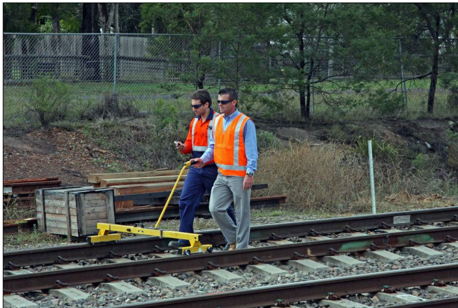
Photograph courtesy Pidgeon Civil Engineering
