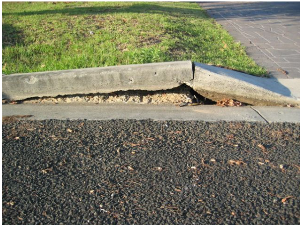
Fig. 3.20 Impacts on local roads above Tahmoor Mine
