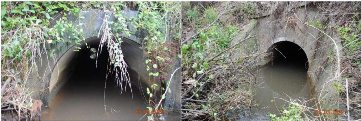
Photographs courtesy Building Inspection Services
