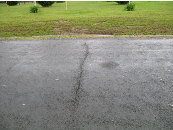
Fig. 3.20 Impacts on local roads above Tahmoor Mine
