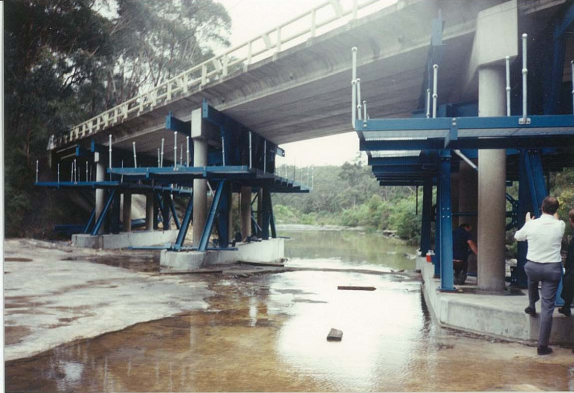
Fig. 3.41 Jacking frames installed at Rockford Road Bridge over Bargo River
