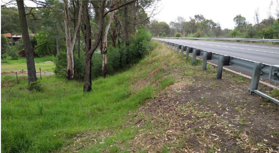
Photograph courtesy Douglas Partners
