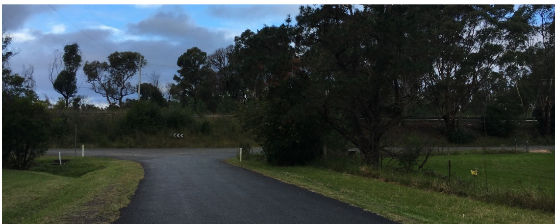
Fig. 3.24 Remembrance Drive embankment from intersection with Caloola Road on upstream side
