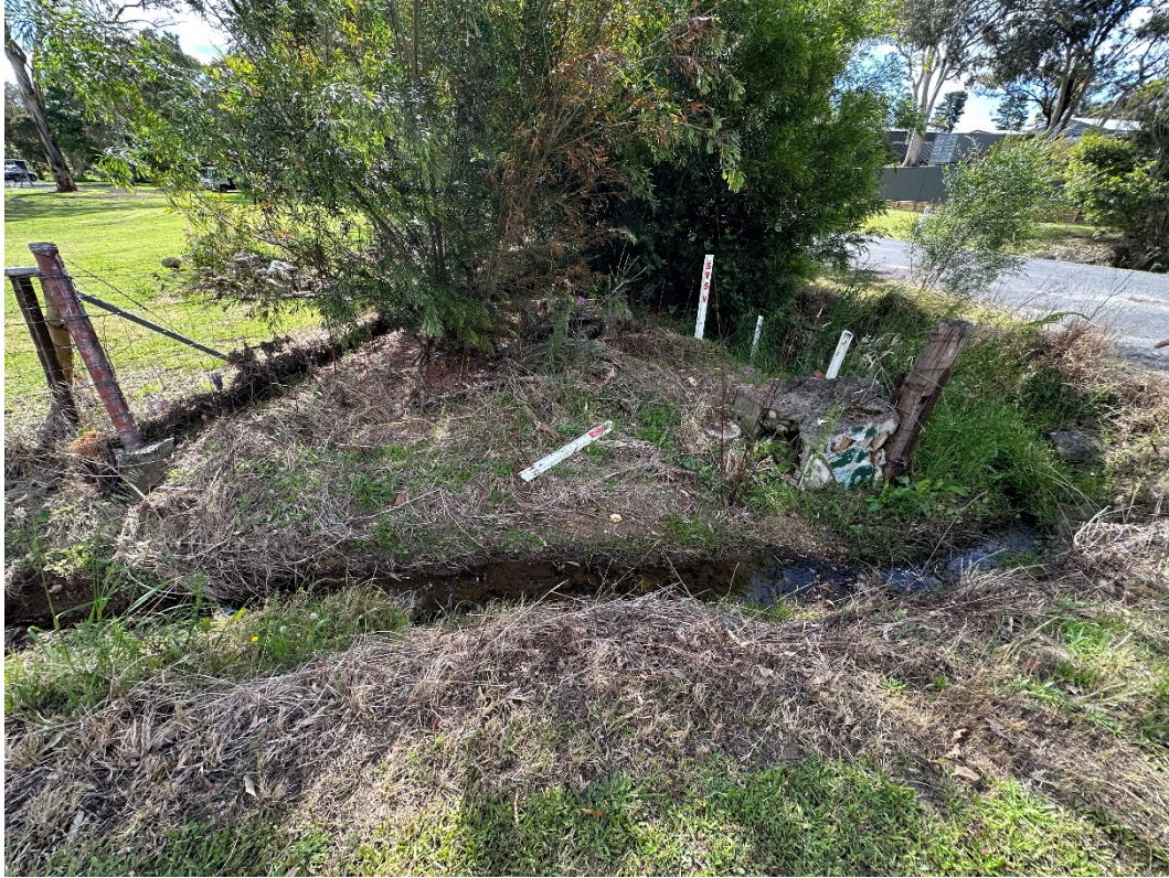
Fig. 3.12 Sydney Water pit for potable water main at intersection of Remembrance Drive and Caloola Road
