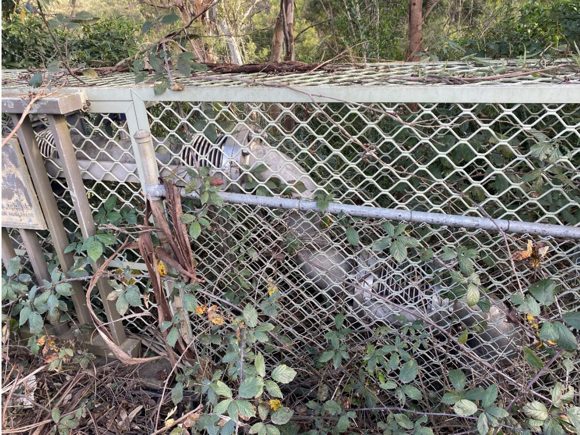
Fig. 3.8 Expansion loop for 150 mm DICL pressure main on Remembrance Drive Bridge over Bargo River
