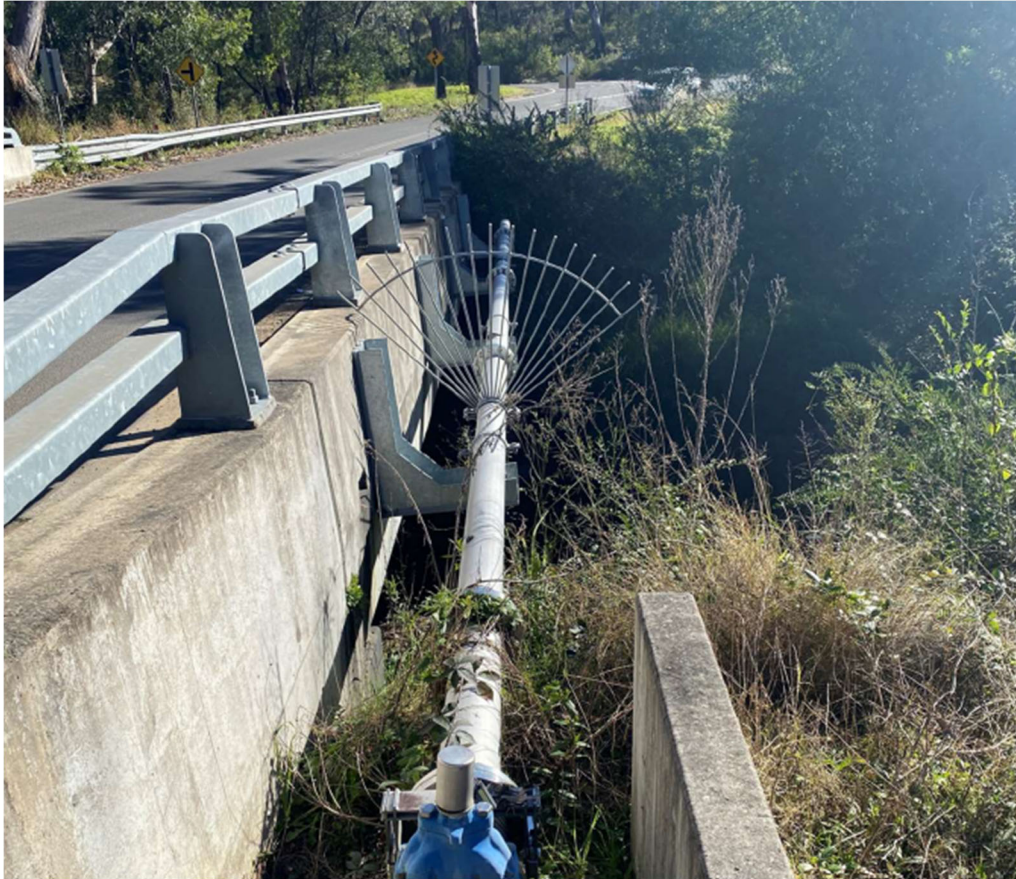
Fig. 3.10 160 mm steel pressure main on Bargo River Road Bridge over tributary to Bargo River
