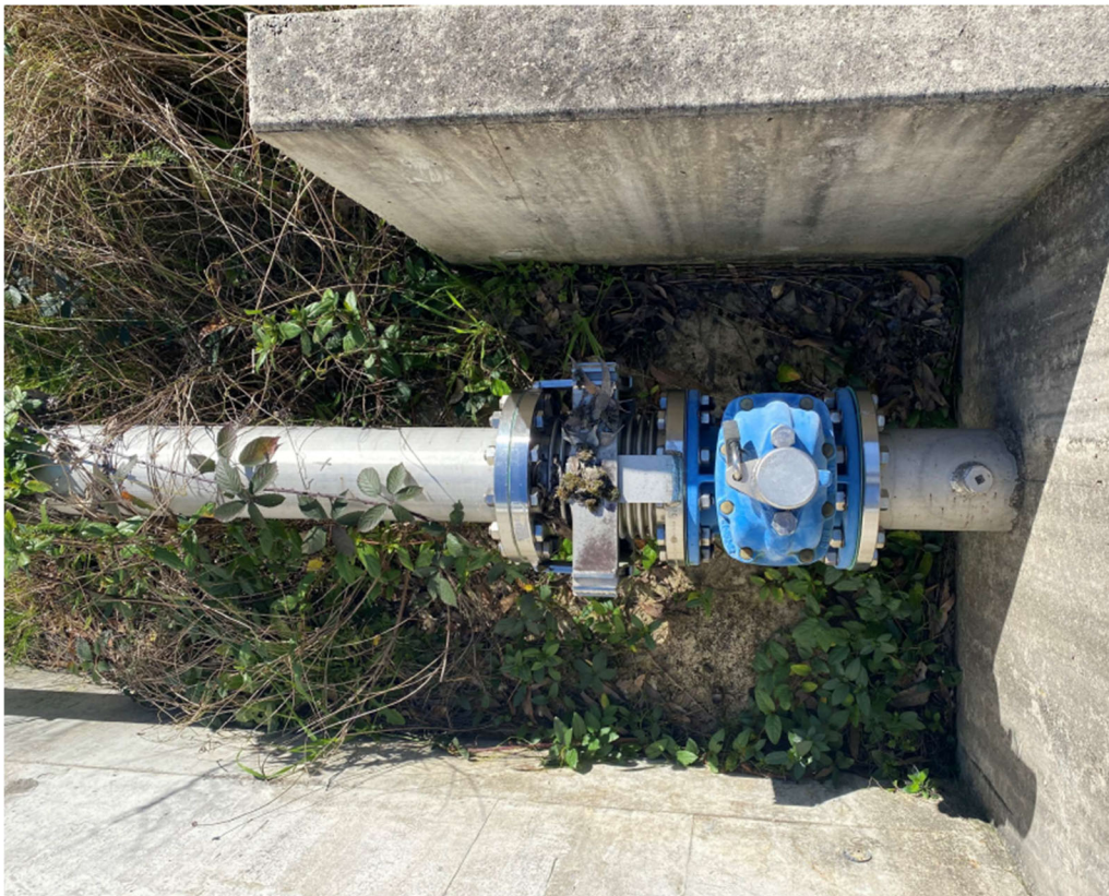
Fig. 3.10 160 mm steel pressure main on Bargo River Road Bridge over tributary to Bargo River
