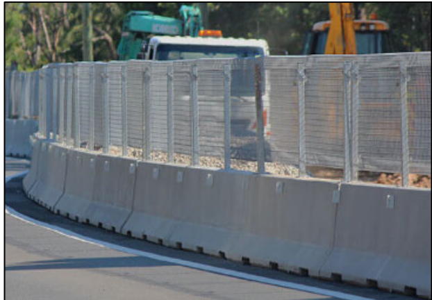
Figure 4 - Barrier with gawk screen high hoarding
