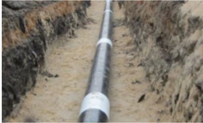
Figure 3 – Pipe exposed or ‘uncoupled’ to eliminate potential ground strain
