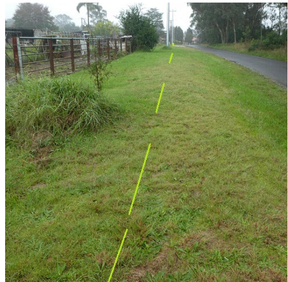
Plate 8 View west along Charlies Point Rd towards Great Southern Rd showing NBN direct buried 20/0.64 HJ cable
