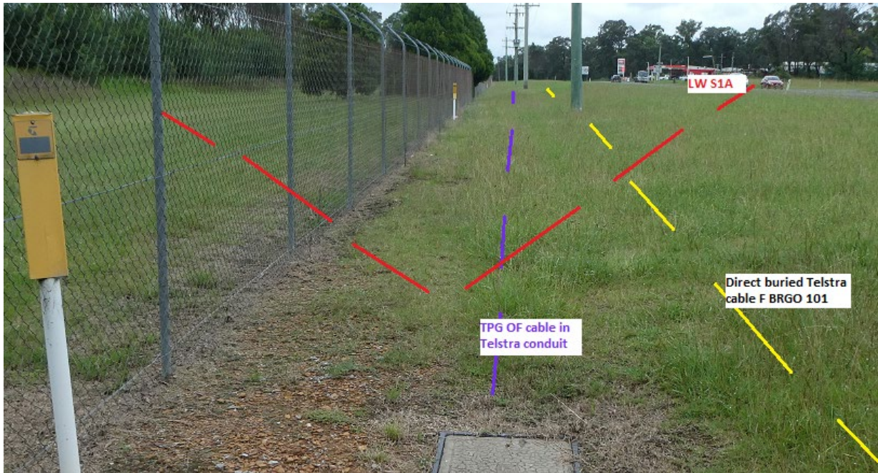
Plate 5:- View south to north end of LW S1A showing TPG OF cable in Telstra conduit and direct buried Telstra IEN cable installed parallel and around 3m-5mm to the west.
