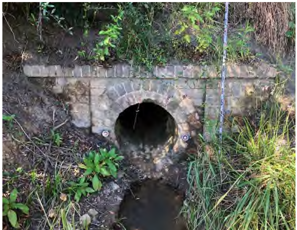
Photo 87.630-1 Western portal. In sound condition
