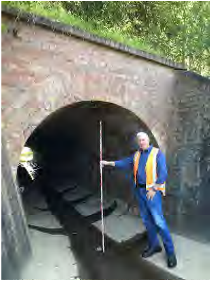
Eastern portal. Culvert is in good condition.
