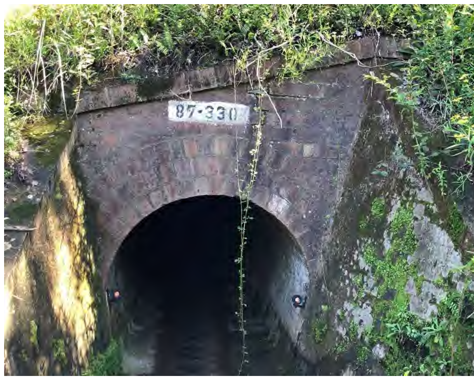
Eastern (downside) portal. In sound condition
