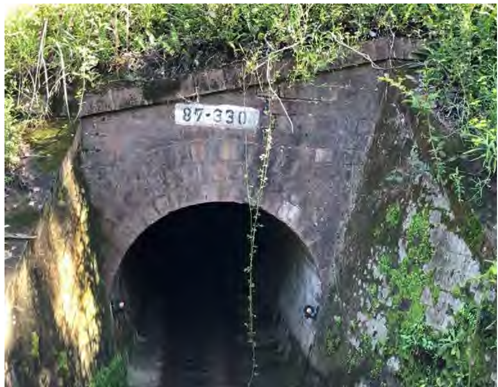
Photo 87.330-1 Eastern (downside) portal. In sound condition
