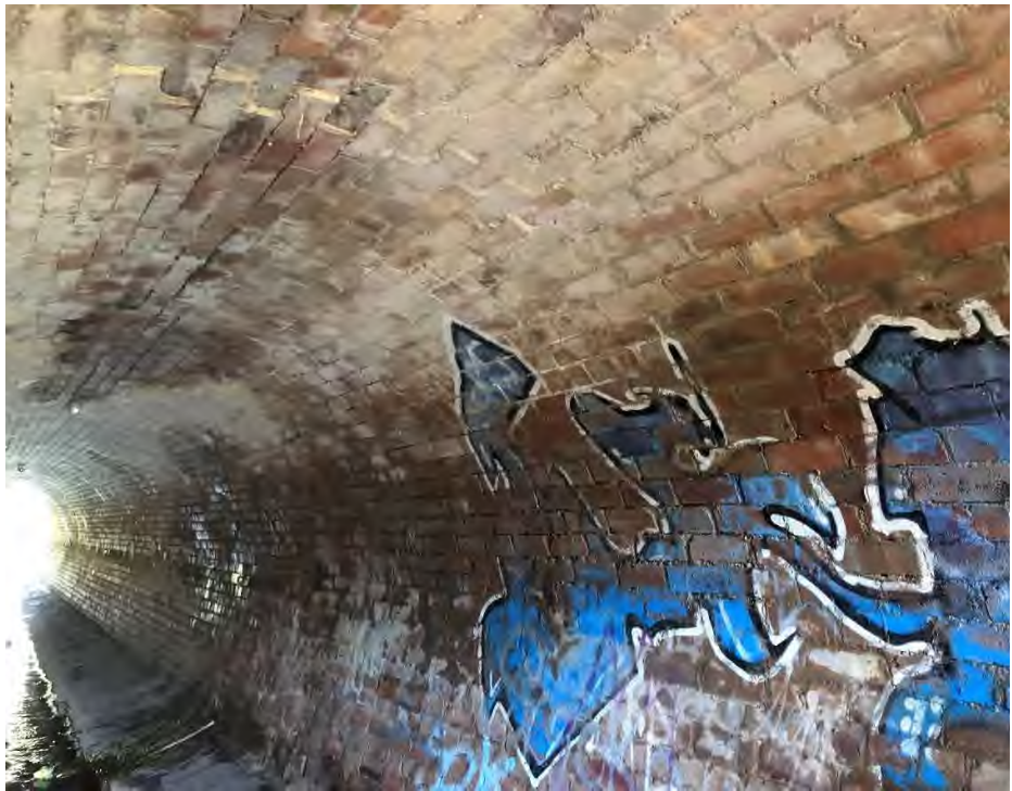
Roof of culvert. View west
