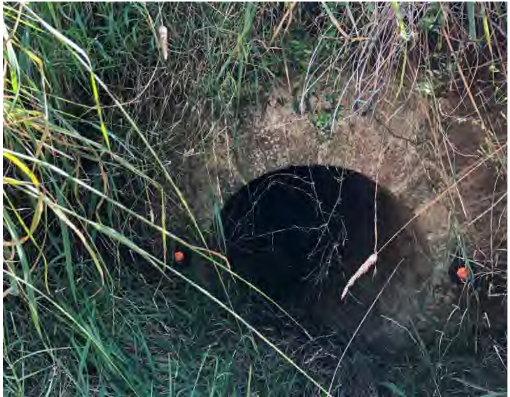
Photo 87.630-2 Eastern portal. Overgrown but appears to be in sound condition.
