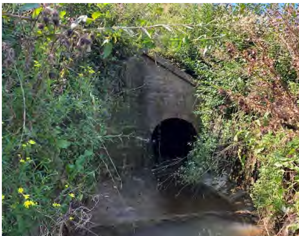
Photo 87.331-1 Western portal. In sound condition.
