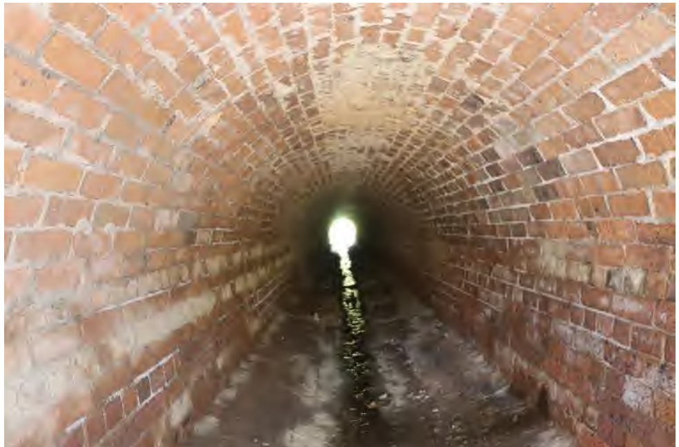
Photo 87.850-3 Masonary culvert barrel.
