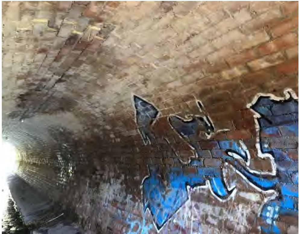
Photo 89.216-2 Roof of culvert. View west
