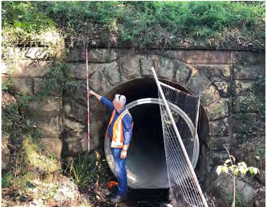
Eastern portal, generally in good condition.
