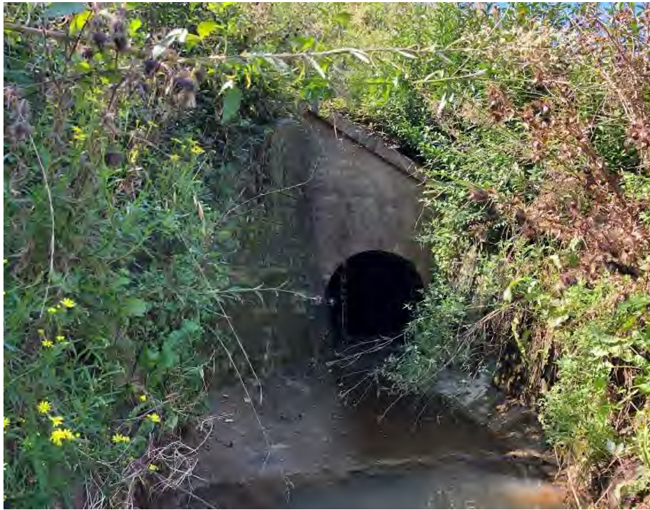
Western portal. In sound condition.
