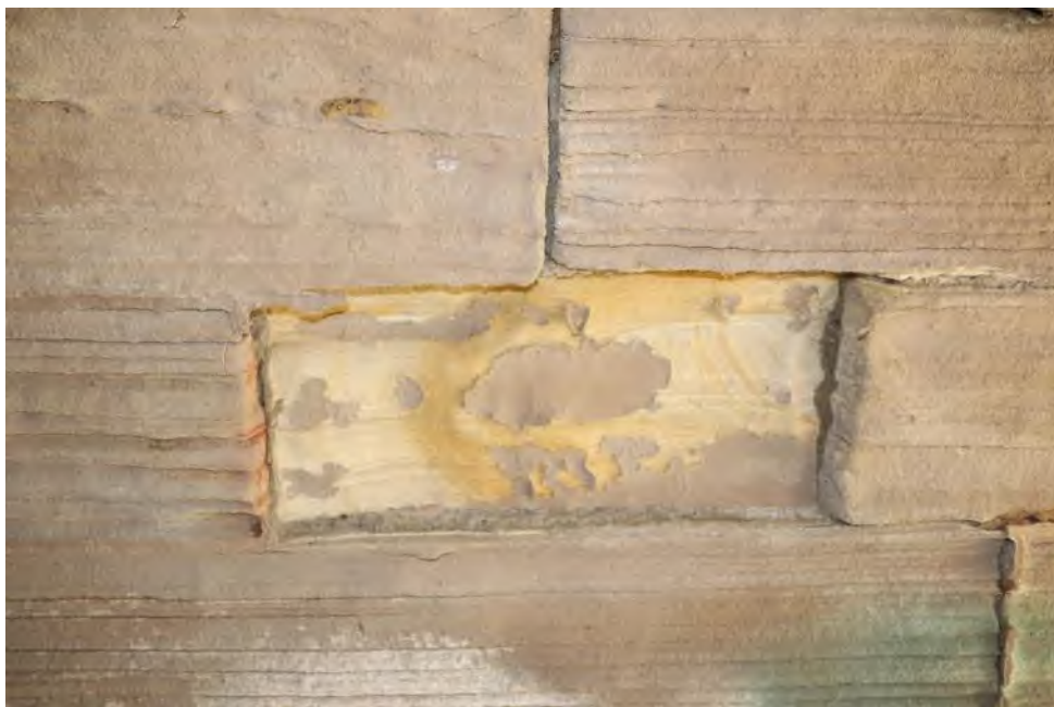
Photo 88.980-4 Example of significantly eroded sandstone block to barrel noted in the pre-mining report.
