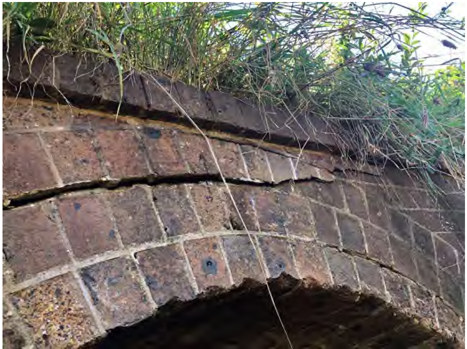
Detail, pre-existing cracking and displacement of bricks around the eastern portal arch that does not appear to have worsened significantly during longwall mining in the Western Domain.
