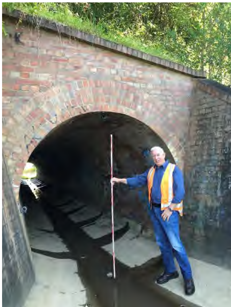
Photo 89.216-1 Eastern portal. Culvert is in good condition.
