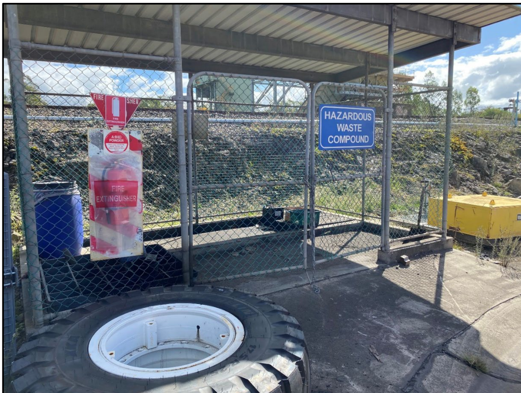
Plate 4. Hazardous Waste Compound (Sealed, bunded roofed)
