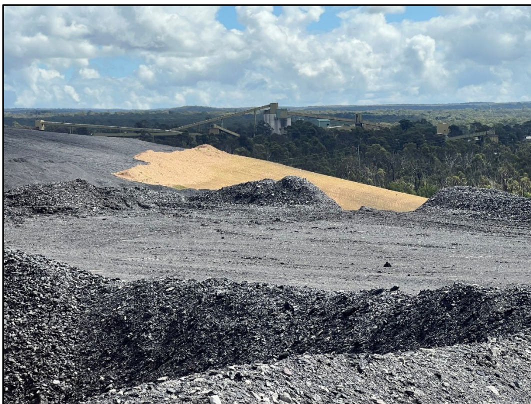
Plate 9. Rehabilitation at REA
