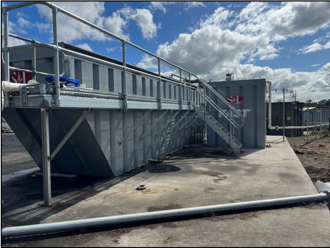
Plate 7. Sewage Treatment Plant
