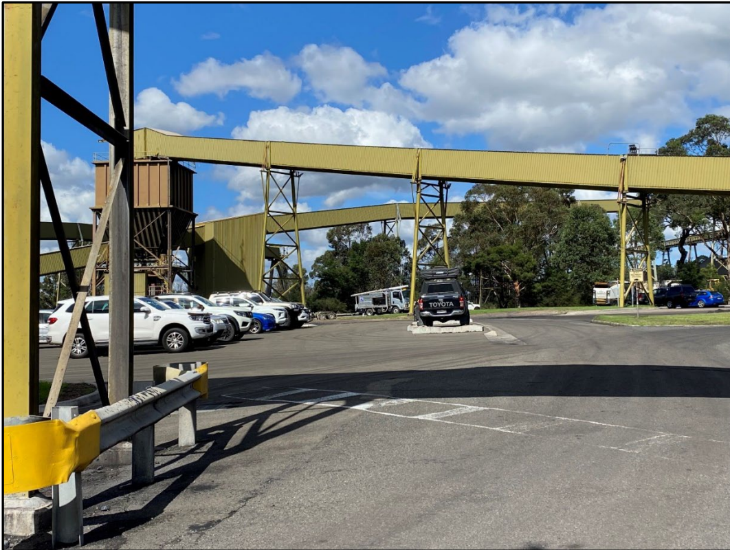
Plate 8. Enclosed Conveyor Belts
